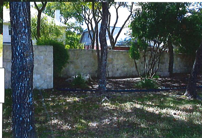
Perimeter Walls and Landscape
