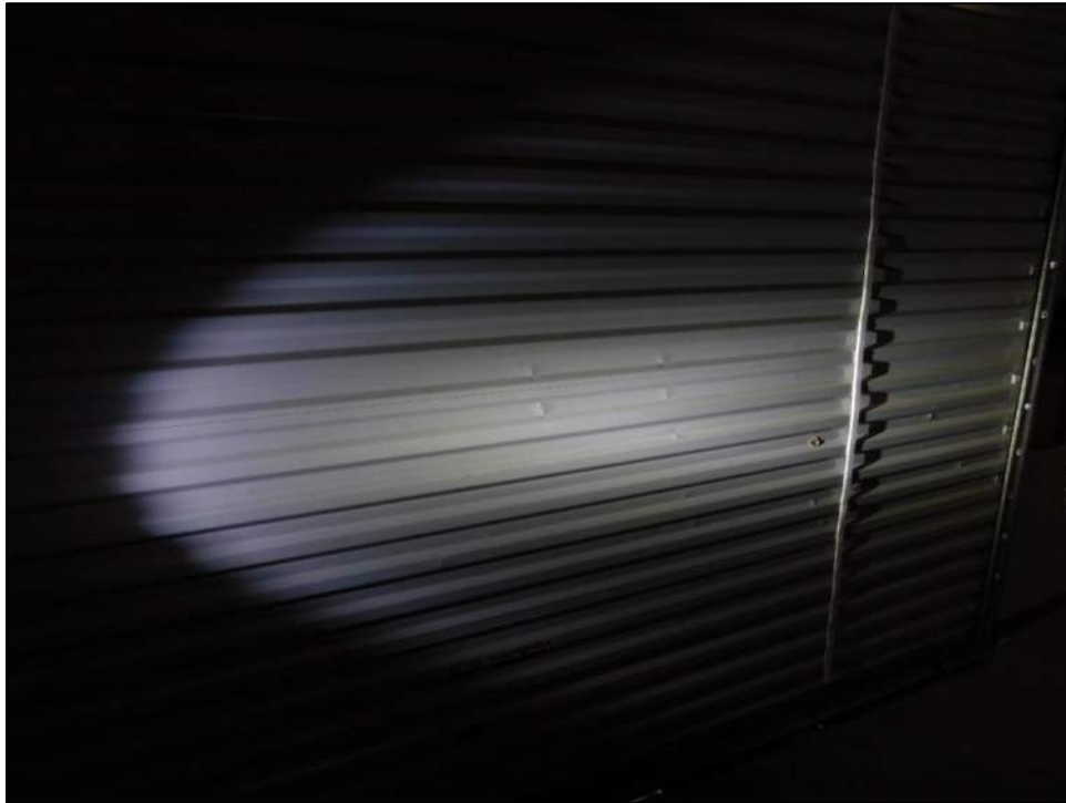
Photo 15: Creasing pattern and arrangement on the lower section of the roll-up was consistent with mechanical impact.
