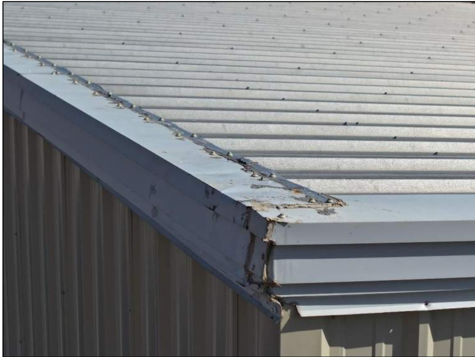
Photo 3: Sealant joints adjoining closure metals remained undisturbed.
