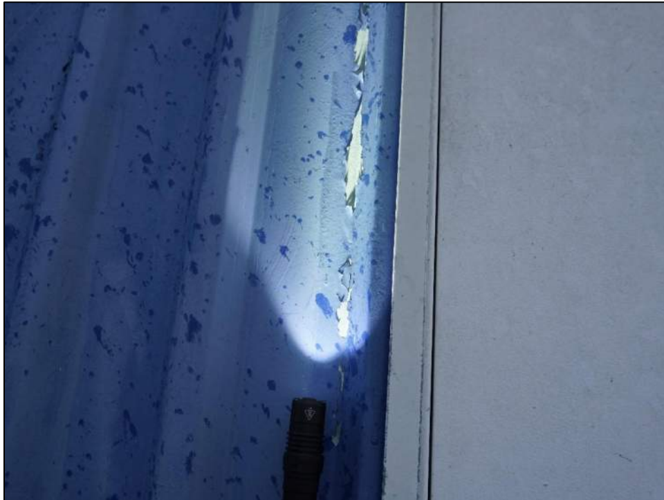
Photo 35: No hail denting was observed on the west wall. Existing coating exhibited aged-related peel.
