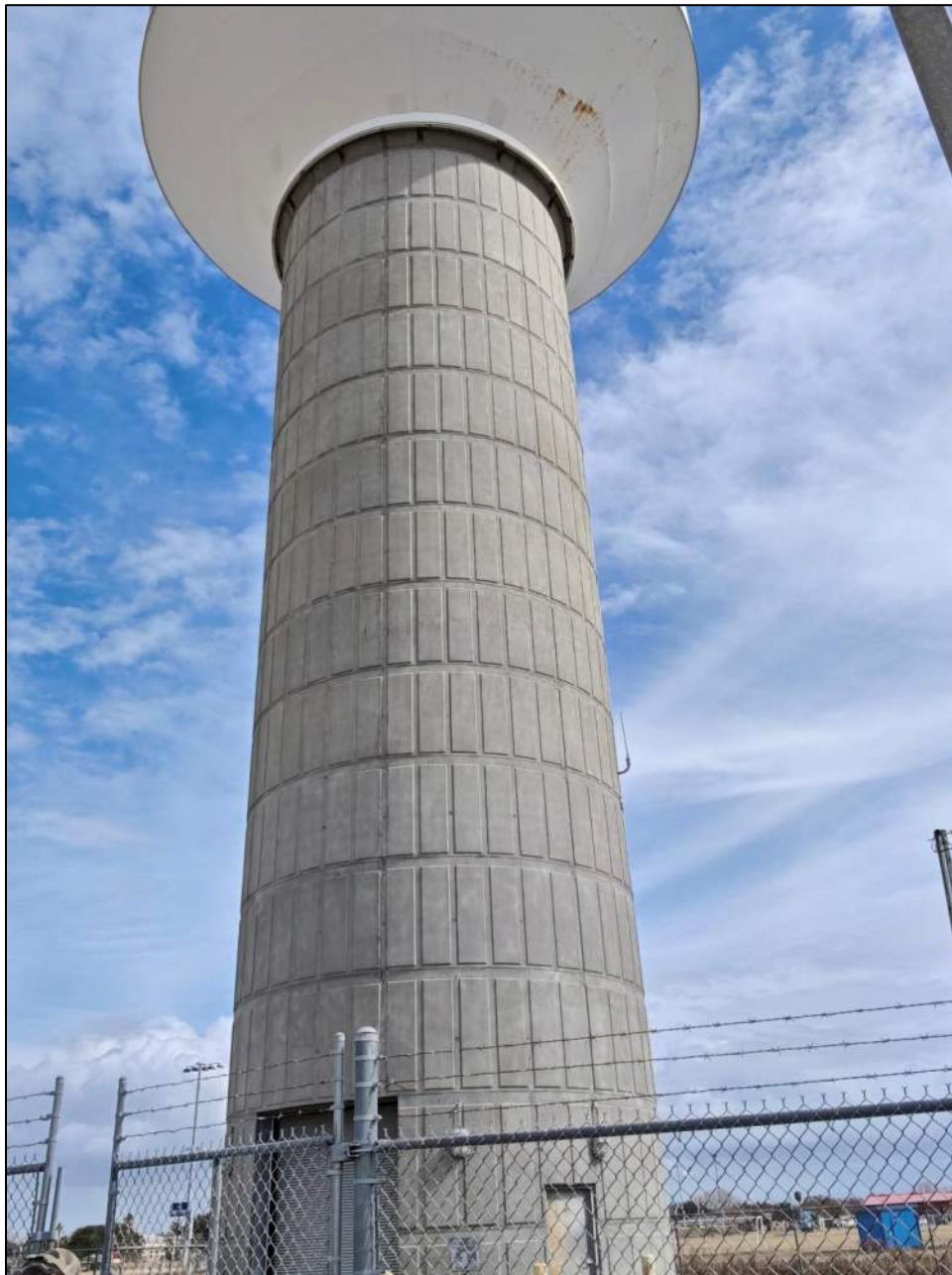
Photo 15: Overview of concrete pedestal of the water tower.
