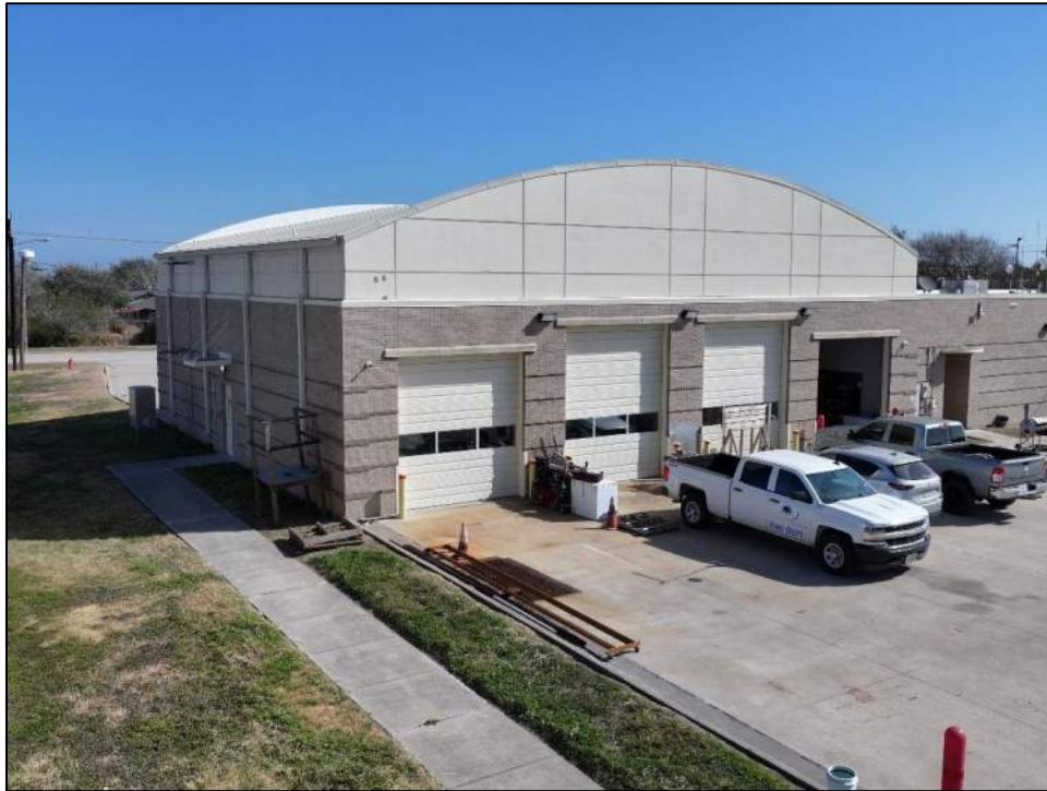
Photo 29: South (rear) elevation of the police department building.
