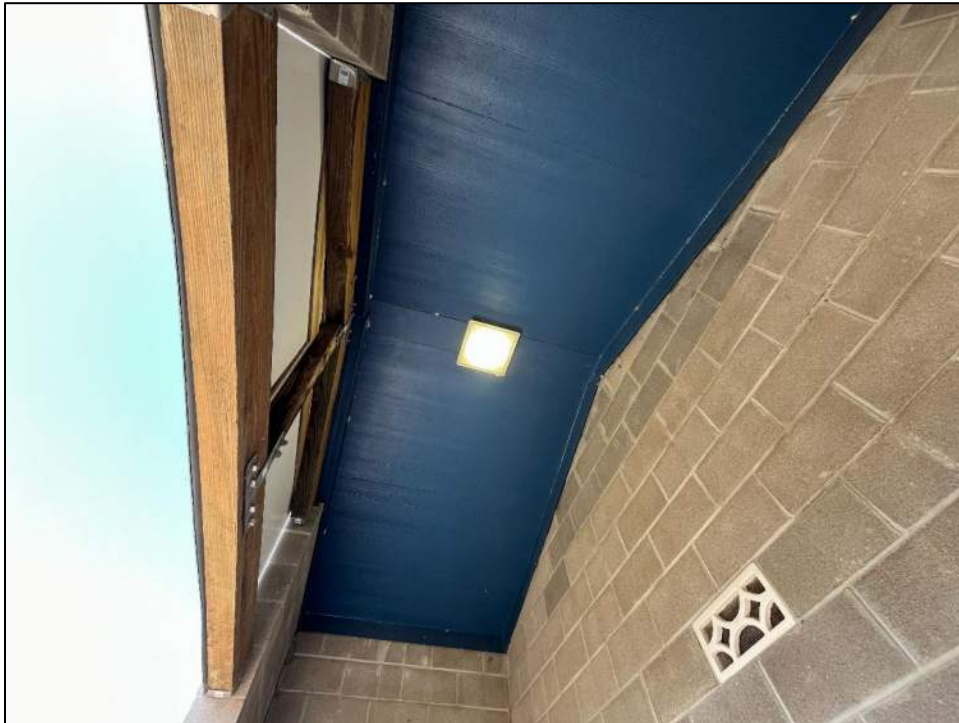
Photo 23: No ceiling stains indicative of roof leaks were observed.
