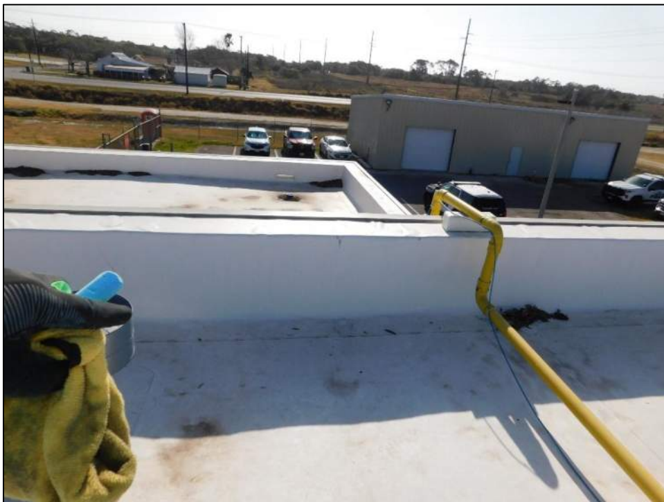
Photo 60: East parapets were closely examined along the base for potential hail impact.
