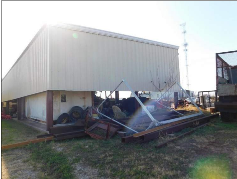
Photo 86: West elevation of the vehicle storage building.
