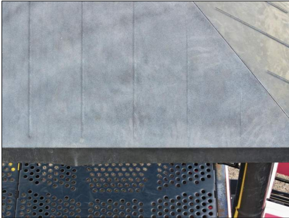
Photo 107: The roof is made of steel plates. No hail impact indentations were observed.
