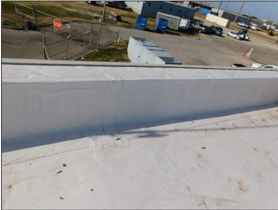
Photo 49: Parapet bases facing the direction of the hail impact were closely inspected for hail impact.
