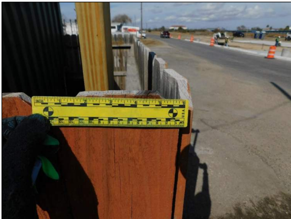
Photo 18: Top of fence pickets were not splintered.
