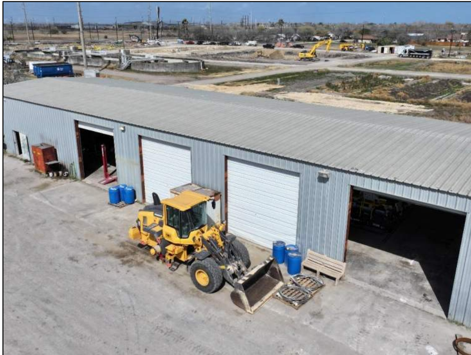
Photo 50: Overview of the vehicle repair building.
