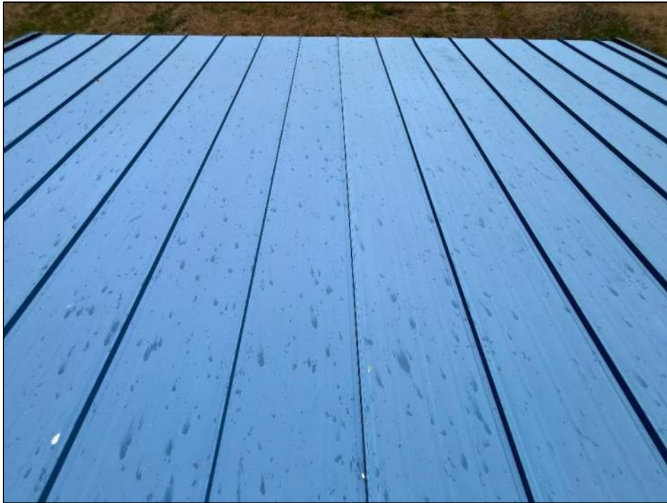
Photo 21: Significantly less dense spatters found on south slope.
