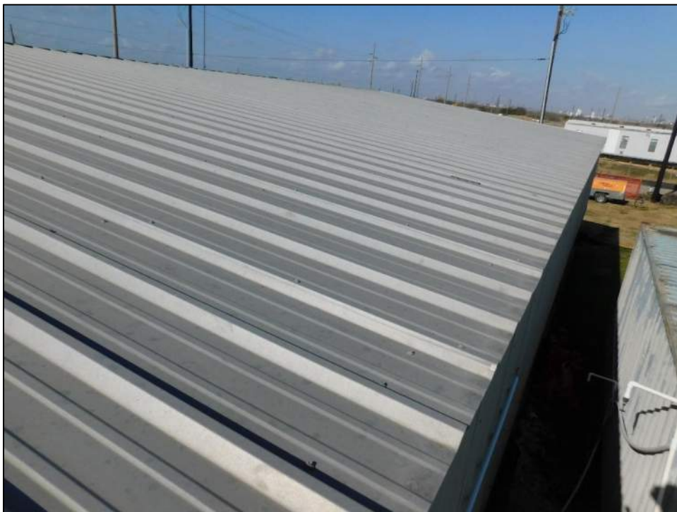
Photo 100: Roof overview. North roof eave remained linear and coplanar.
