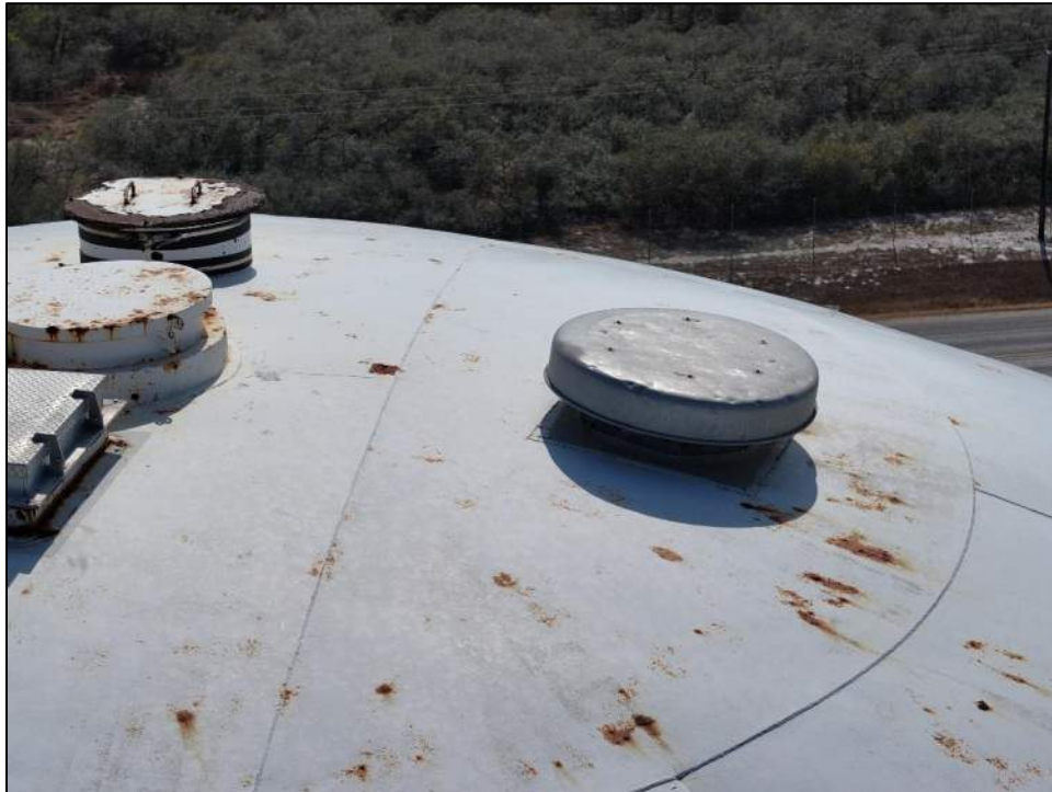
Photo 21: Aluminum vent cover exhibited hail denting.
