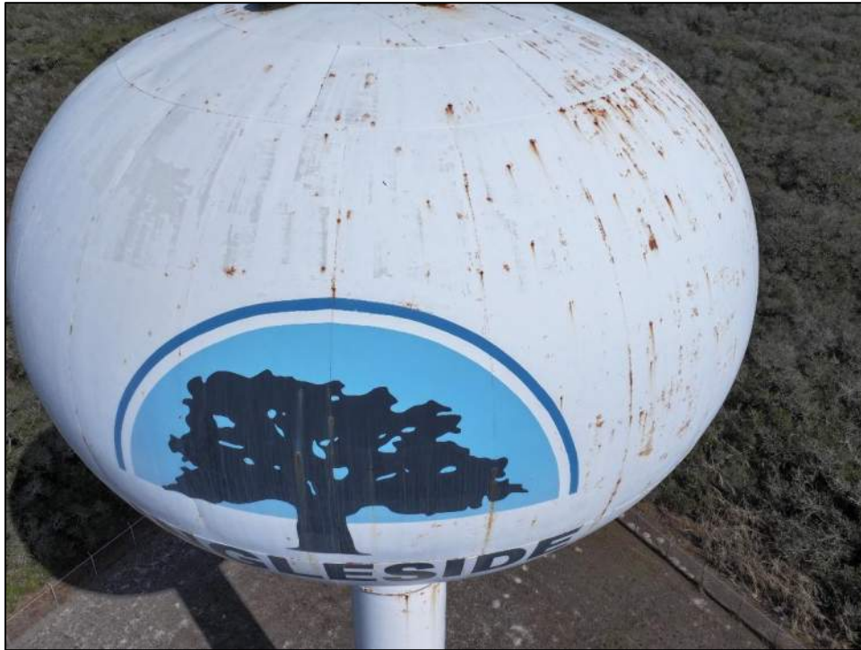
Photo 13: Southwest elevation. South elevation exhibited widespread rusting and steel corrosion.
