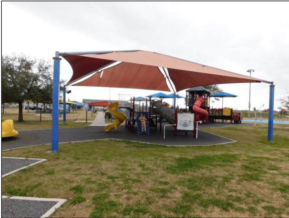
Photo 113: Side view of the playground soft-top canopy.
