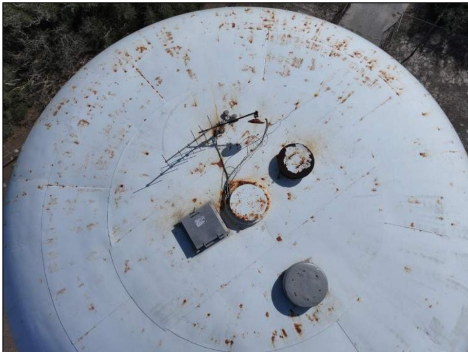
Photo 2: Top-down view of tank roof.
