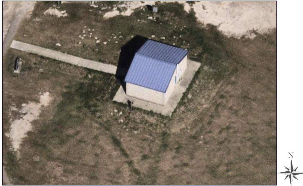
Figure 13 – Structure 018-001, the Cove Park Restroom. Date of Imagery: November 9, 2024. Source: Nearmap®.
