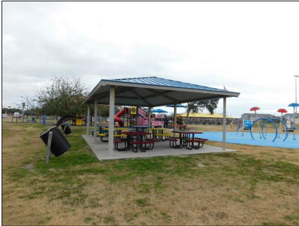
Photo 1: East elevation of the splashpad pavilion.
