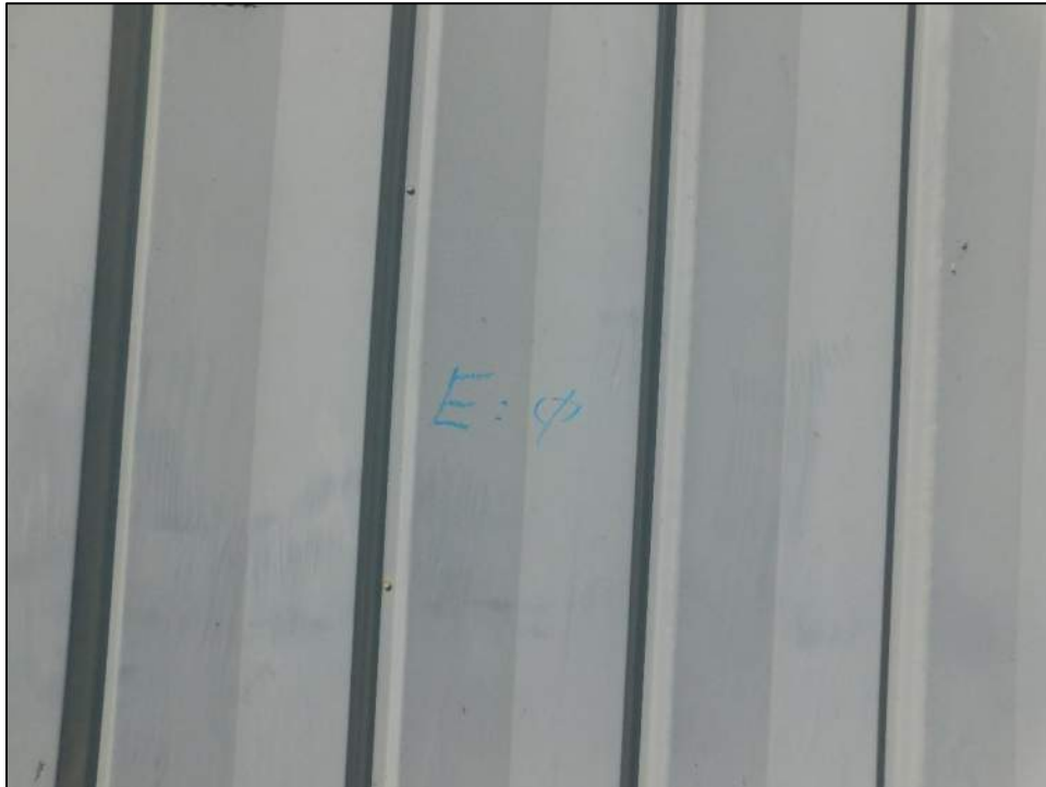
Photo 9: East elevation wall panels exhibited no hail spatters.
