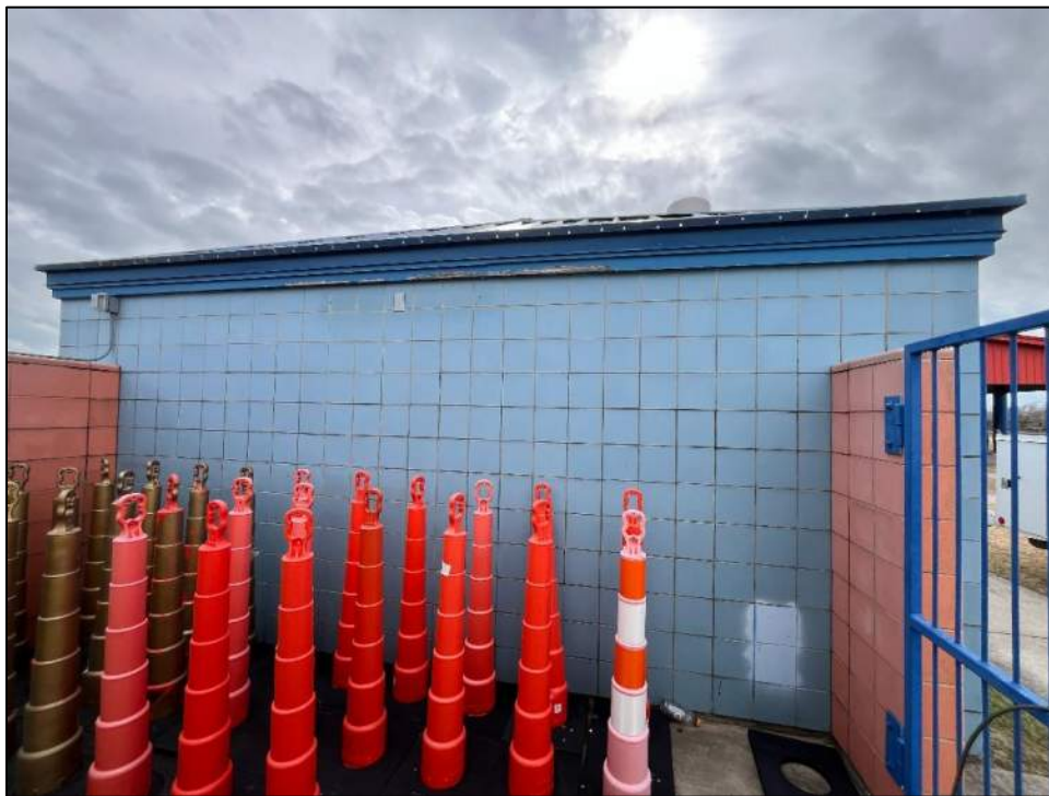
Photo 124: North (rear) elevation. No fractured tiles were observed.
