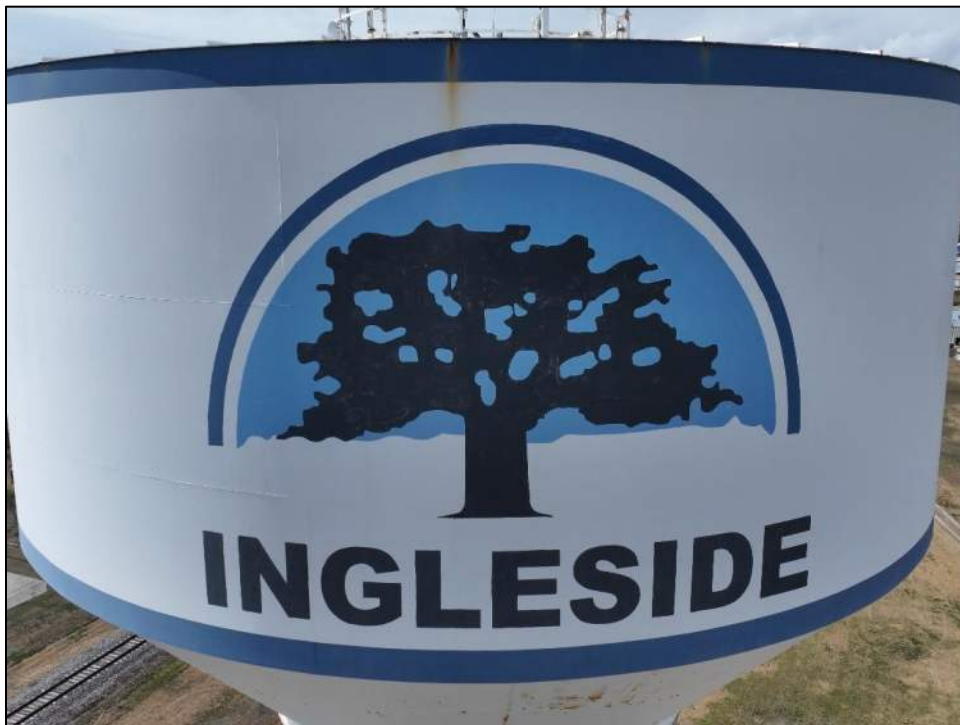
Photo 8: East-facing elevation remained intact.
