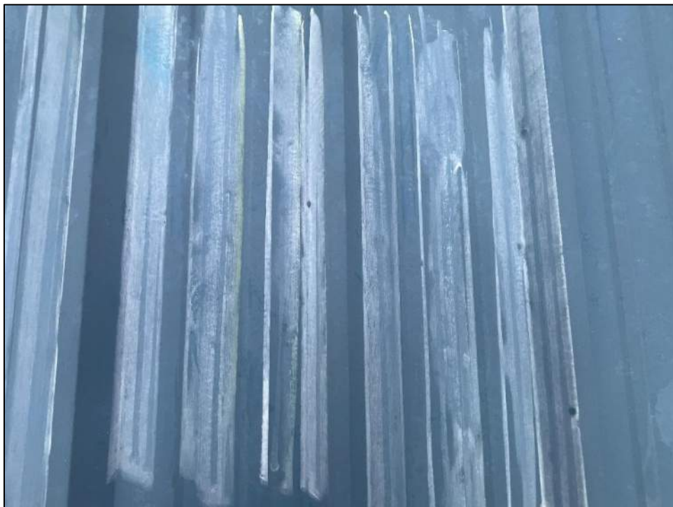
Photo 25: No discernible hail denting to south slope due to steep slope.
