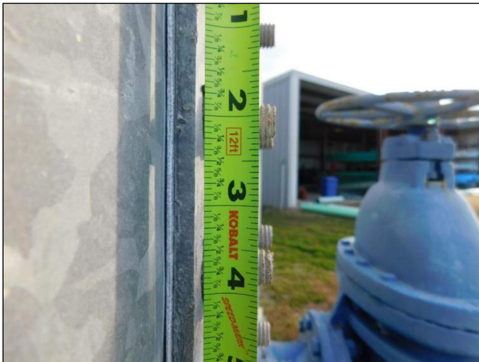
Photo 66: Steel wall plates were approximately 1/4-inch thick
