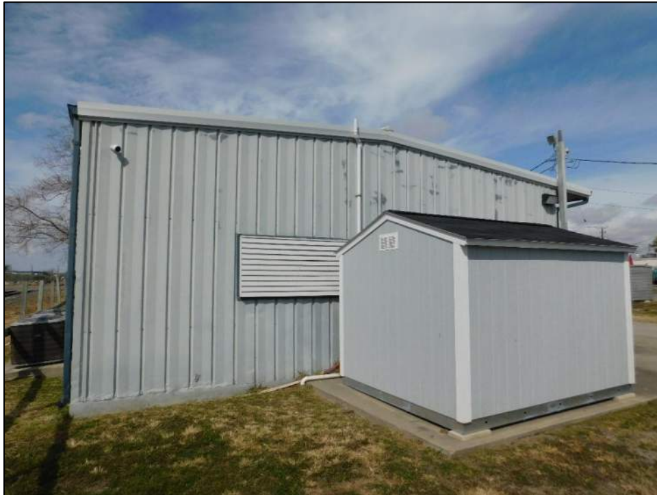
Photo 7: East elevation wall panels exhibited no hail spatters.
