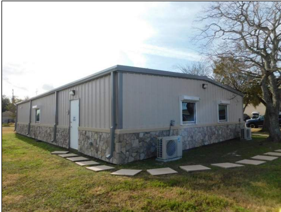
Photo 3: West elevation. Windows remained intact
