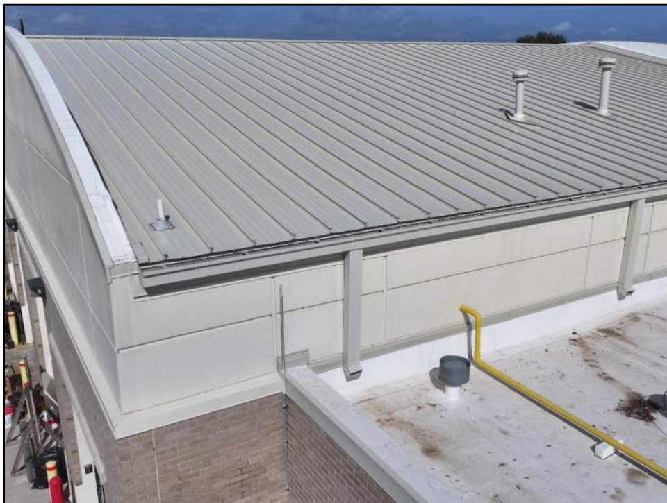
Photo 34: Downspouts on east kneewalls of the fire department remained intact
