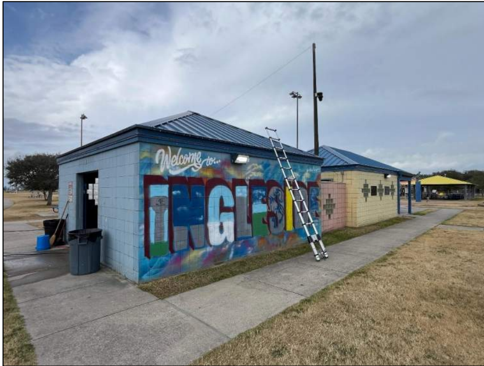
Photo 121: South and east elevations.
