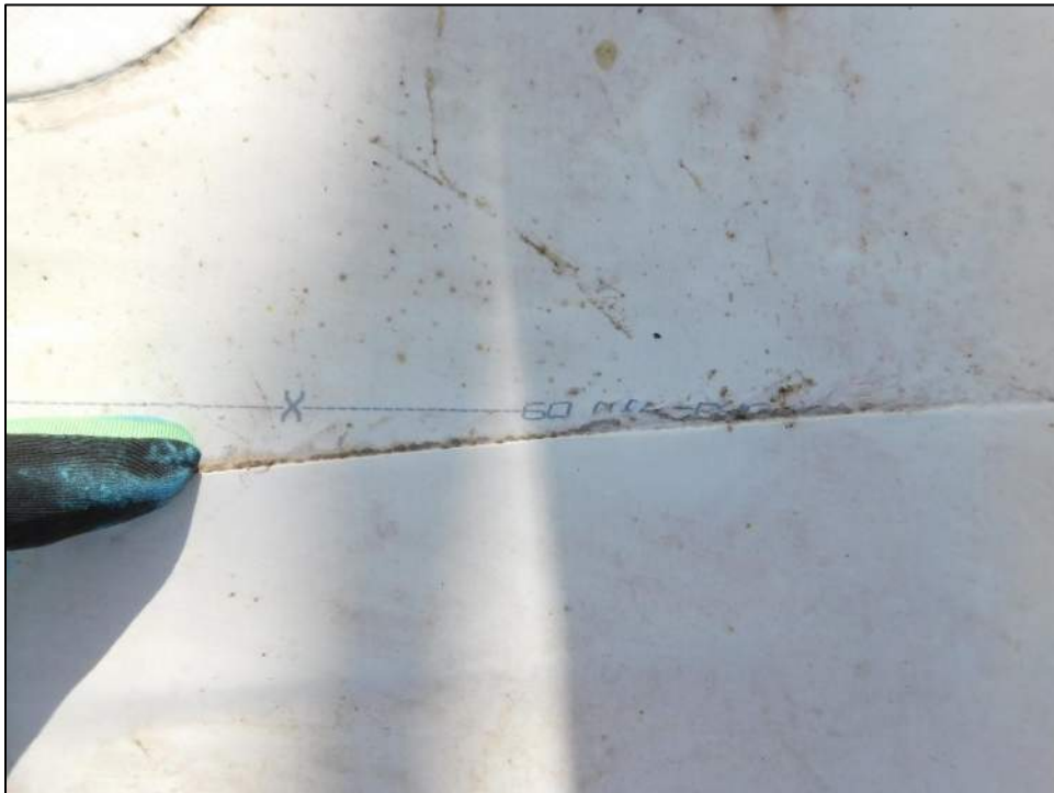
Photo 54: close-up of the 60-mill PVC marking.
