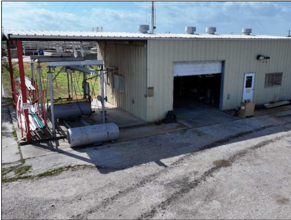
Photo 1: Front (north) elevation of the electrical (waste water pump room) building.
