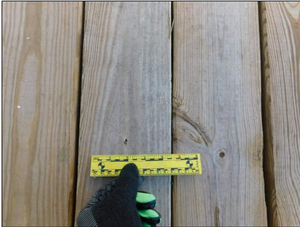
Photo 88: No crushed wood grains were observed on the wooden ramp.
