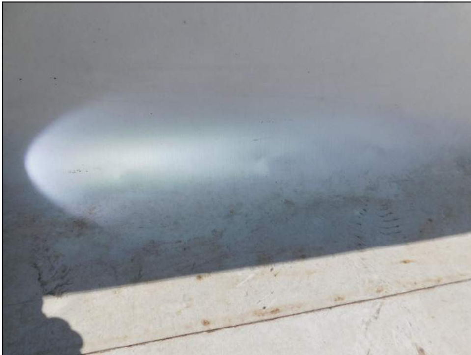
Photo 26: Unsupported PVC membranes at the base of parapets facing the direction of the hail were not punctured dimpled or scuffed.
