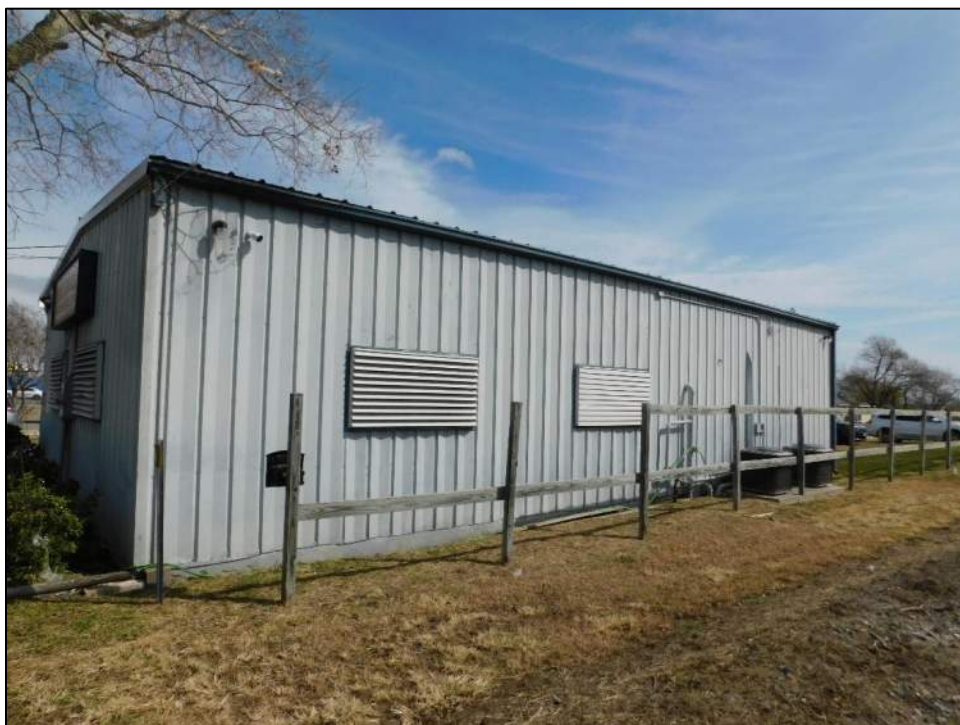
Photo 6: South elevation of building was unaffected by hail.
