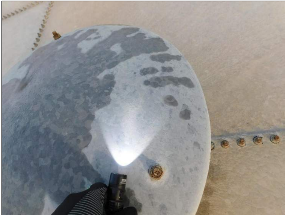
Photo 72: Tank roof vent was not dented.
