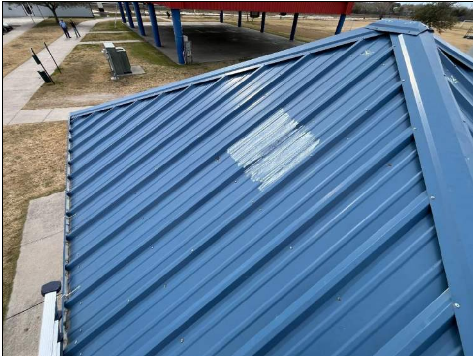
Photo 125: East slope. Eave closure remained intact.
