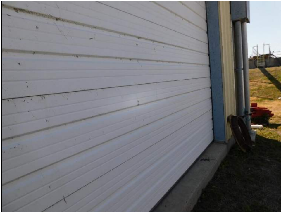
Photo 10: No hail denting was observed on the west wall roll-up door panels.
