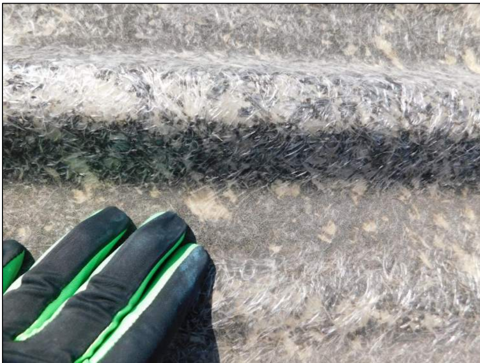
Photo 92: Skylight panels were not fractured at the spatters.
