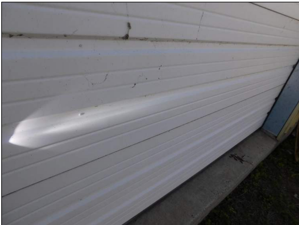
Photo 11: No hail denting was observed on the west wall roll-up door panels.
