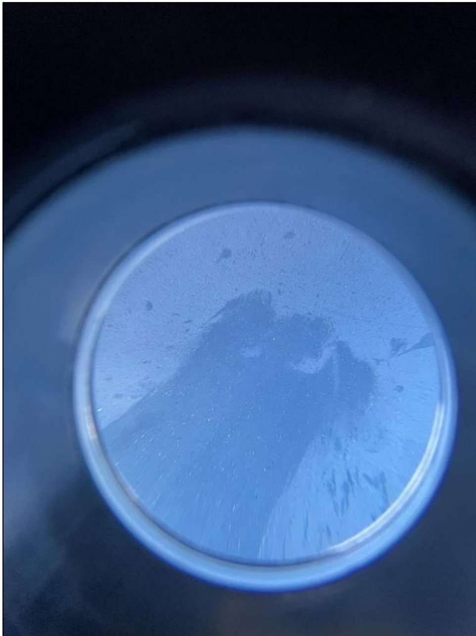
Photo 35: No coating disruptions were observed.
