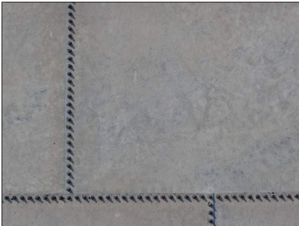
Photo 64: Tank wall surface exhibited no galvanization disruption.
