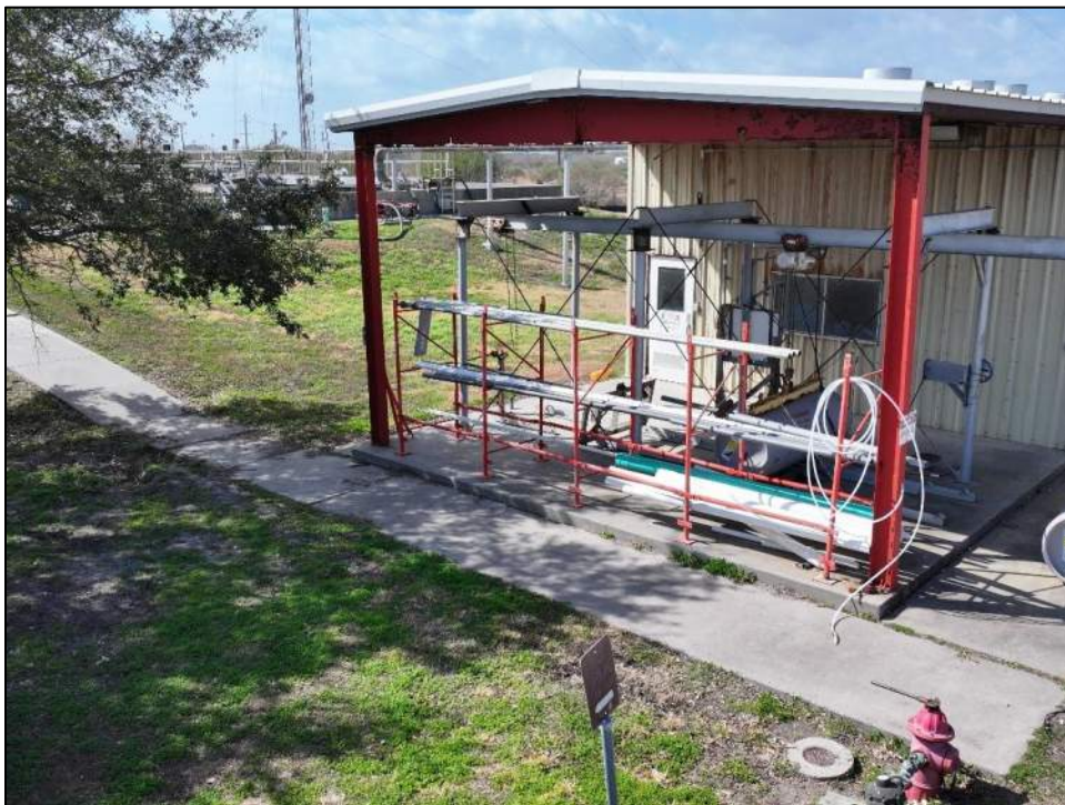
Photo 2: East canopy extension to the electrical building.
