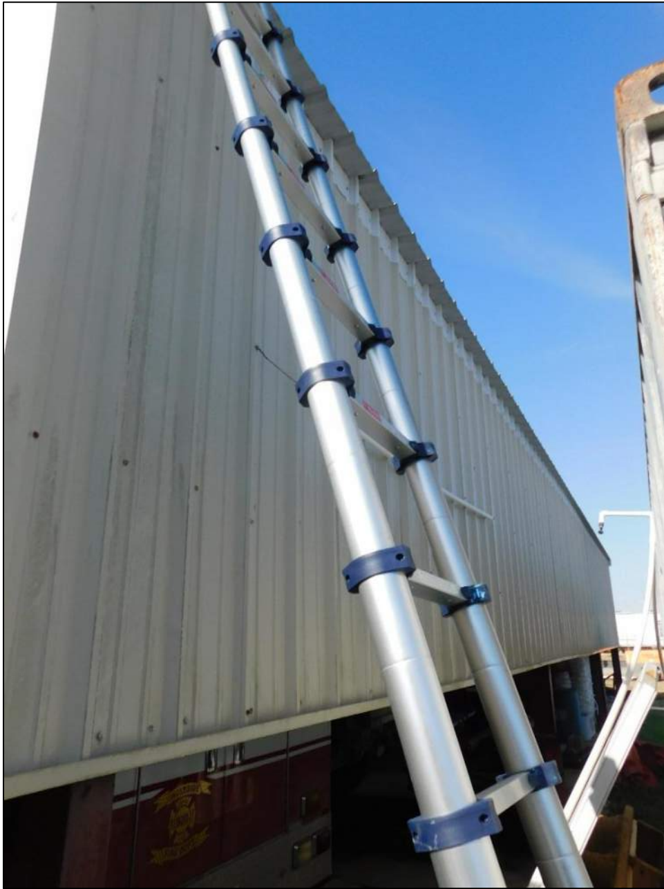
Photo 97: North elevation of the vehicle storage building.
