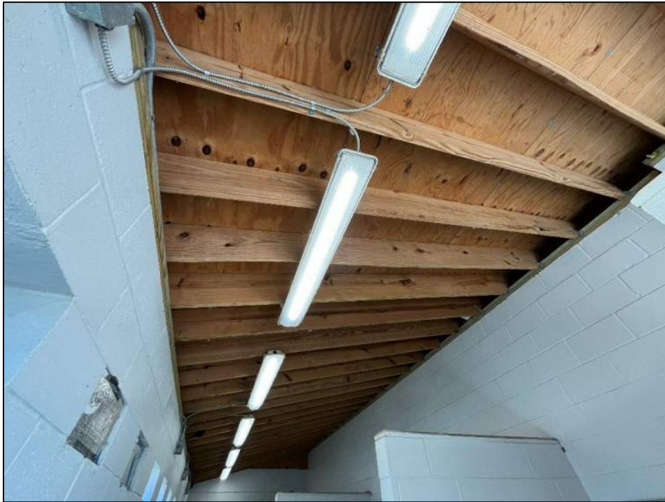
Photo 38: Restroom ceiling deck remained in sound conditions.
