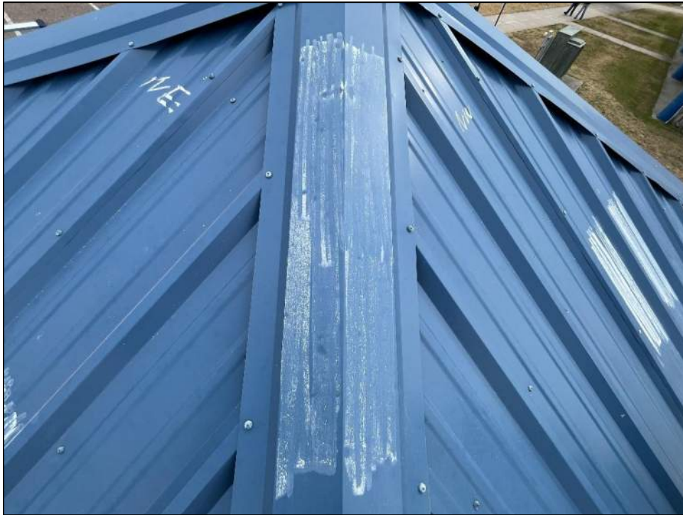
Photo 130: Similarly dented hip cap facing north.
