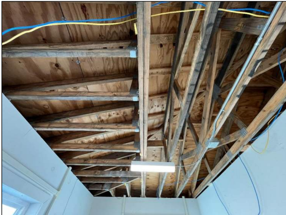
Photo 37: Plywood roof deck above the 2nd floor space were absent of recent moisture stains.
