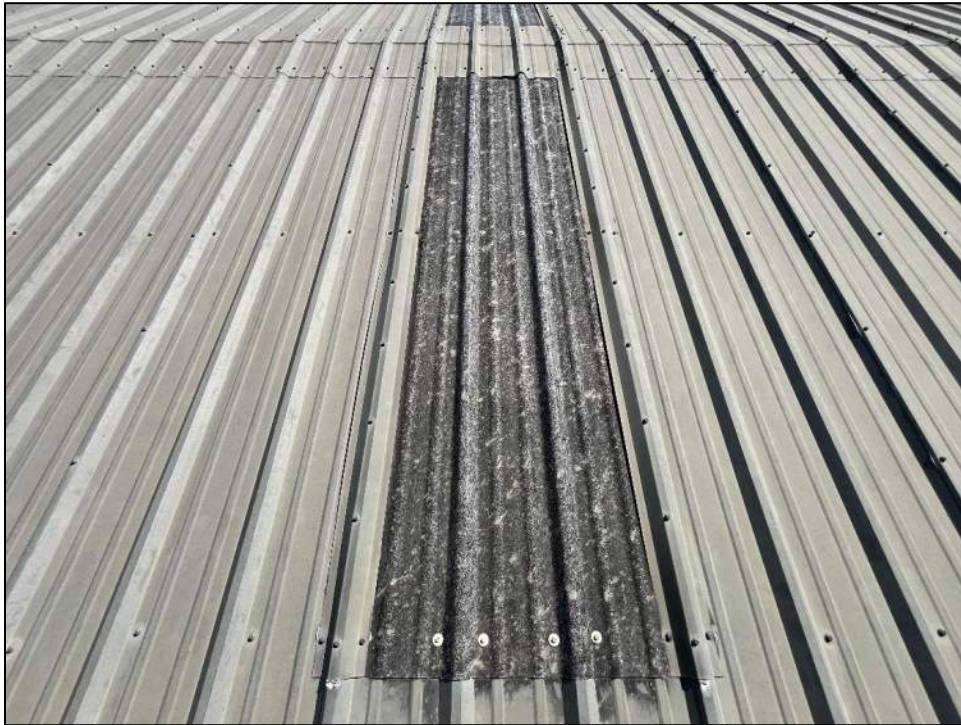
Photo 93: Skylight panels were not fractured at the spatters.
