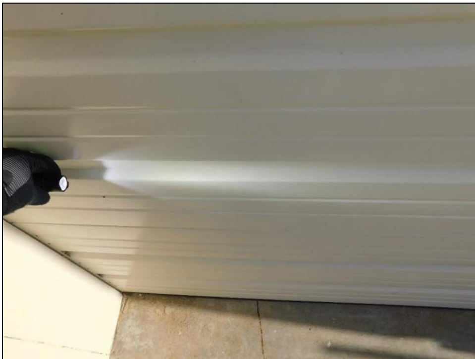
Photo 40: Rear roll-up doors exhibited no hail denting.
