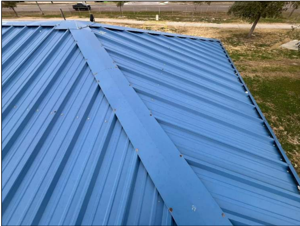
Photo 15: East and south slopes sustained significantly less hail denting.
