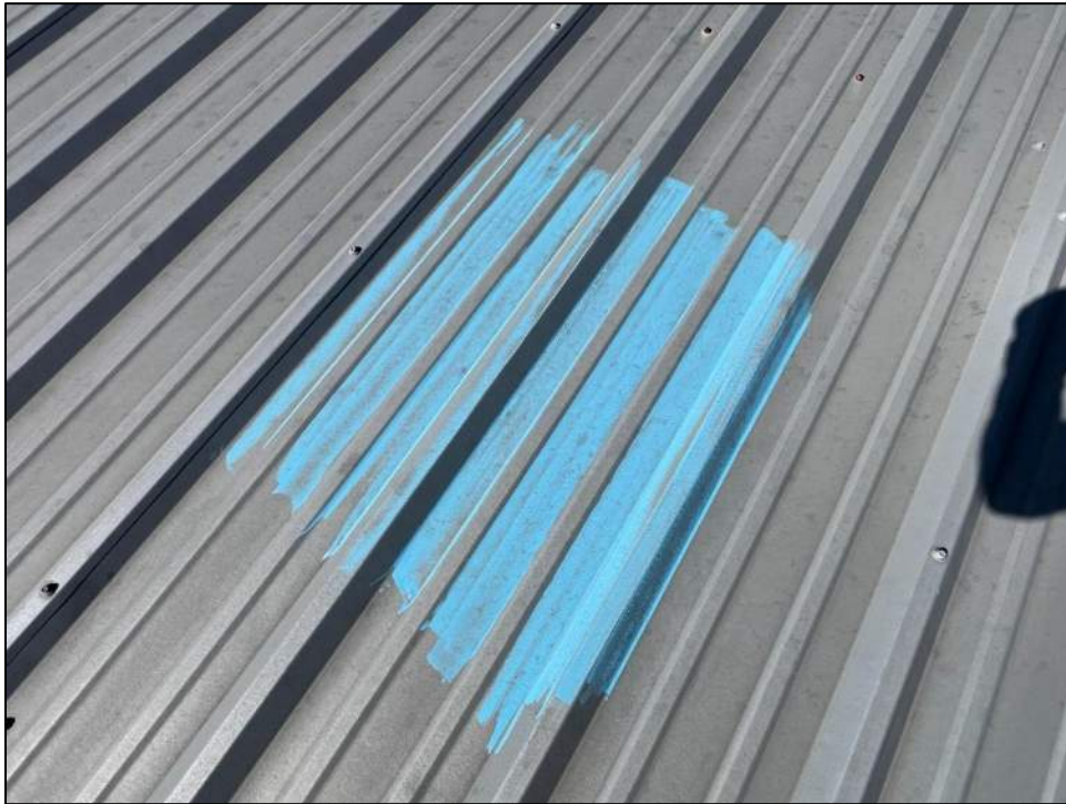
Photo 17: Denting consistent with hail impact was observed on the galvalume metal R-panel.
