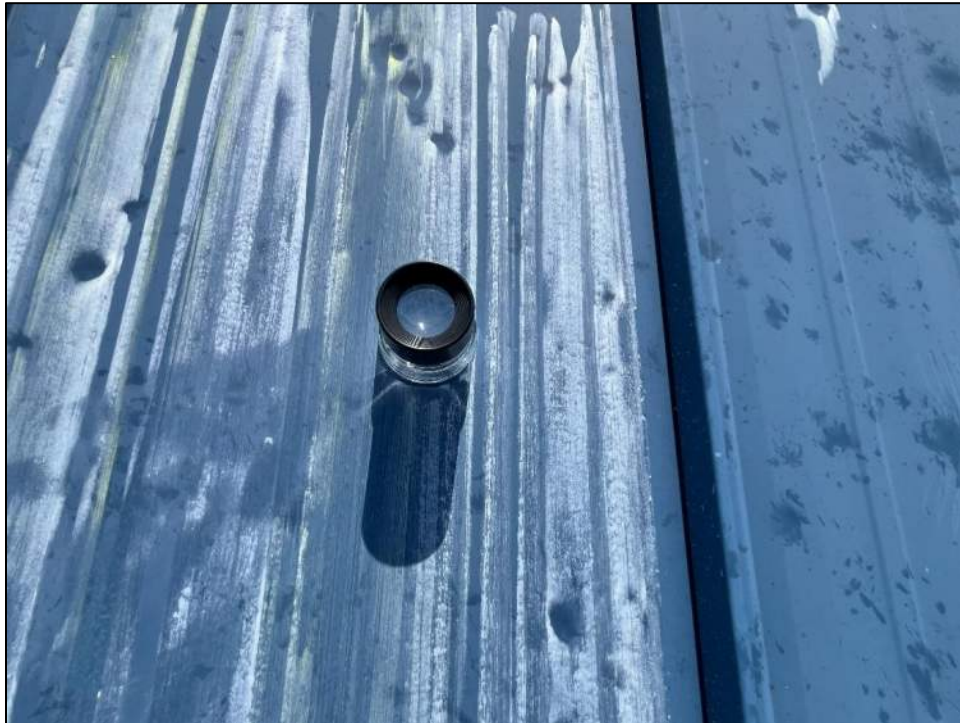
Photo 15: Microscope inspection indicated no coating disruption at hail dents or spatters.
