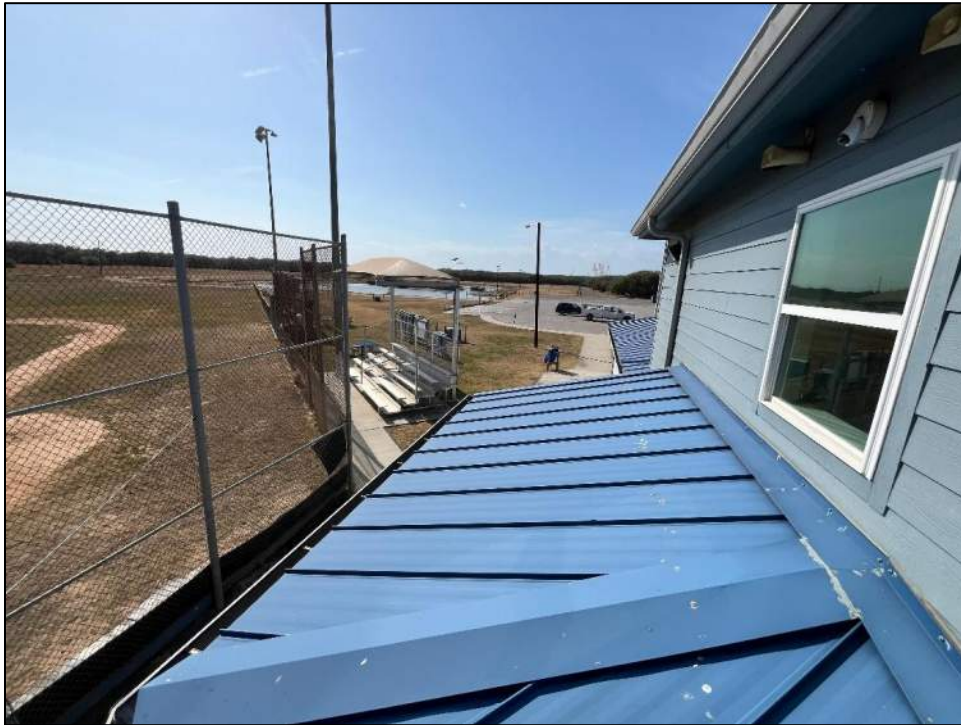
Photo 25: Lower half-octagonal apron roofing facing east were absent of hail spatters.
