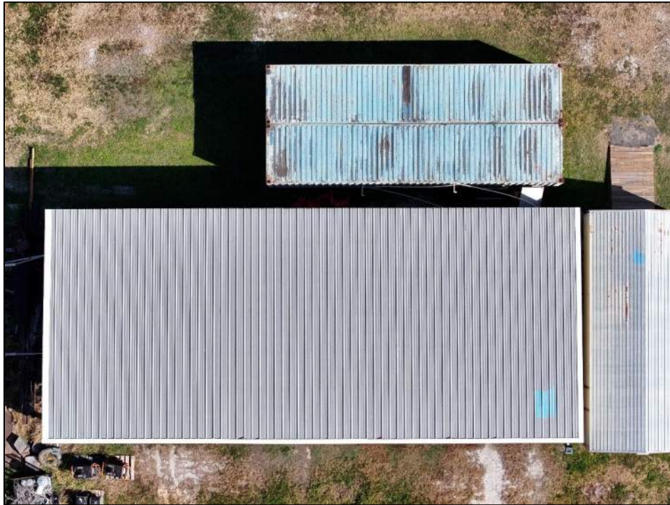
Photo 79: Overview of the storage shed metal roof.
