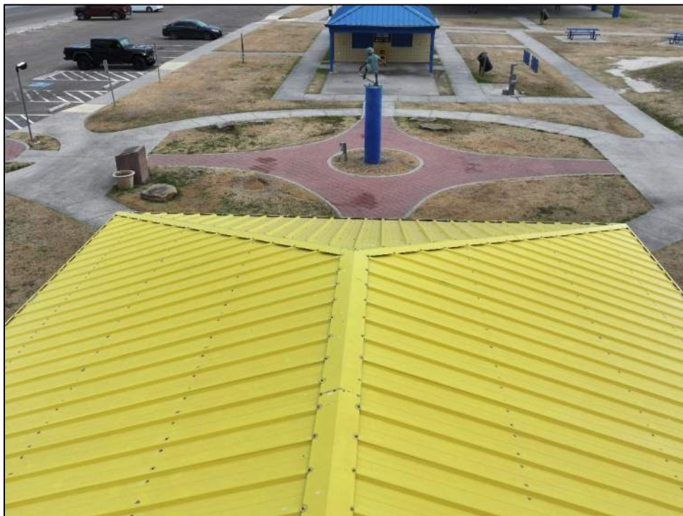
Photo 83: Ridge and hip caps were not displaced or uplifted.
