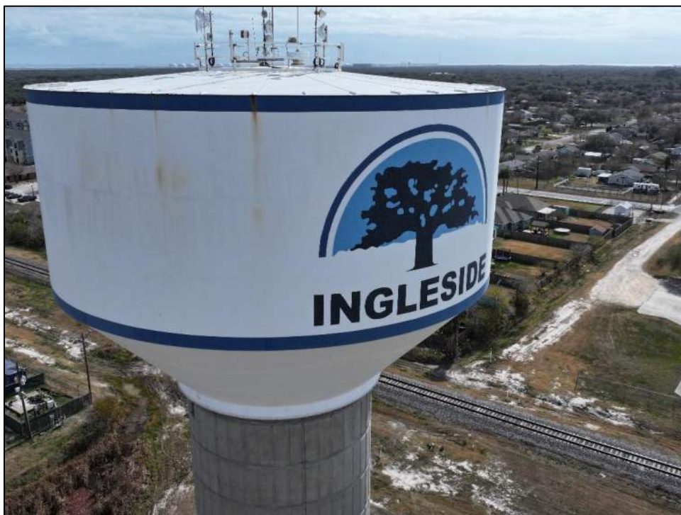
Photo 4: North elevation of the water tank.
