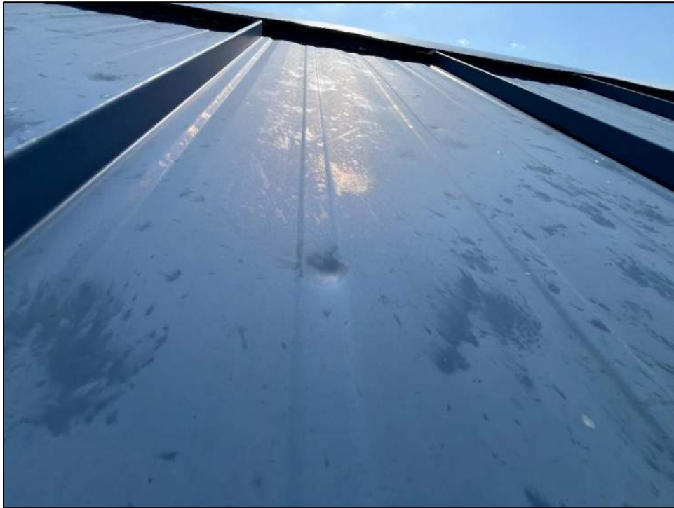
Photo 19: Microscope inspection indicated no coating disruption at hail dents or spatters.
