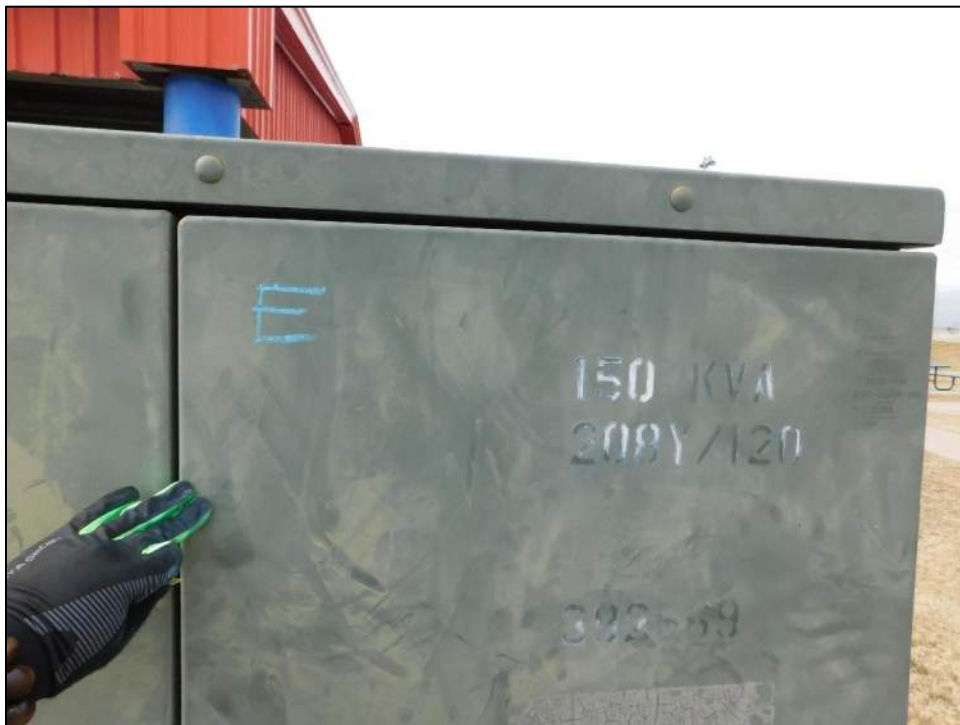
Photo 30: No hail spatters on east-facing surfaces.
