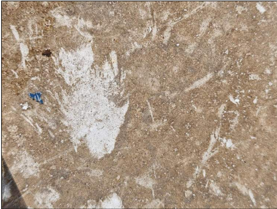
Photo 29: Close-up of a hail spatter.
