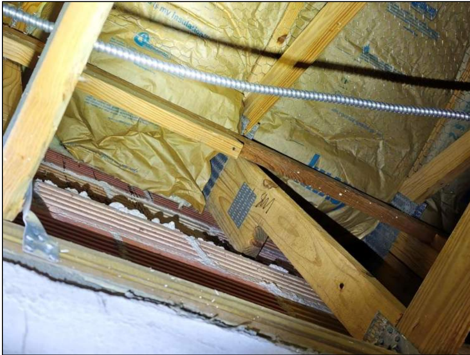
Photo 37: Roofing insulation exhibited no moisture distress above the stained ceiling tile.
