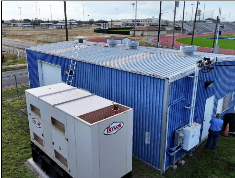
Photo 27: Overview of the pump station building in the Water Department complex.
