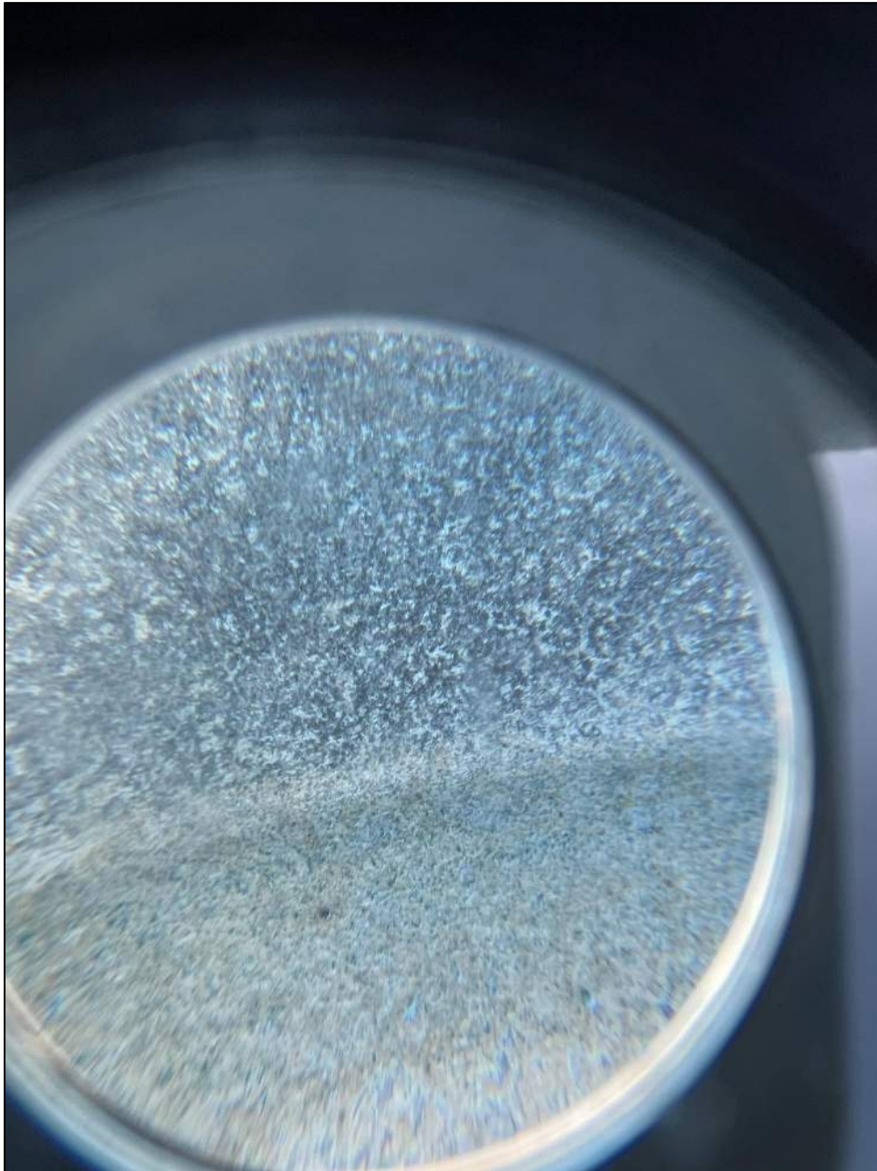
Photo 28: No coating disruptions were observed on the galvanized metal roof decking.
