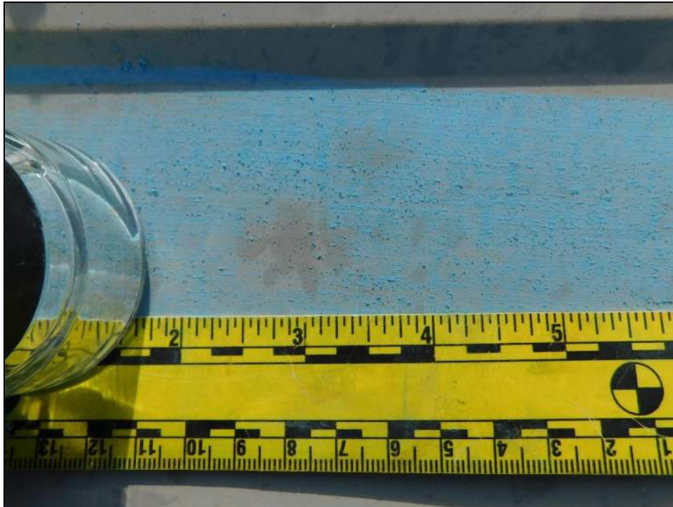
Photo 23: No coating disruptions were observed at the hail dents or spatters.
