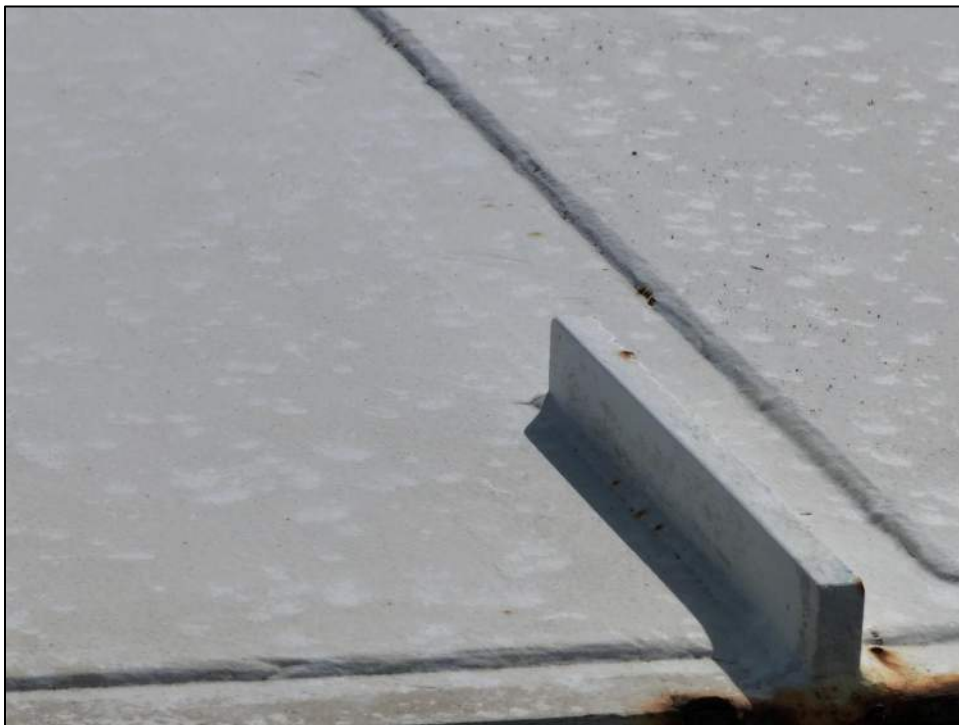
Photo 10: Rooftop spatters consistent with 1-inch hailfall.
