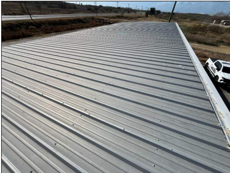
Photo 16: Roof overview (looking south).
