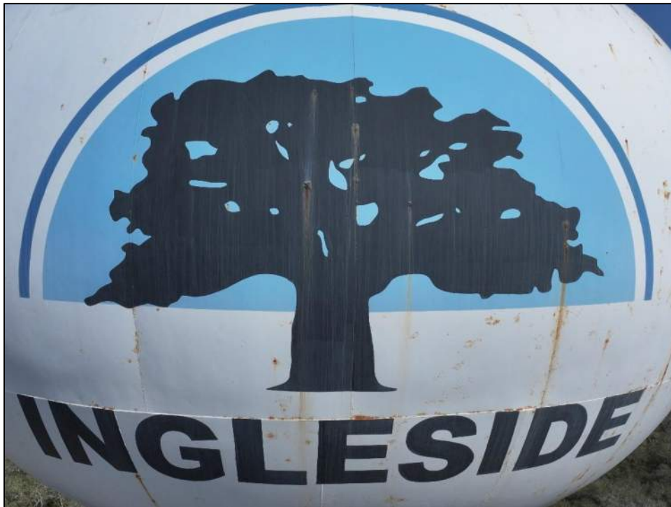
Photo 15: No coating disruption to painted surface.
