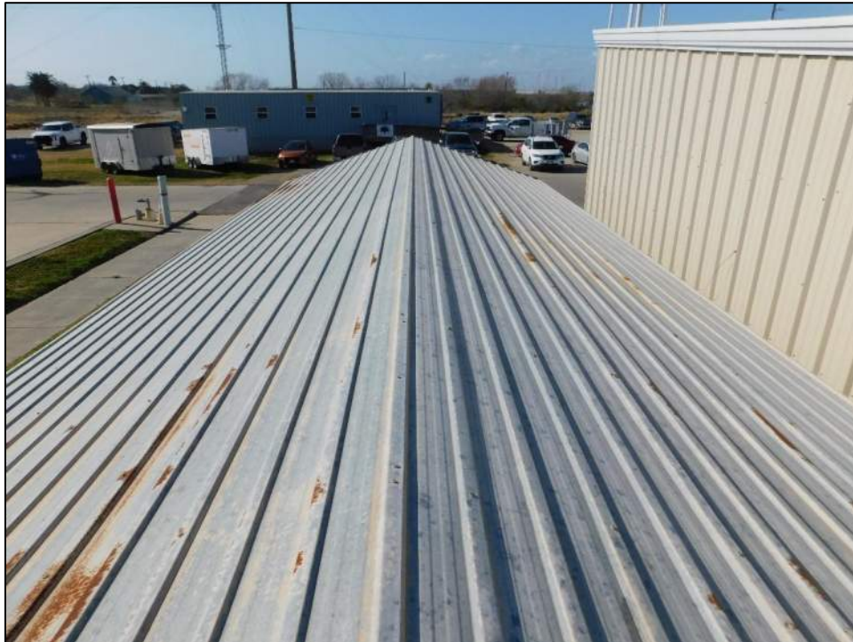
Photo 111: Roof of the storage building (relocated from east side of the police department building).
