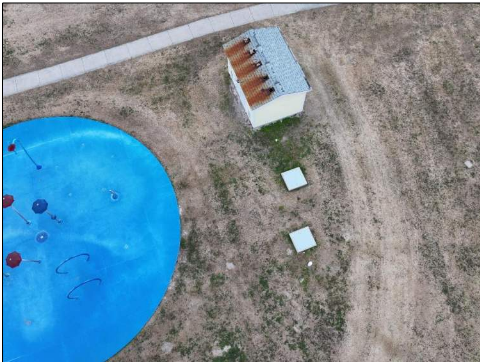
Photo 6: Deteriorated tool shed west of the splashpad.
