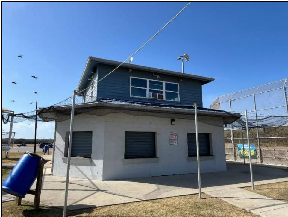
Photo 2: East (rear) elevation).
