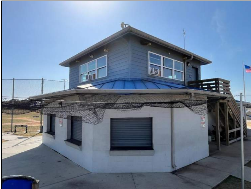
Photo 3: Rear and north elevations. Windowpanes remained intact. No displaced gutters or downspouts were observed.
