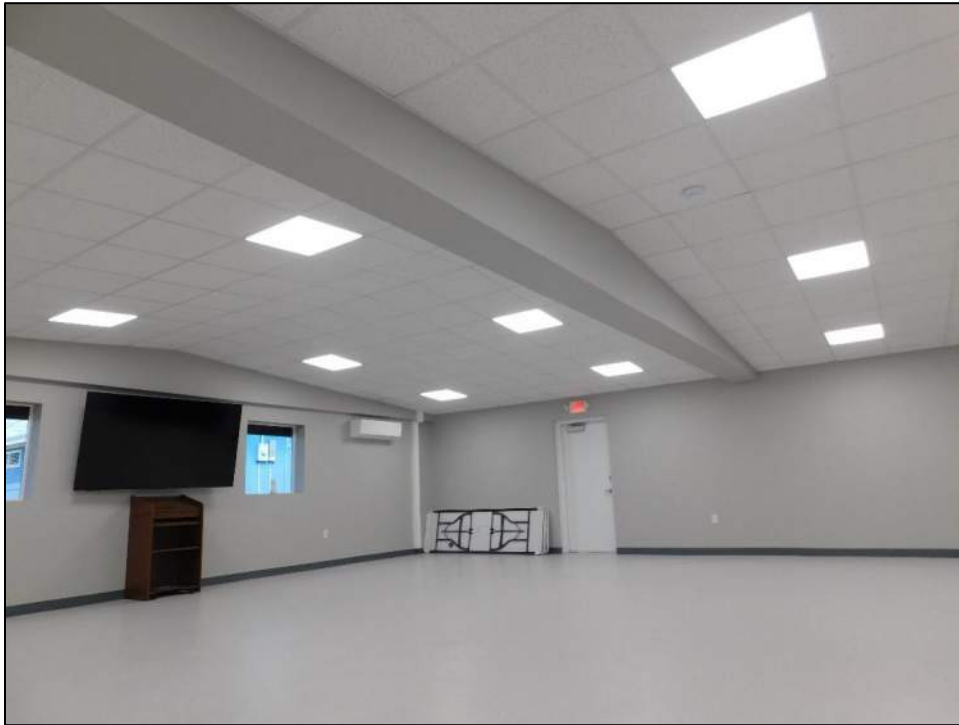
Photo 30: Interior finishes remained in sound condition.
