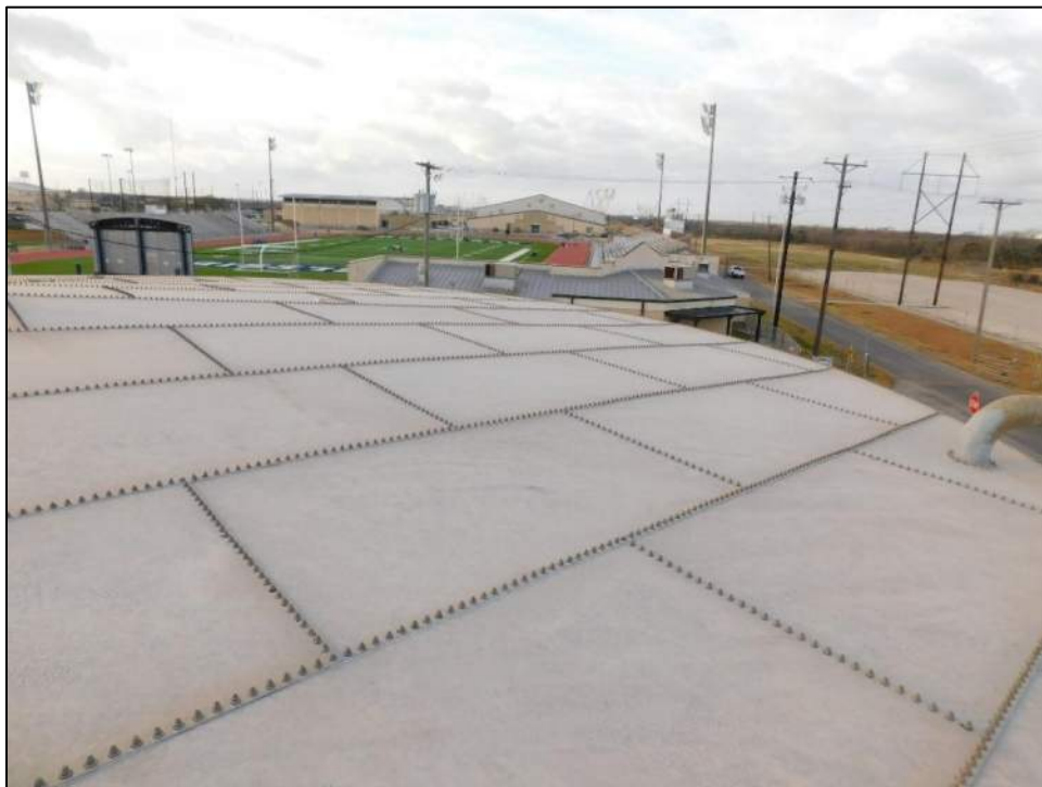
Photo 69: Roof top of tank remained structurally intact.
