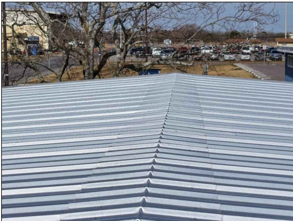
Photo 19: Ridge panels was intact.
