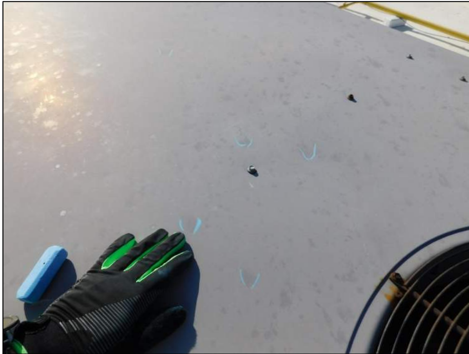
Photo 57: No denting was observed on the HVAC unit casing on the roof.
