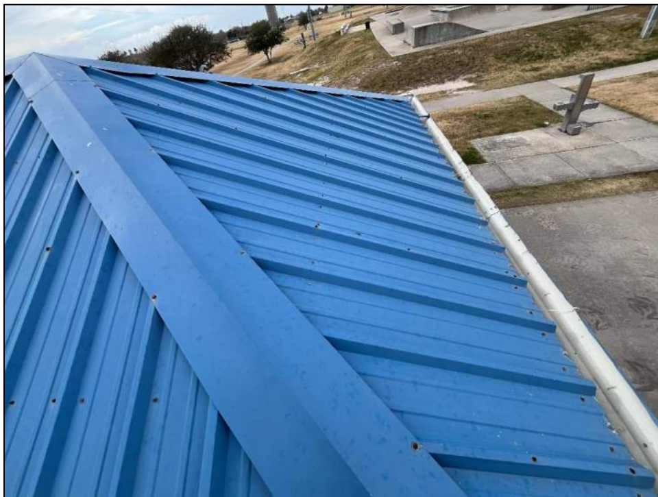
Photo 67: North slope and ridge cap were not deformed or displaced.
