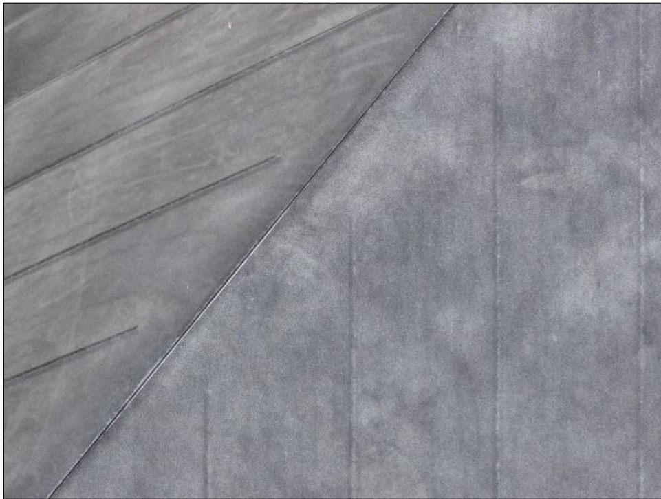
Photo 106: The roof is made of steel plates. No hail impact indentations were observed.
