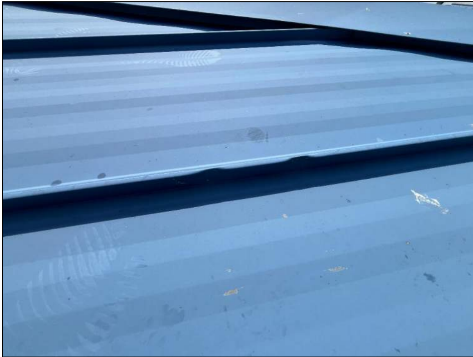
Photo 27: Typical seam crimp areas irrelevant to storm effects.
