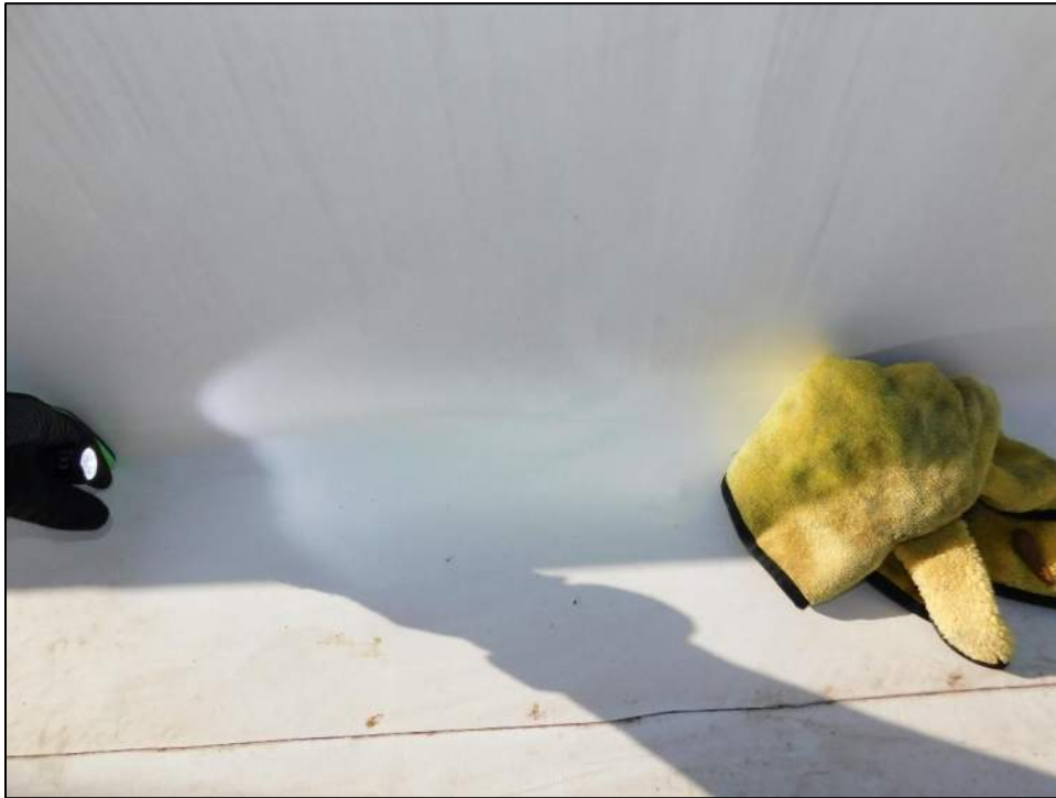
Photo 51: Parapet bases facing the direction of the hail impact were closely inspected after surface cleaning for hail impact.
