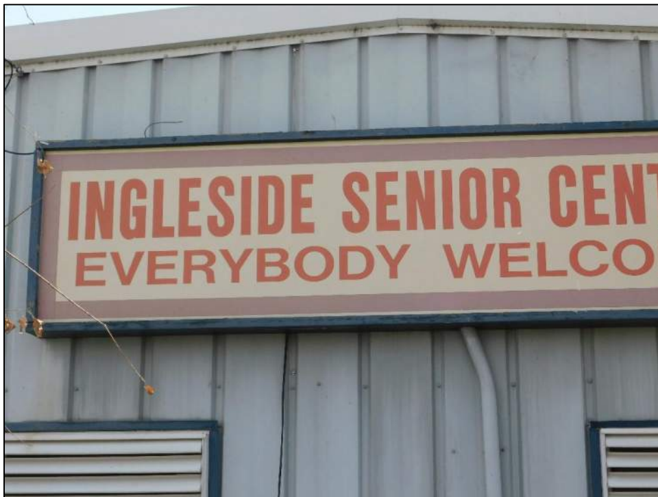
Photo 8: No signage impact damage observed on the wall sign on west elevation.
