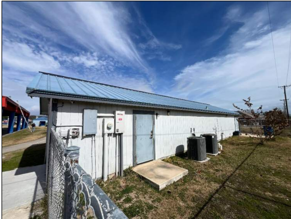
Photo 3: South (rear) elevation.
