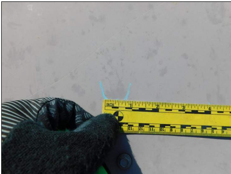
Photo 58: maximum hail spatter marks reflect 1.0-inch hail at the site.
