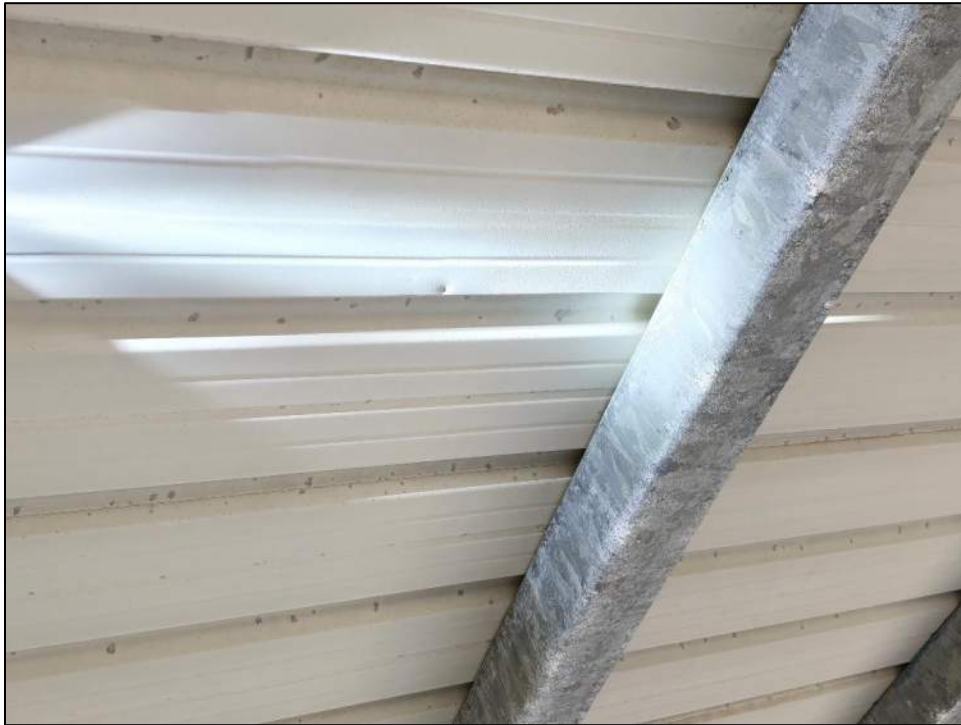
Photo 88: Upward denting on the east slope (inconsistent with hail impacts).
