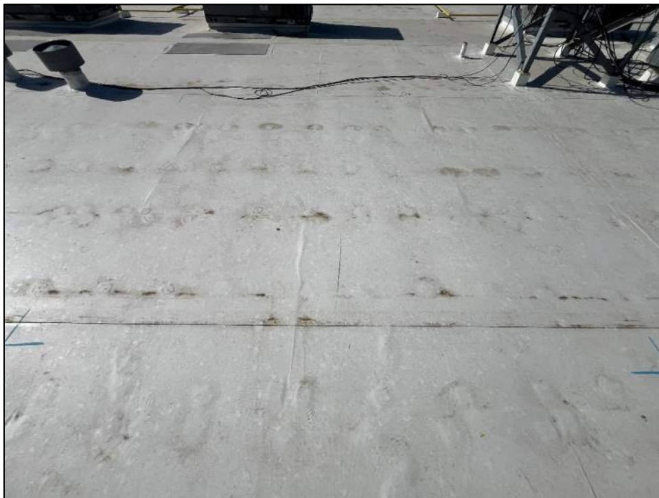
Photo 73: Test square on the PVC roof above the police department identified no hail impact fractures to the membrane.
