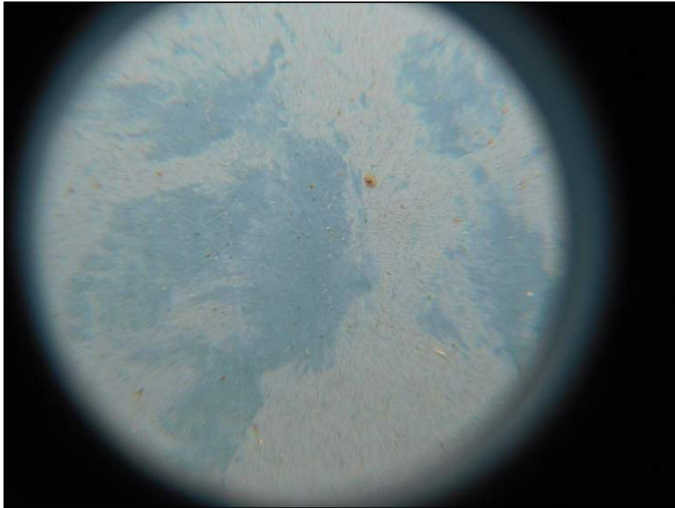
Photo 13: No coating disruption was present at the hail spatter.
