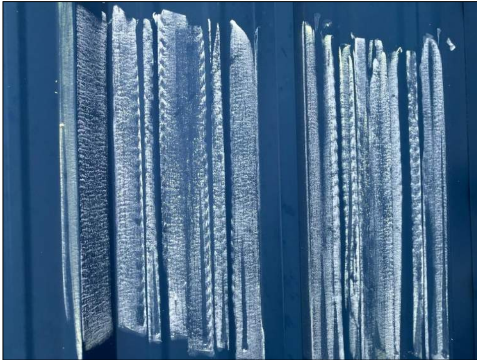
Photo 134: Hail denting on south slope was minimum compared to west and north slopes.
