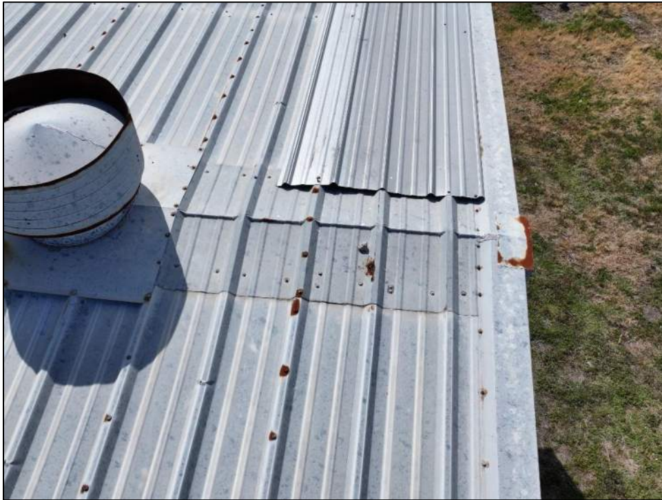
Photo 20: Partial panel (incompatible profile) overlay.
