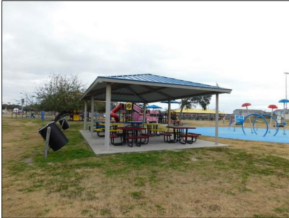
Photo 1: East elevation of the splashpad pavilion.
