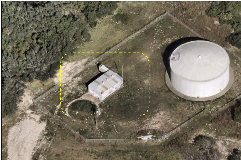
Figure 2 – Structure 002-001, Pump Station: November 9, 2024. Source: Nearmap®.
