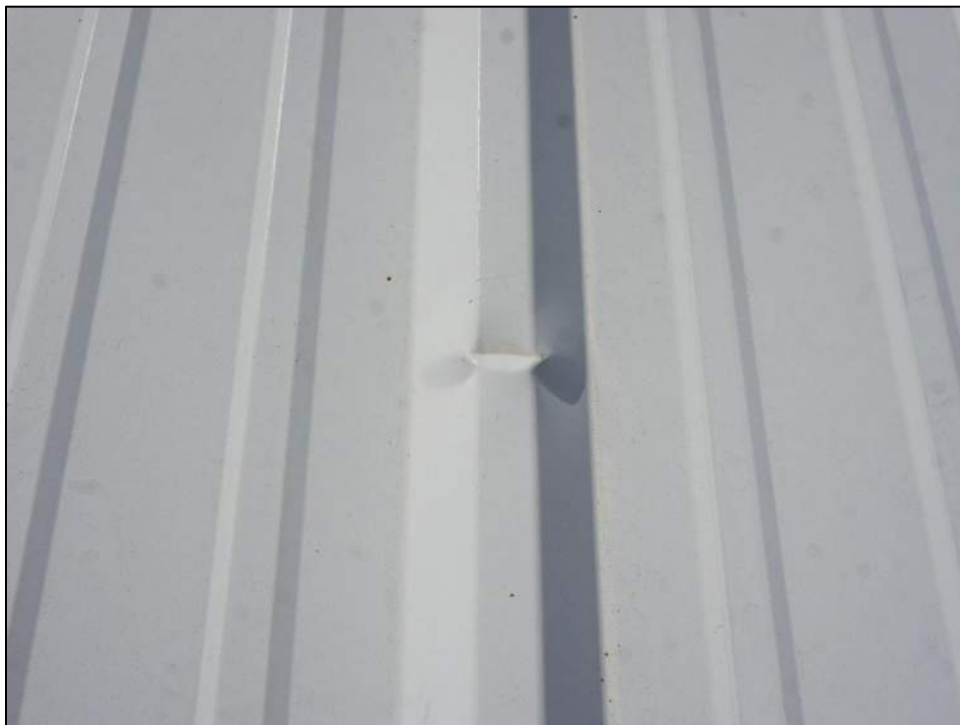
Photo 26: Roof panel rib creases inconsistent with effects of hail impact.
