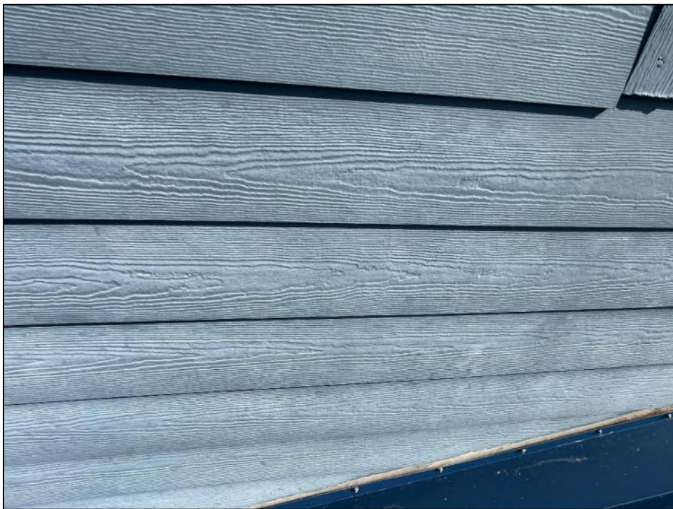
Photo 18: No impact chipping was observed on the painted lap siding along south elevation (west elevation).
