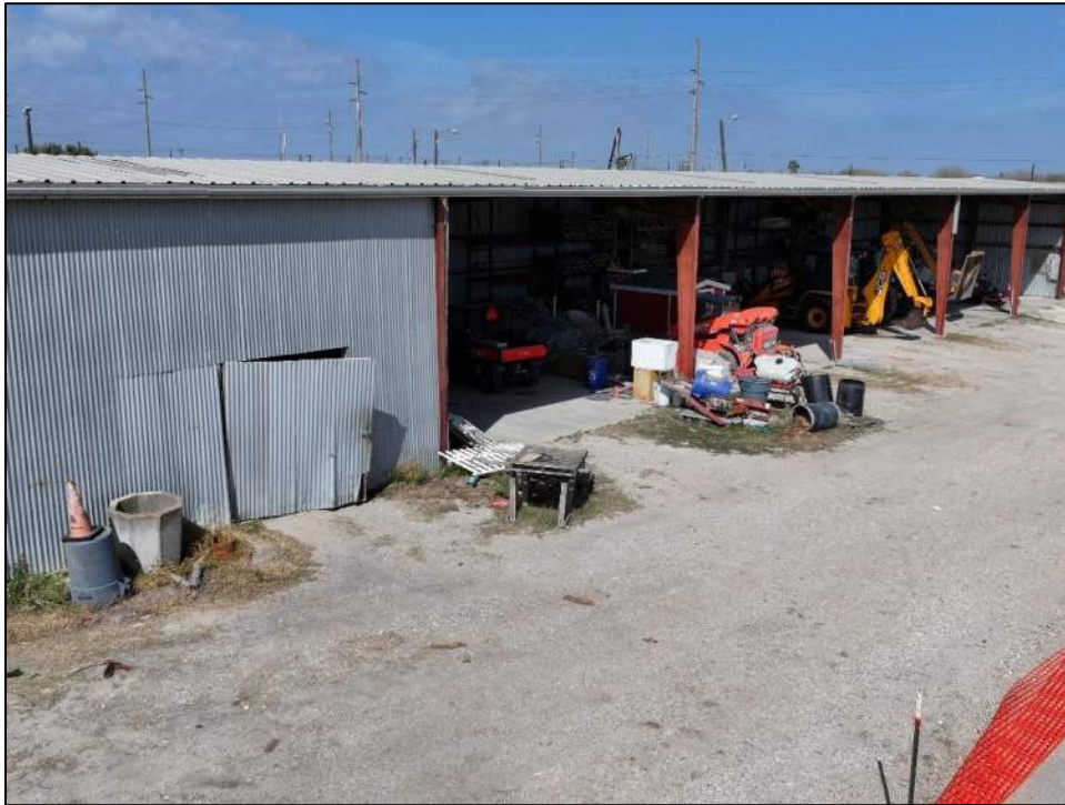
Photo 75: East elevation of the vehicle storage building.
