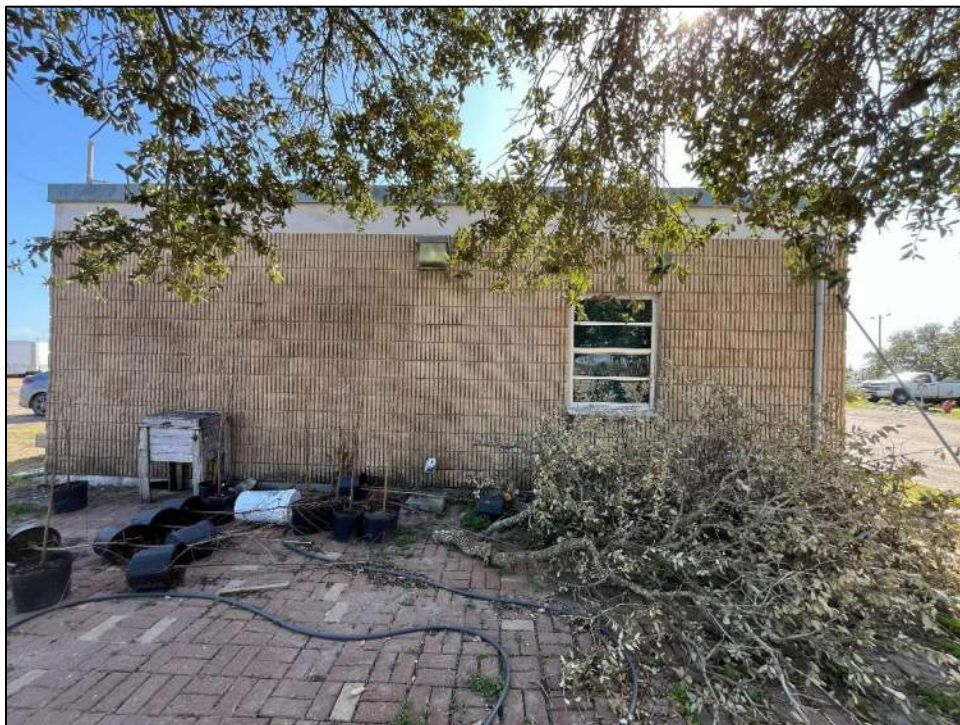
Photo 37: West elevation. Windows remained intact.
