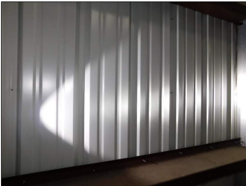
Photo 12: No hail denting visible on inside of west or north wall panels.
