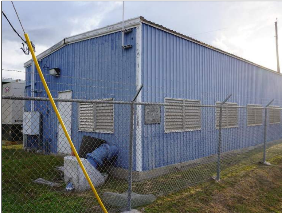
Photo 29: West and south elevations.
