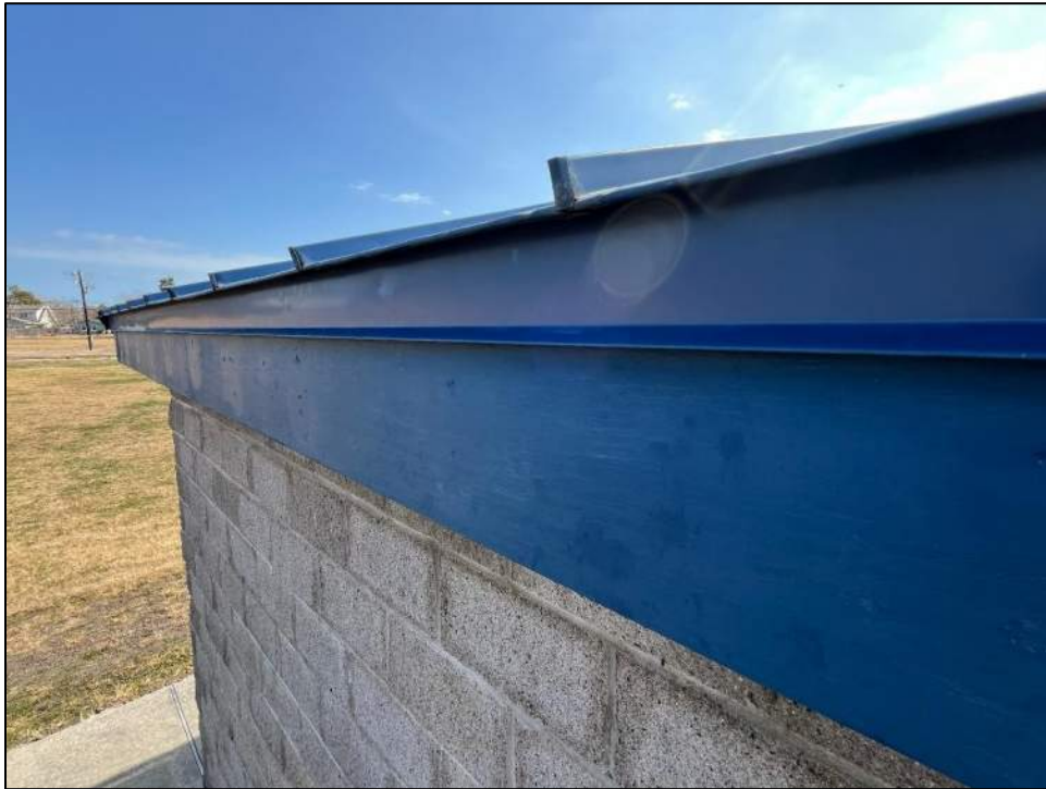
Photo 9: West gable end rake drip edges remained securely attached.
