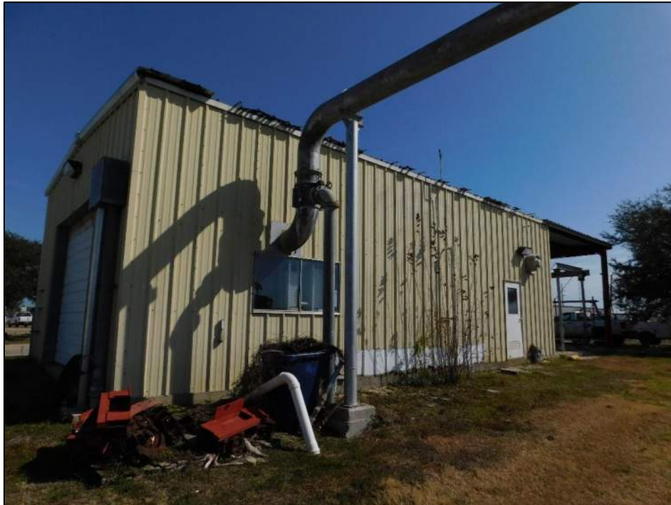
Photo 5: Rear (south) elevation.
