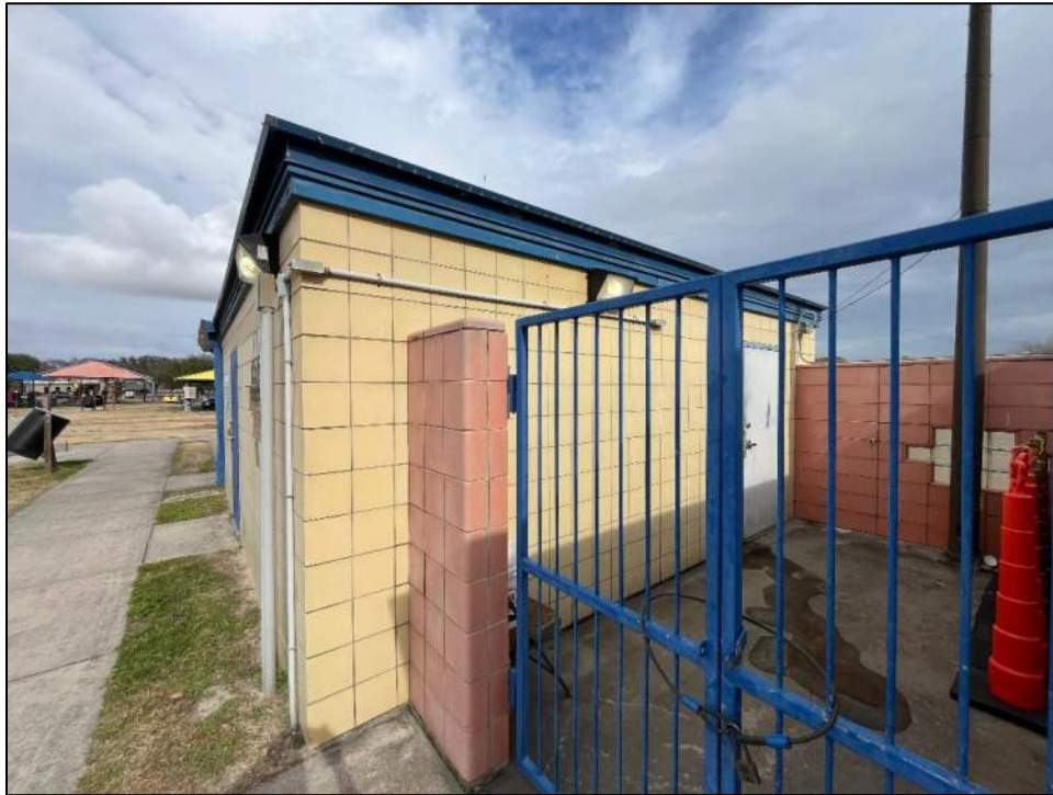
Photo 64: South (rear) elevation.
