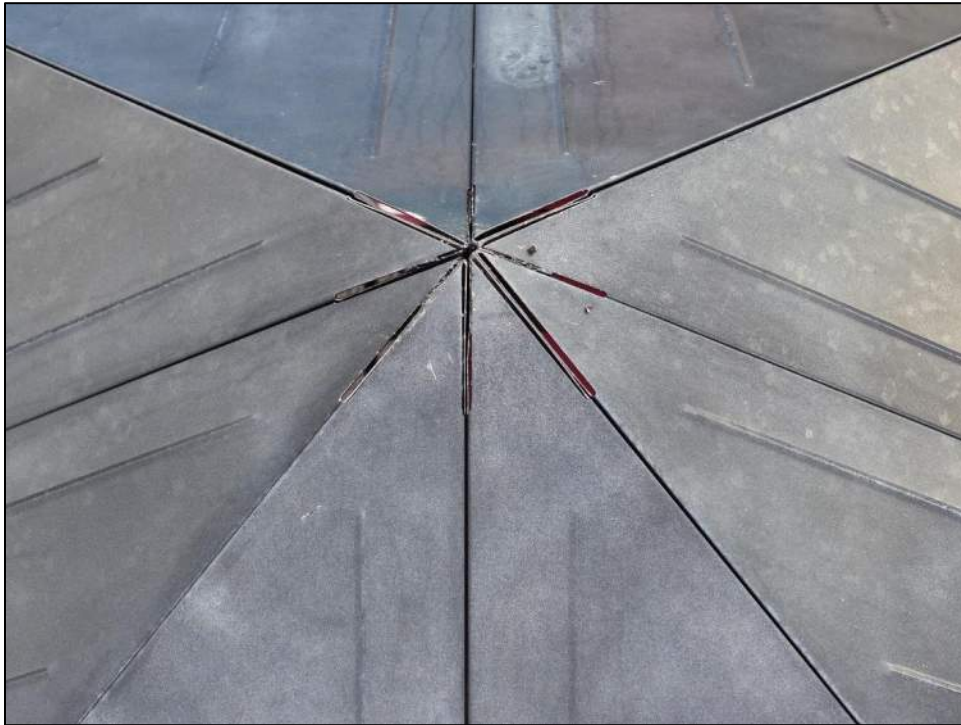
Photo 105: The roof is made of steel plates. No hail impact indentations were observed.
