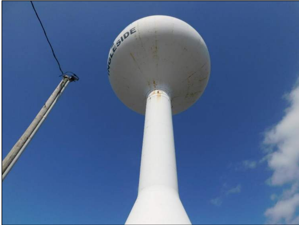
Photo 1: Upward view of the tank.
