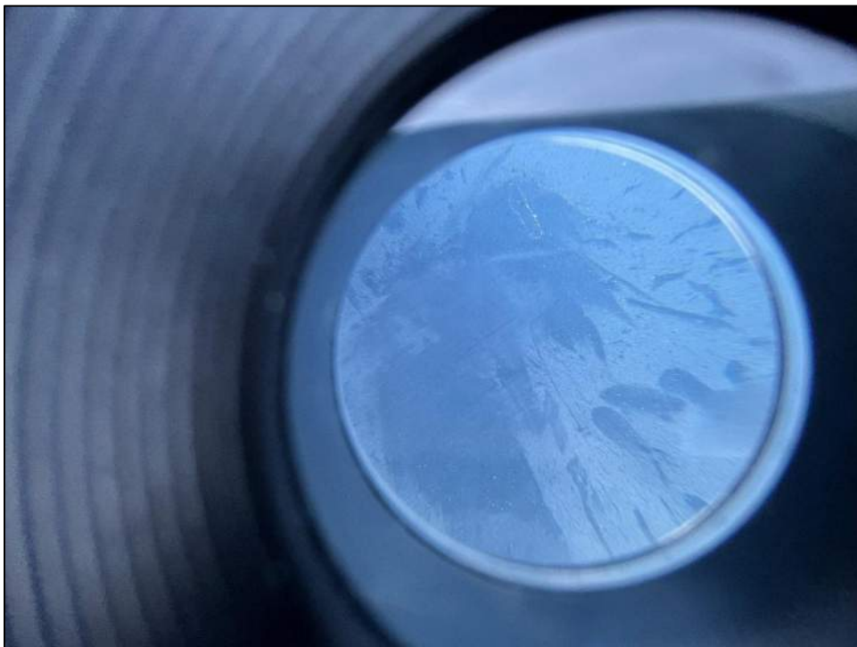
Photo 34: No coating disruptions were observed.
