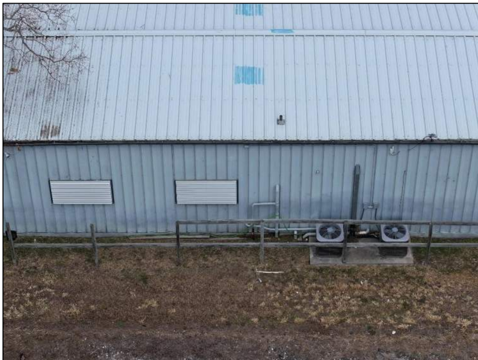
Photo 4: South (rear) elevation.
