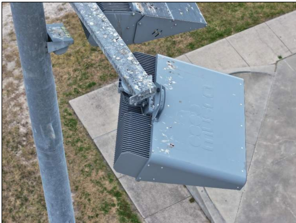
Photo 22: Nearby pole lights were not factured or dented.
