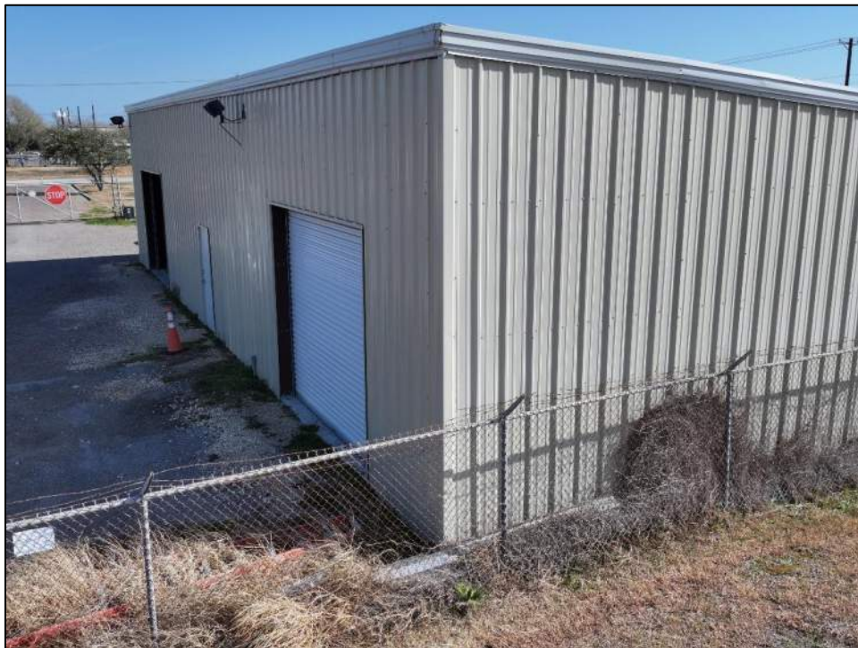
Photo 2: West elevation had 2 roll-up doors.
