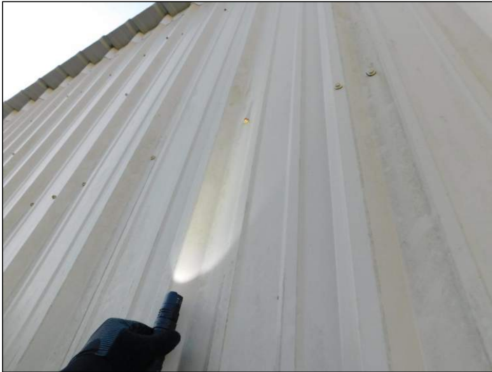
Photo 99: No hail indentations observed on the metal R-panel walls in the north elevation.
