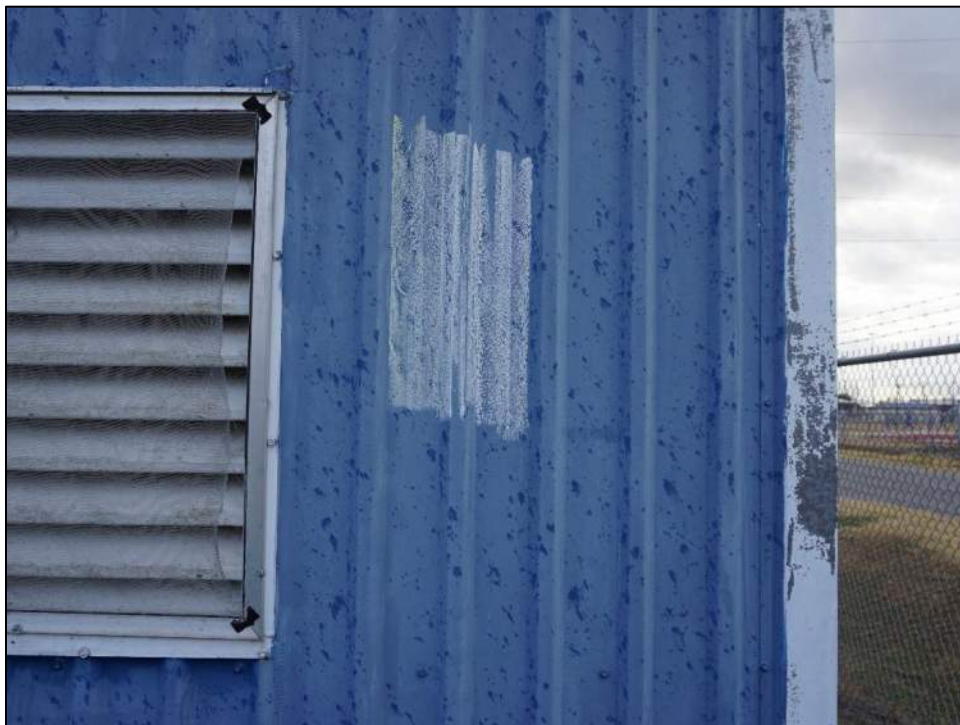
Photo 36: No hail denting was observed on the west wall. Existing coating exhibited aged-related peel.
