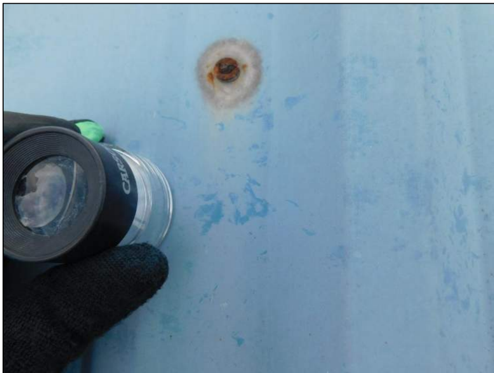
Photo 12: Close examination of a large spatter on the north slope.
