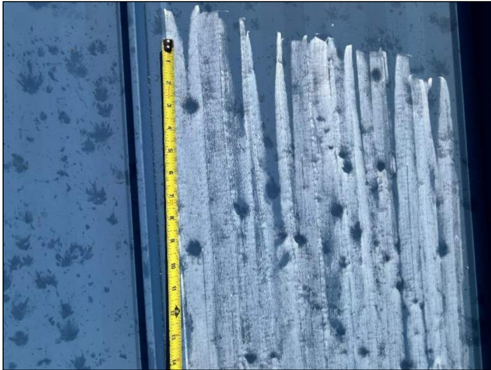
Photo 13: Maximum Hail denting measured 1/2 inch in inner diameter.
