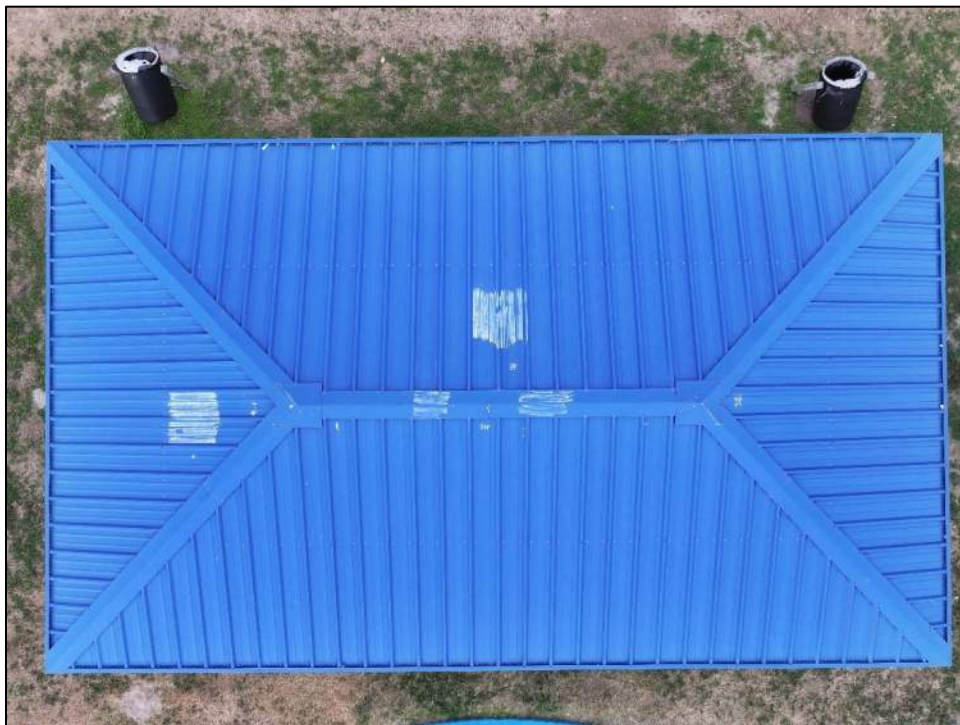
Photo 4: Top-down view of roof.
