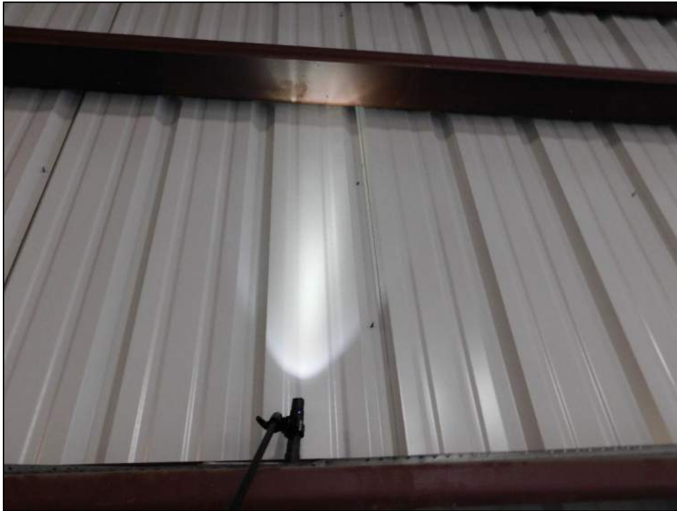
Photo 13: No hail denting visible on inside of west or north wall panels.
