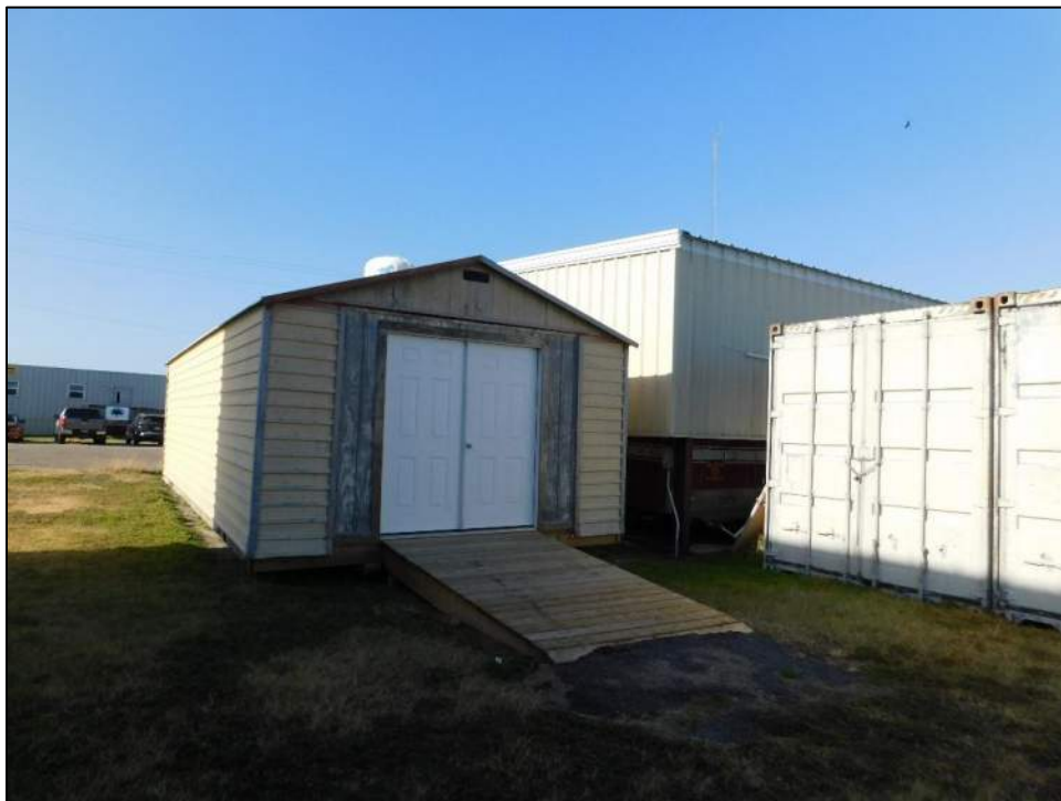
Photo 80: North (front) elevation of a storage building west of the fire department and police station building.
