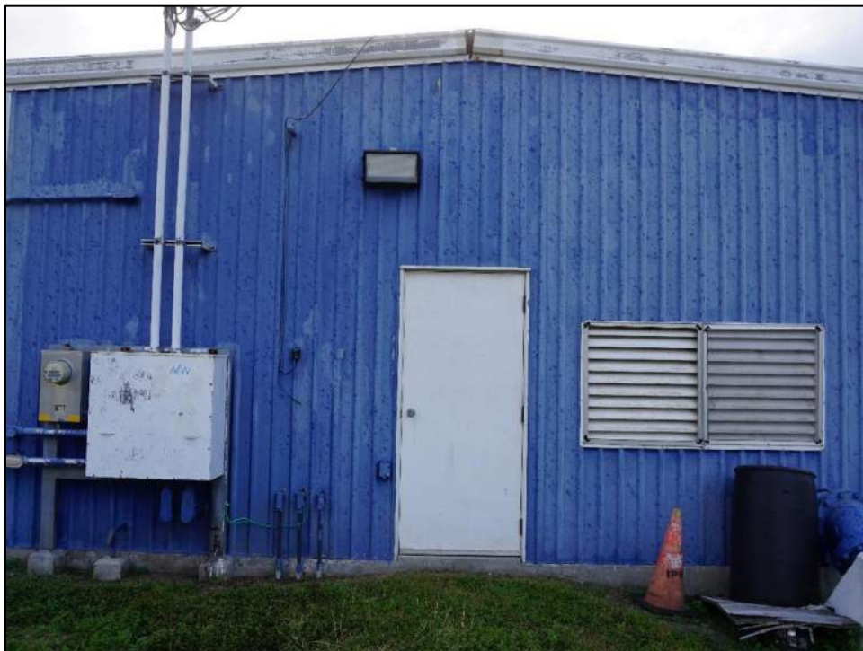
Photo 32: West elevation exhibited dense spatter marks.
