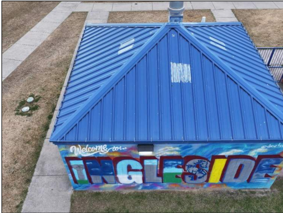
Photo 119: Restroom building - top-down overview.
