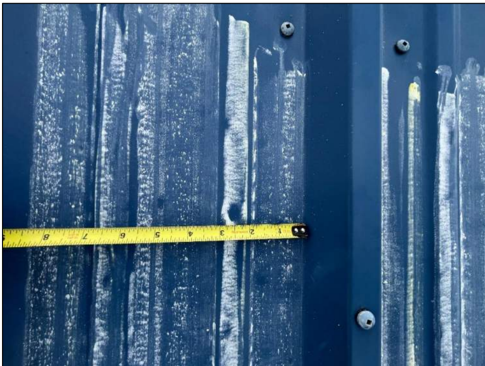
Photo 128: Hail denting on north slope had maximum inner diameter of less than 1/2 inch consistent with impact from 1-inch hail.
