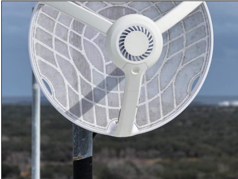
Photo 13: Rooftop appurtenances were not fractured by hail impact.
