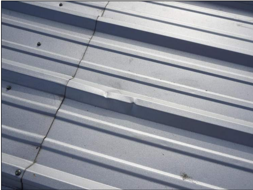
Photo 20: Typical creased roof deck ribs consistent with foot traffic and irrelevant to hail.
