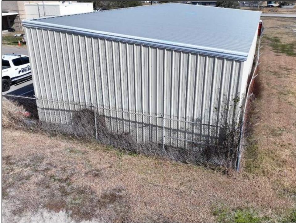
Photo 1: South (southwest) elevation of the police storage building.
