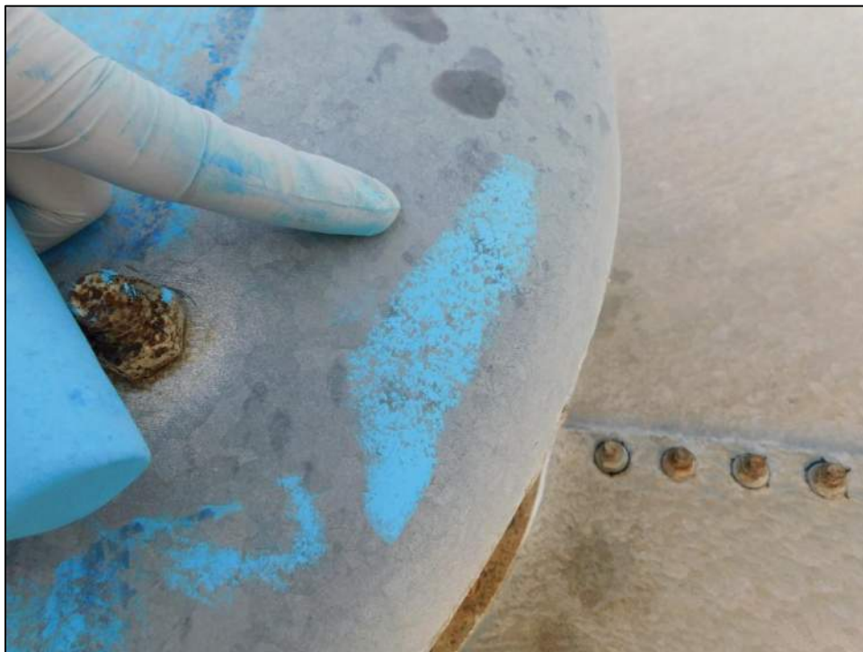
Photo 73: Tank roof vent was not dented
