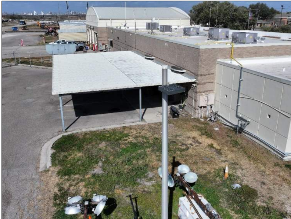
Photo 33: Rear elevation of the police station building.
