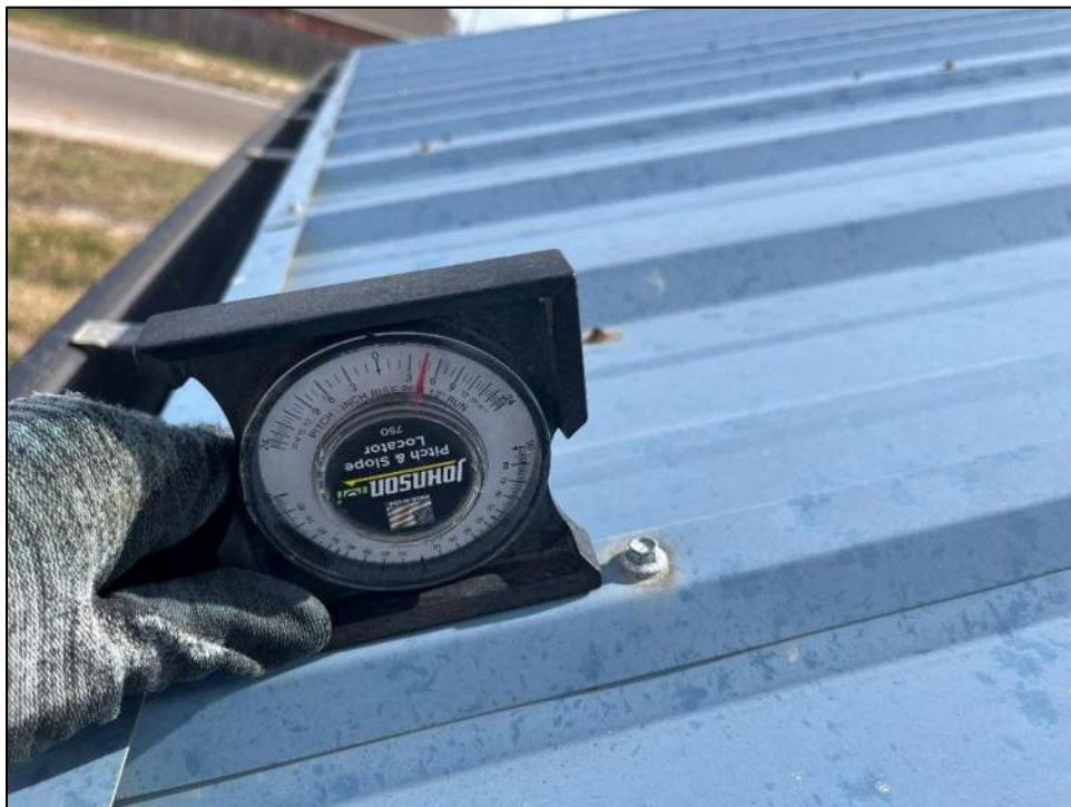
Photo 14: 4.5:12 roof pitch.
