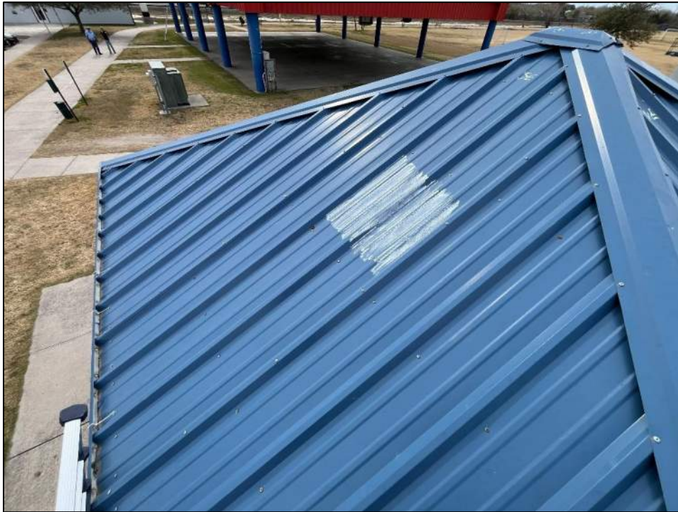
Photo 125: East slope. Eave closure remained intact.
