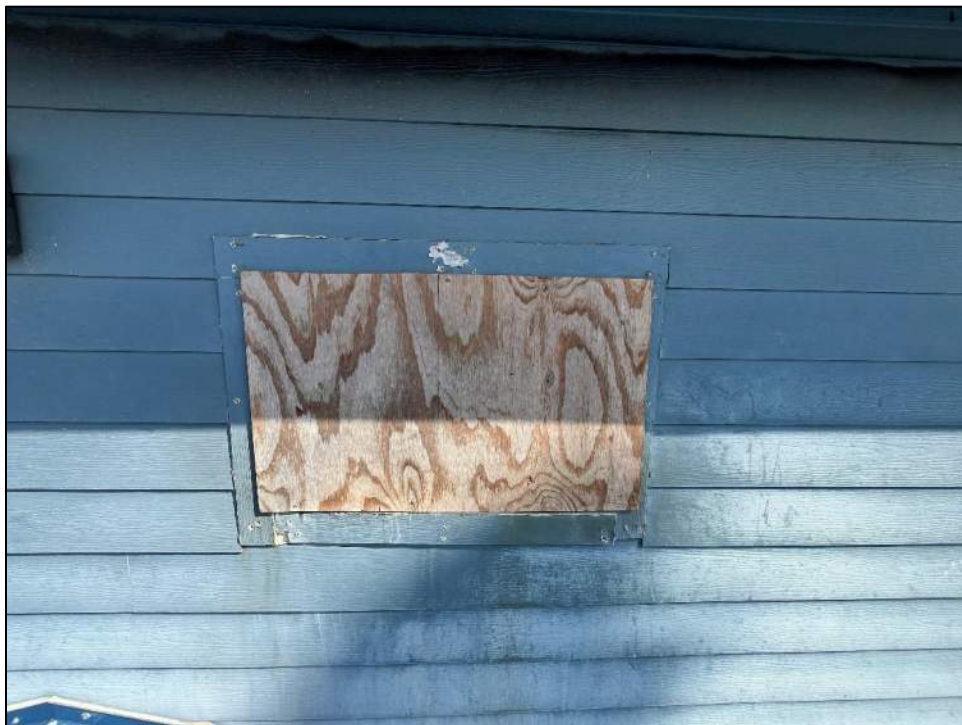
Photo 20: Pre-existing plywood boarding of a formerly AC-housing window on west wall.
