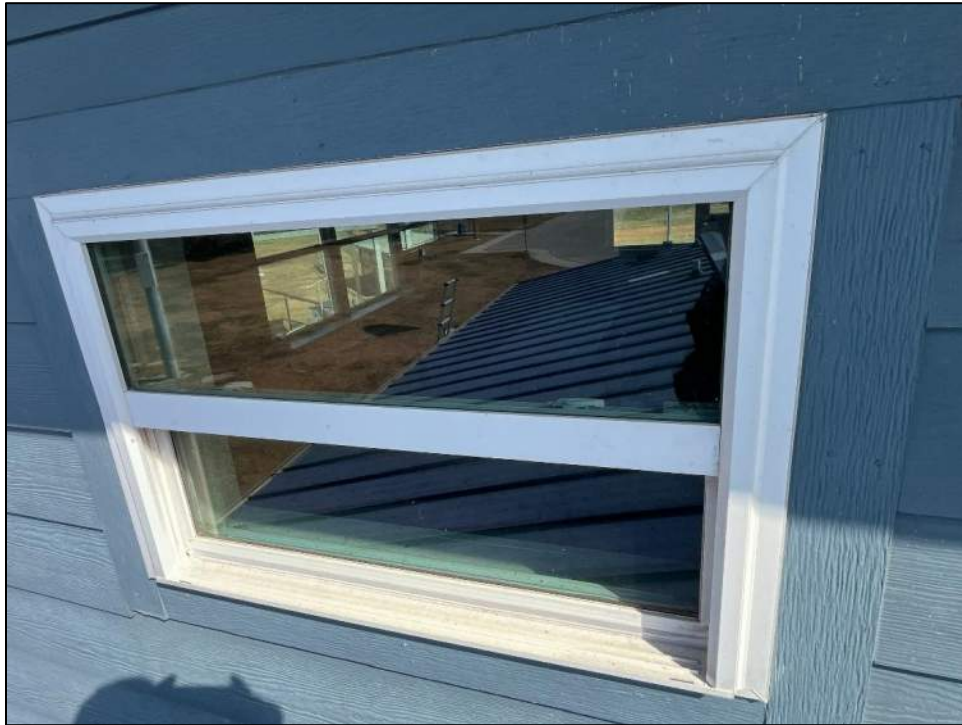
Photo 19: Windows remained intact (west elevation).
