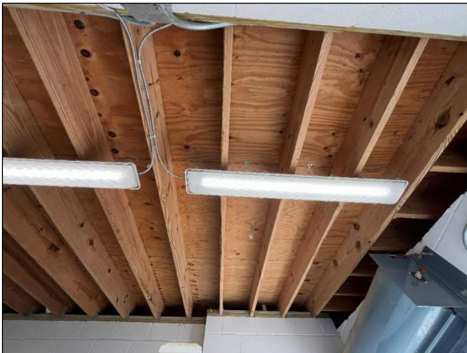
Photo 39: Plywood roof deck above the restroom were absent of recent moisture stains.
