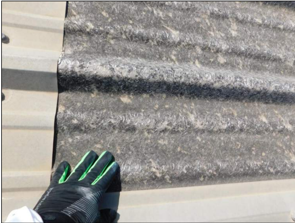
Photo 91: Skylight panels were not fractured at the spatters.
