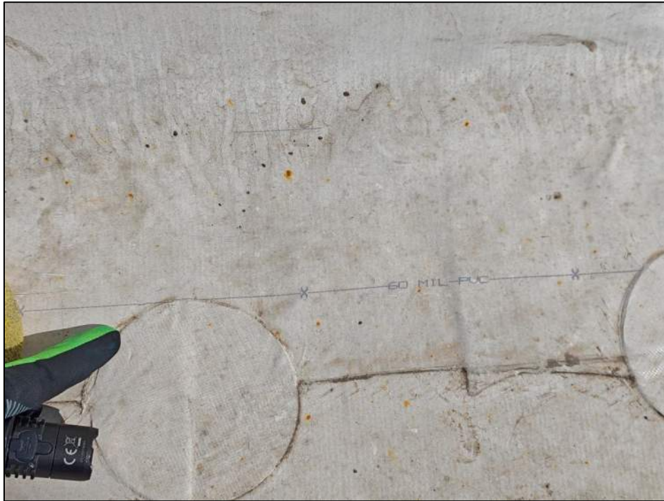
Photo 27: The roof was covered with 60 mil PVC membrane roofing.
