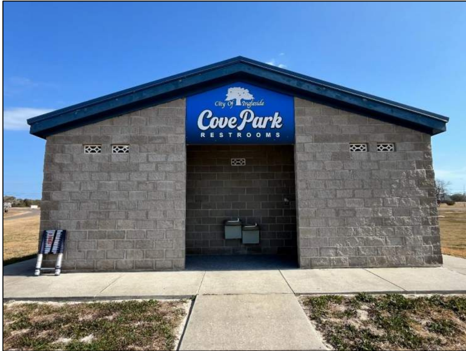
Photo 1: West (front) elevation.
