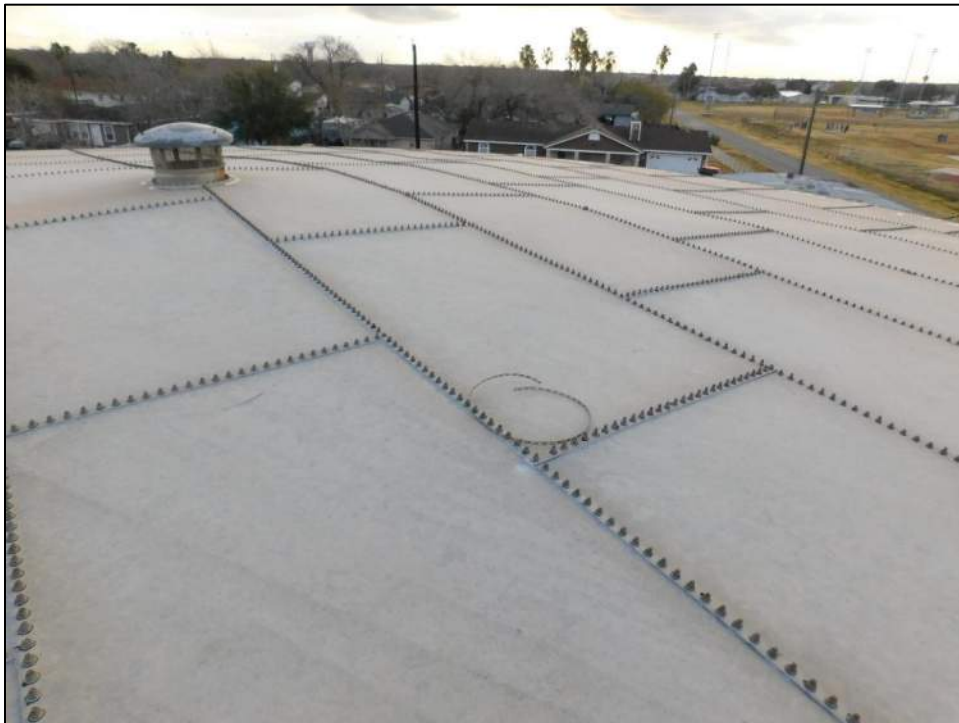
Photo 71: Tank roof remained structurally intact.
