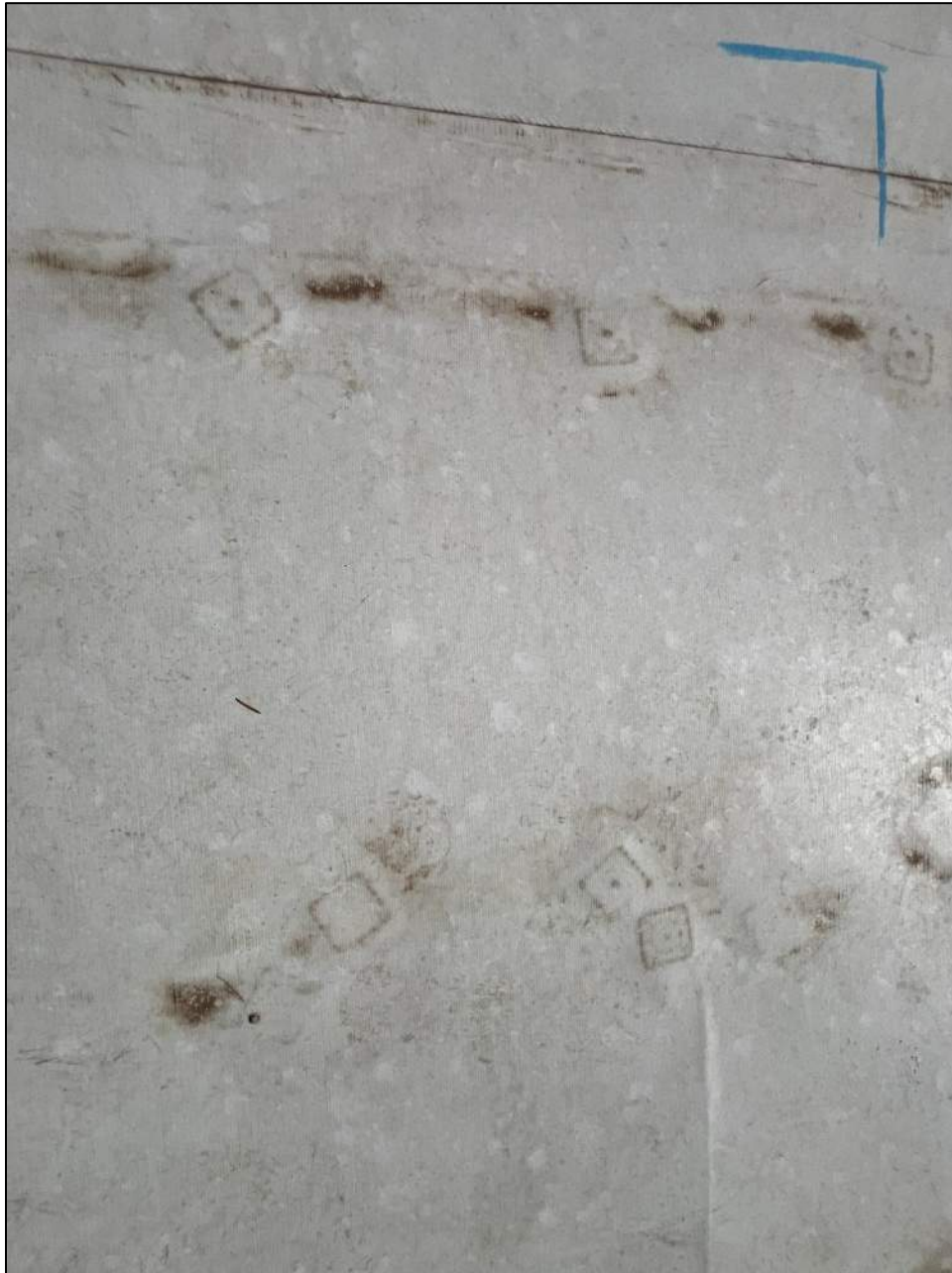
Photo 76: No impact fractures were observed at the tented membranes in the vicinity of stress plates.
