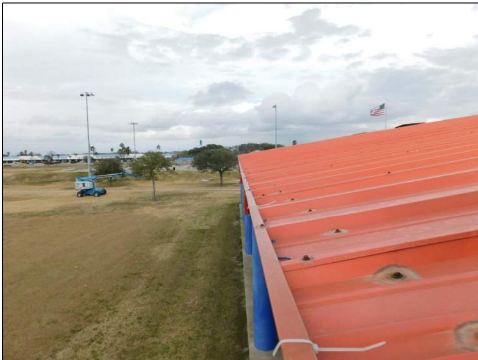
Photo 49: Gutters along west roof eave remained intact.
