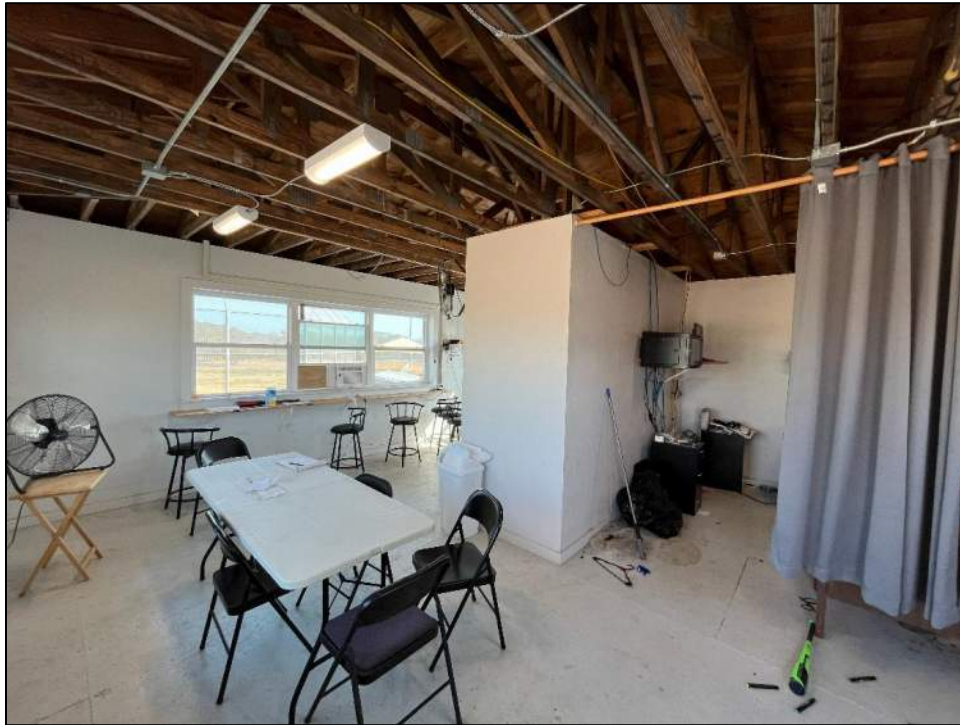
Photo 36: Interior space of the upper floor was inspected. No evidence of recent water infiltration was observed.
