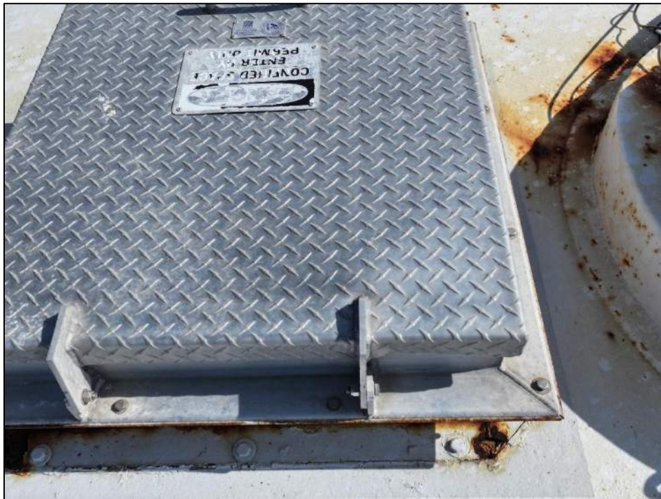
Photo 23: Embossed square access doors on roof remained intact.
