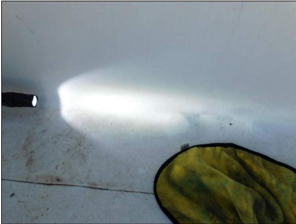
Photo 61: Parapet bases facing the direction of the hail impact were closely inspected after surface cleaning for hail impact.
