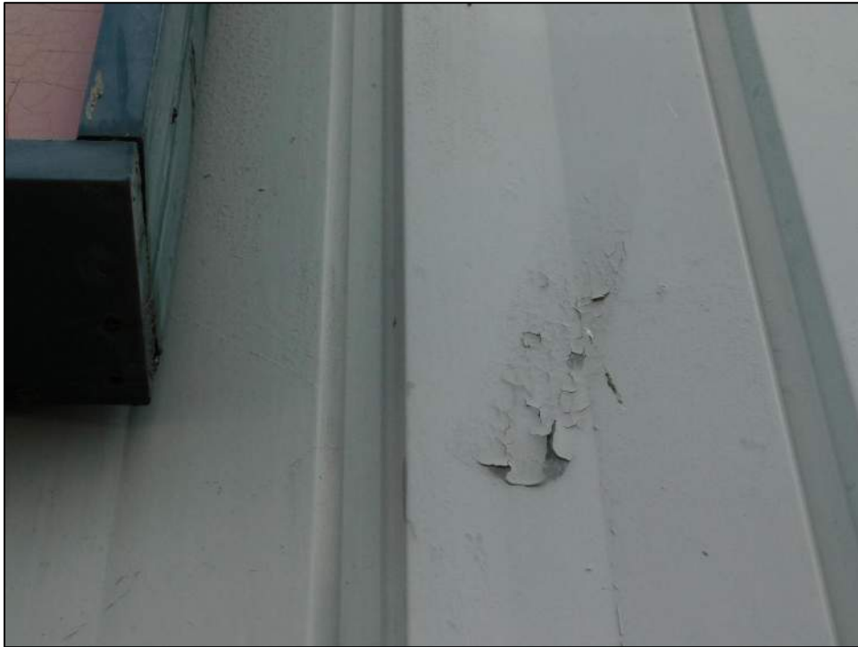
Photo 21: Paint peel near the west wall sign irrelevant to hail impact.
