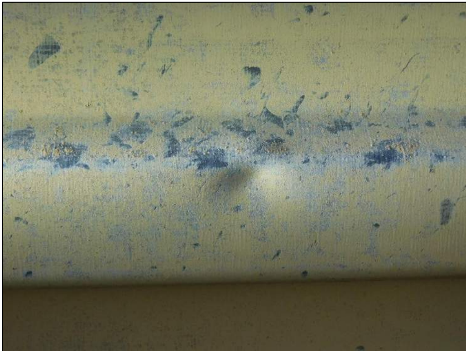
Photo 95: Denting on the front wall of the storage building unaccompanied by hail spatter.
