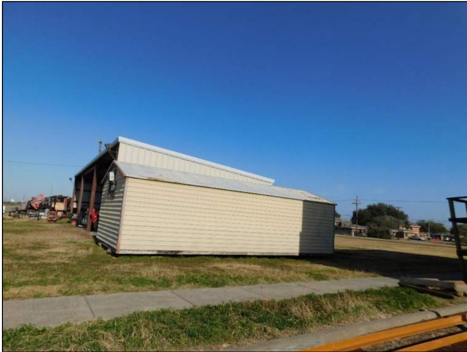
Photo 81: East elevation of the storage building.
