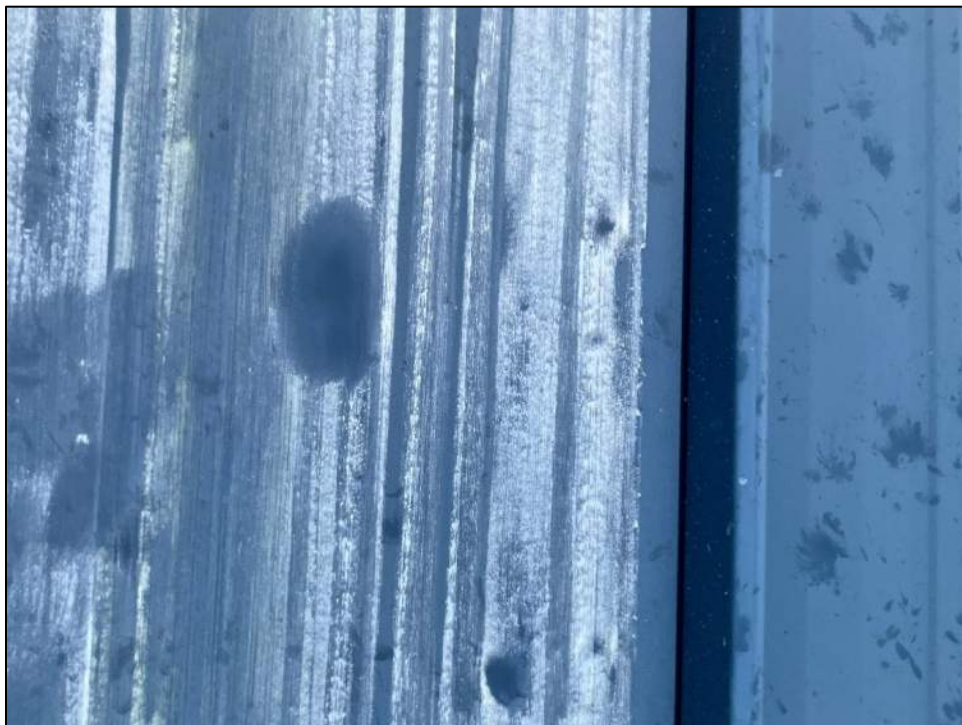
Photo 14: No coating disruptions were observed at the hail dents or spatters.
