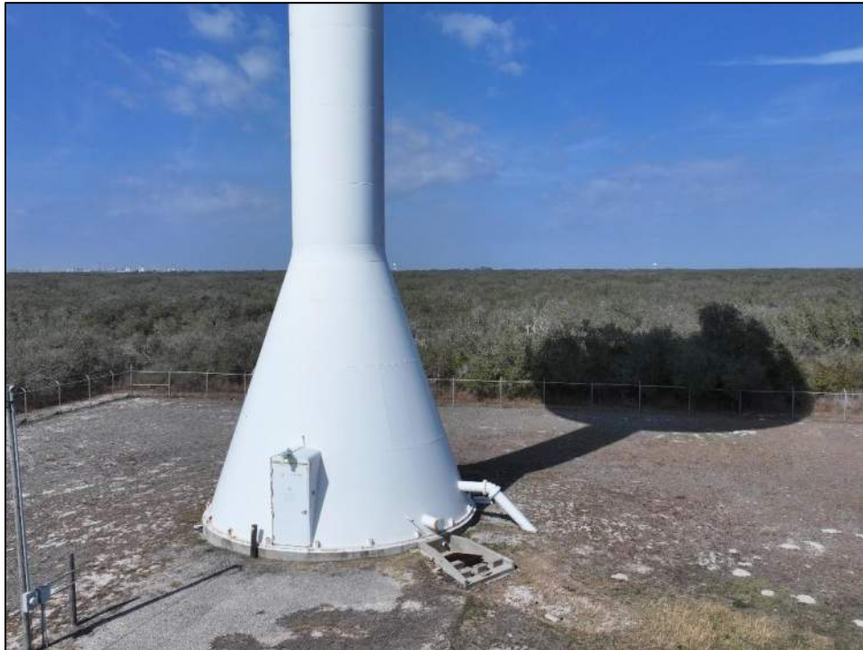
Photo 3: Steel base of the water tank.
