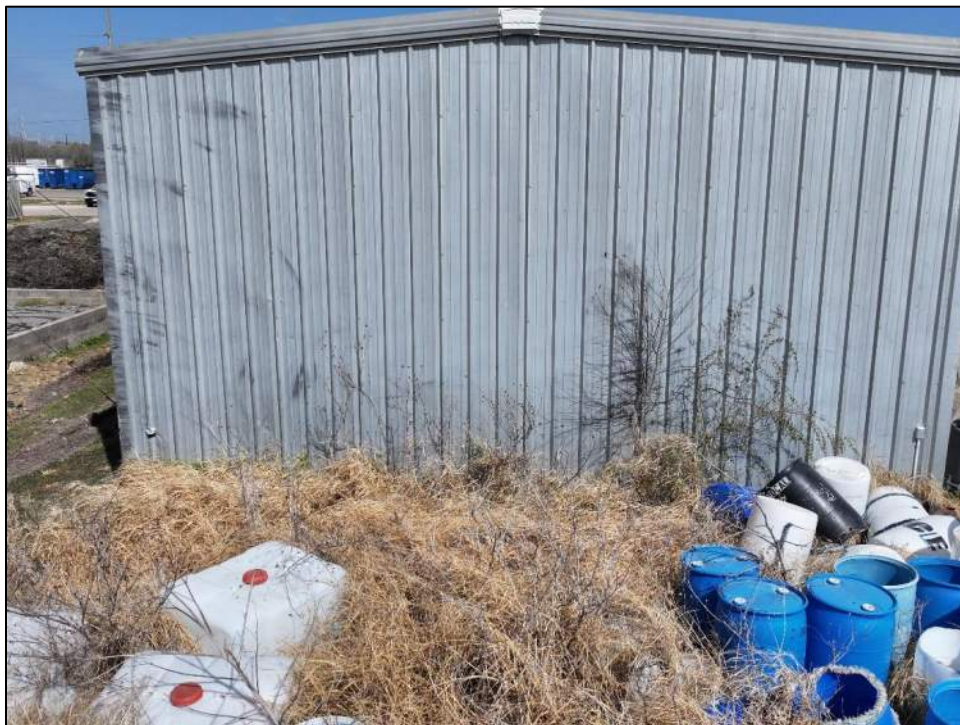
Photo 74: South elevation of the vehicle storage building.
