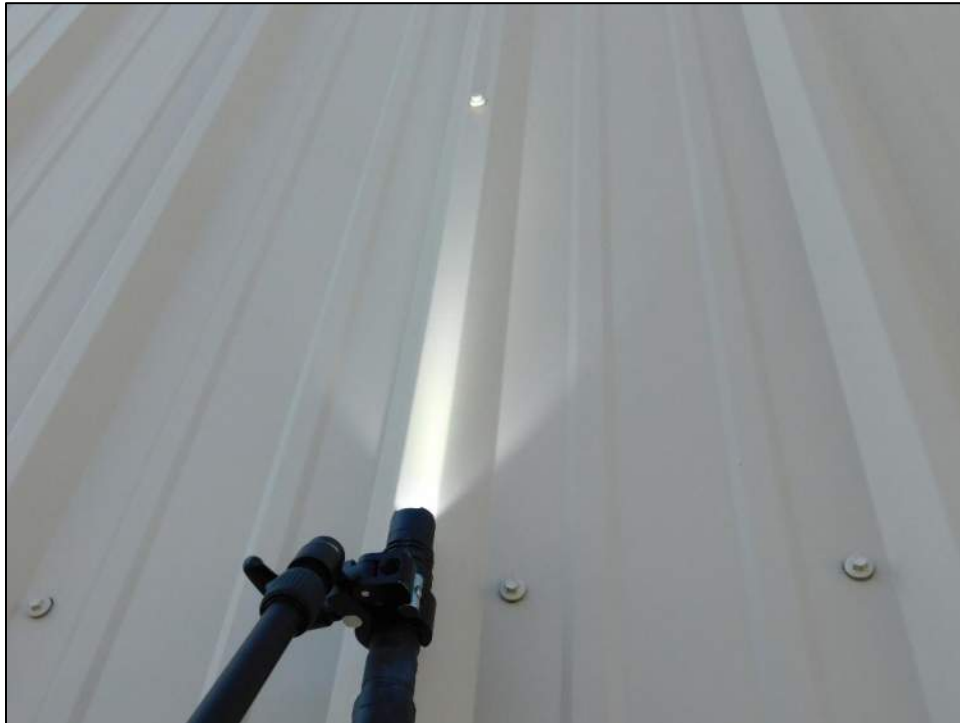
Photo 7: No hail denting visible on north or west walls.
