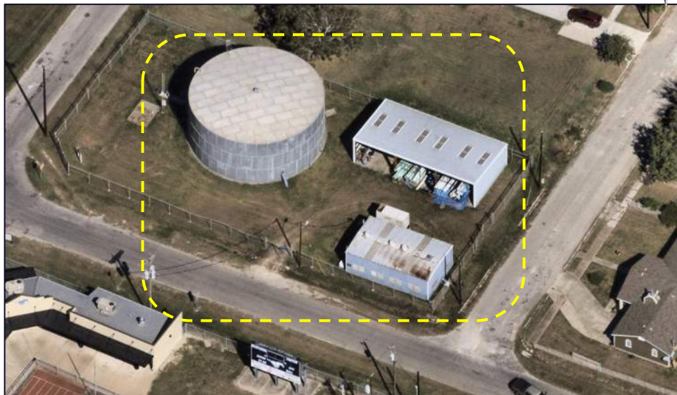
Figure 12 – Structure Group 017 (001-003), the Water Department. Date of Imagery: November 9, 2024. Source: Nearmap®.
