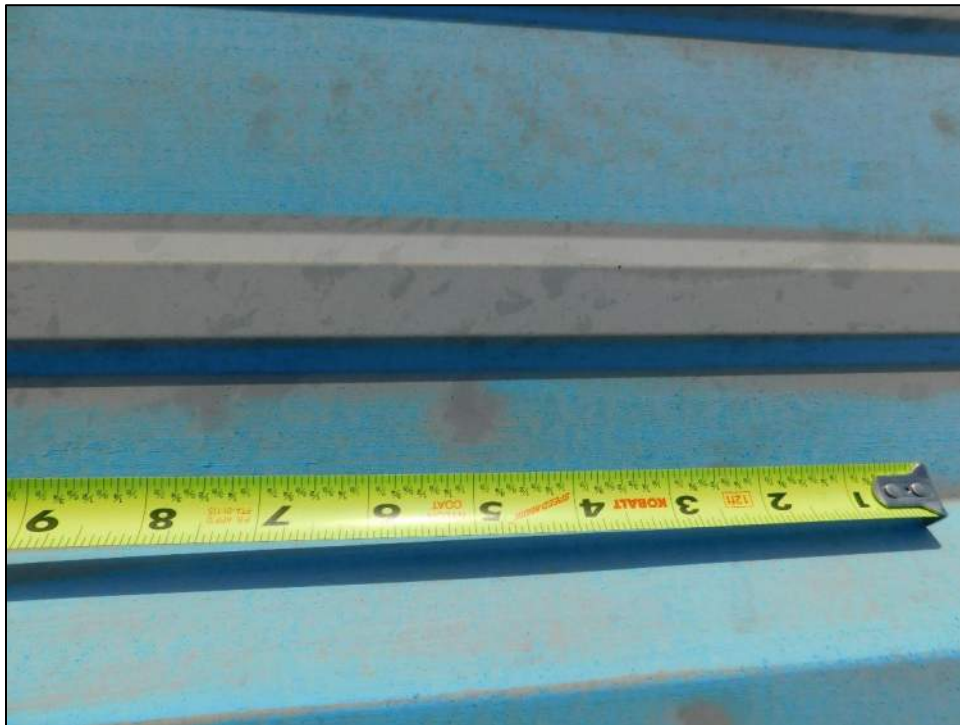
Photo 21: No coating disruptions were observed at the hail dents or spatters.
