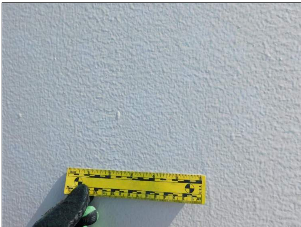
Photo 12: Surface coating of tank stem remained intact.
