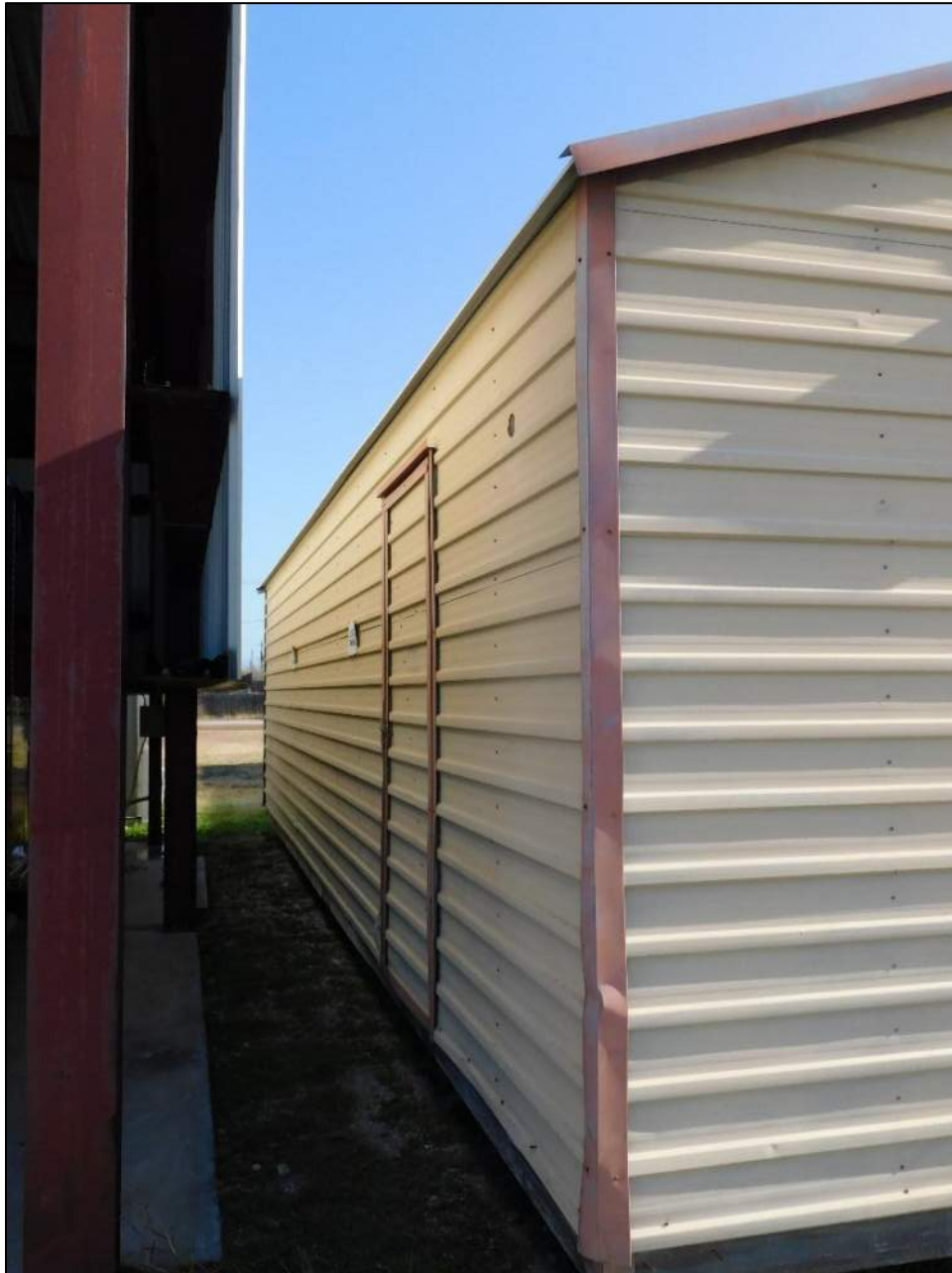
Photo 83: West elevation of the storage building.
