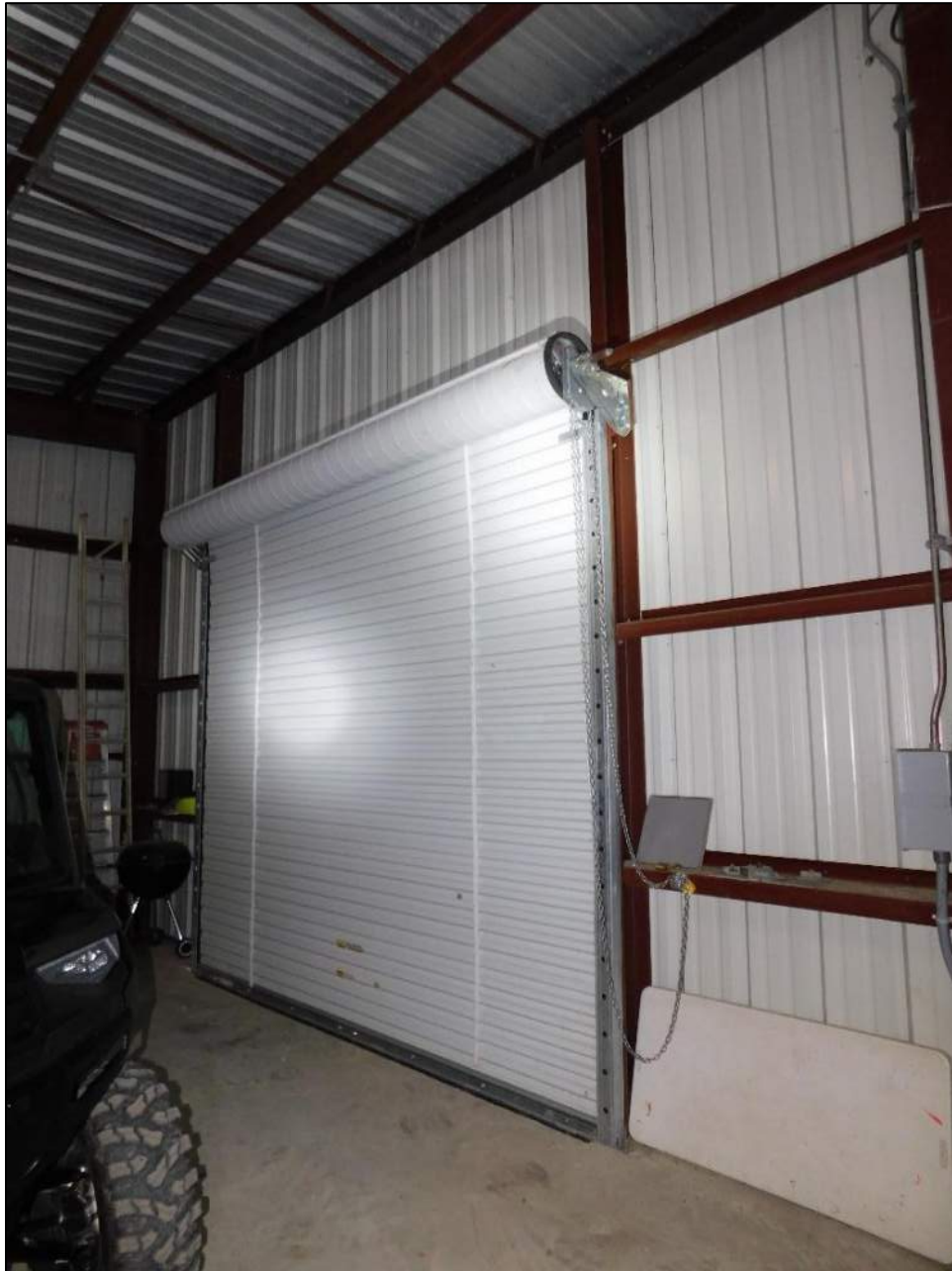
Photo 14: Inside view of the south roll-up door on the west wall.
