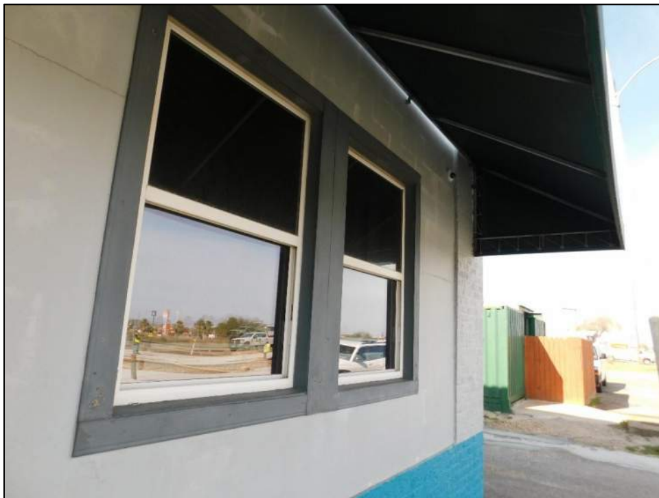
Photo 12: Windows along east elevation remained intact.
