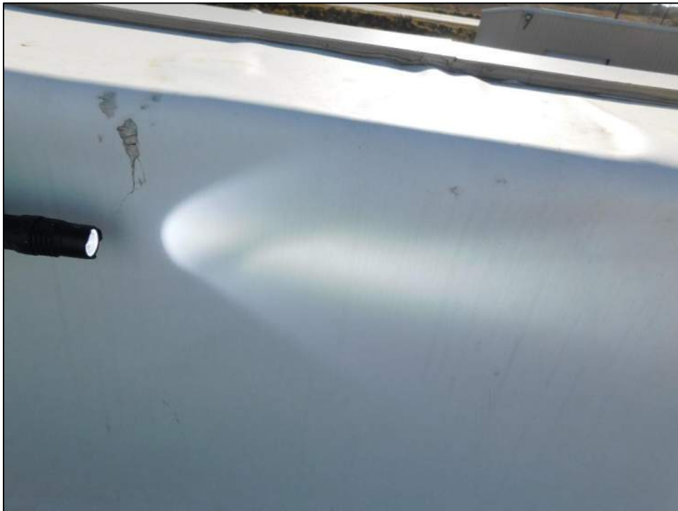
Photo 62: No hail impact dimpling puncture or surface disruptions were observed at the membrane flashing at the bases of the parapets.
