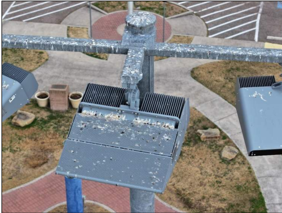
Photo 23: Nearby pole lights were not fractured or dented.
