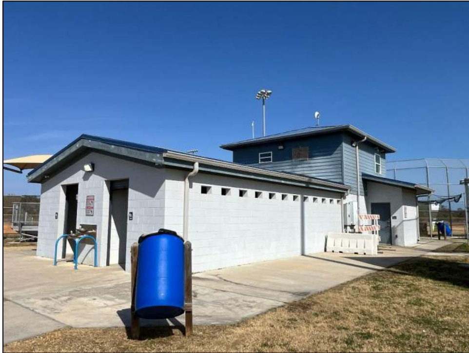
Photo 1: Front (west) and south elevations.
