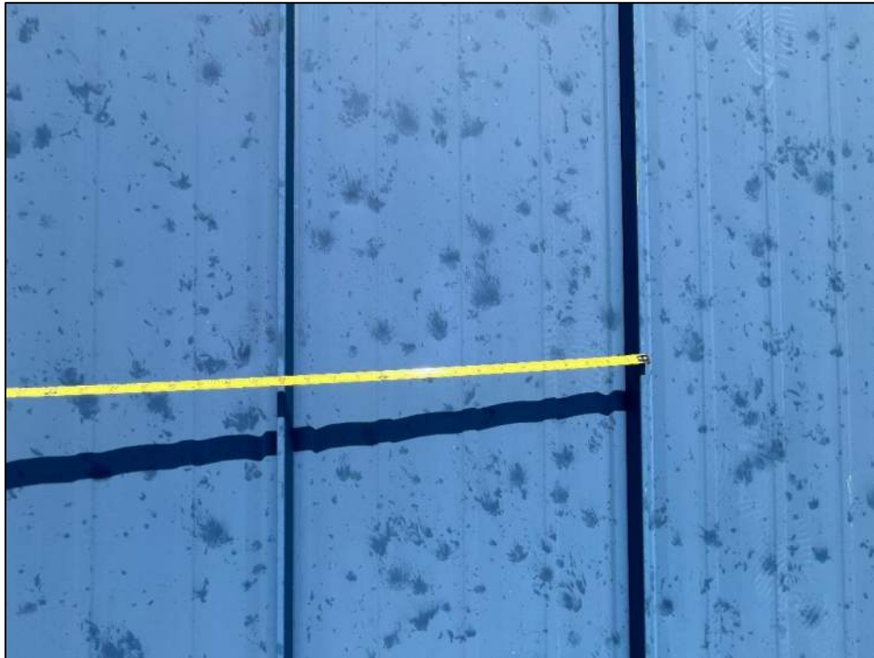
Photo 11: Largest hail spatter reflected up to 1.5-inch hail at this site.
