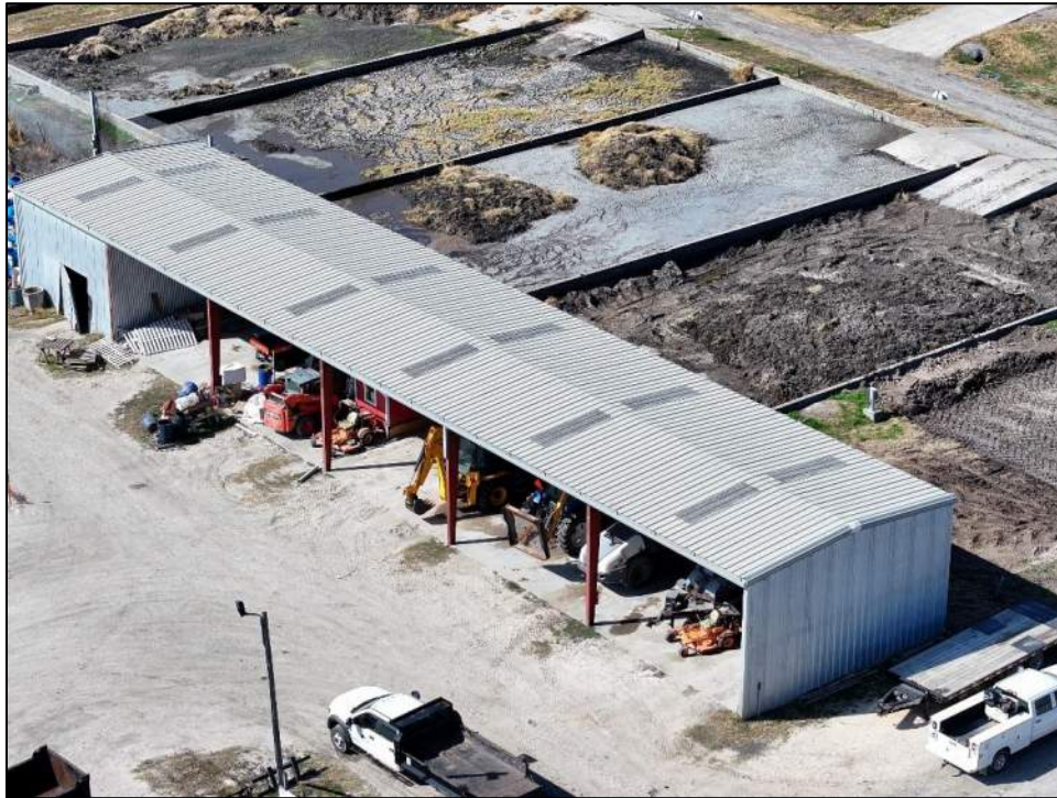
Photo 73: Overview of the equipment pole barn building.
