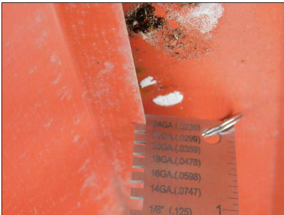
Photo 37: 24 gauge metal thickness.
