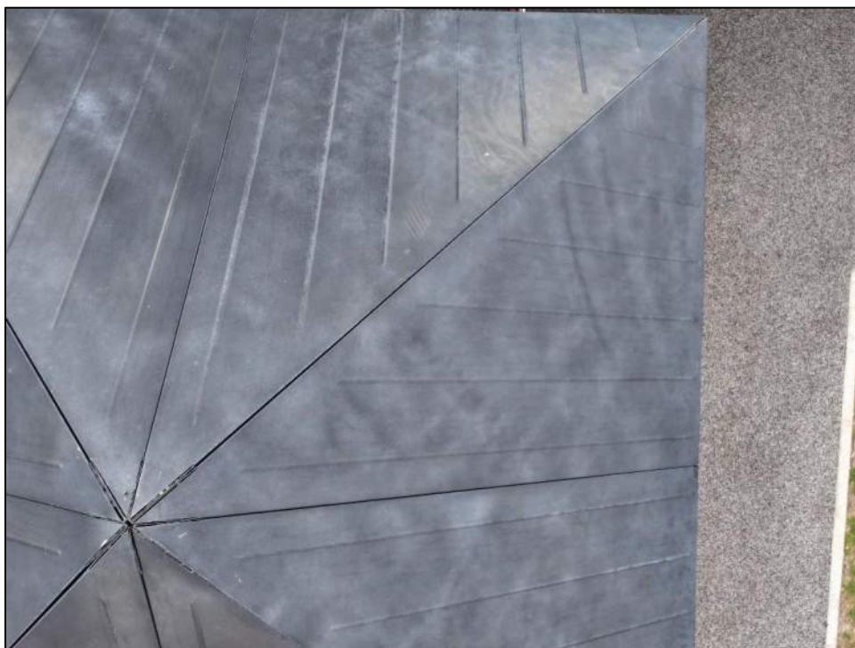
Photo 104: The roof is made of steel plates. No hail impact indentations were observed.
