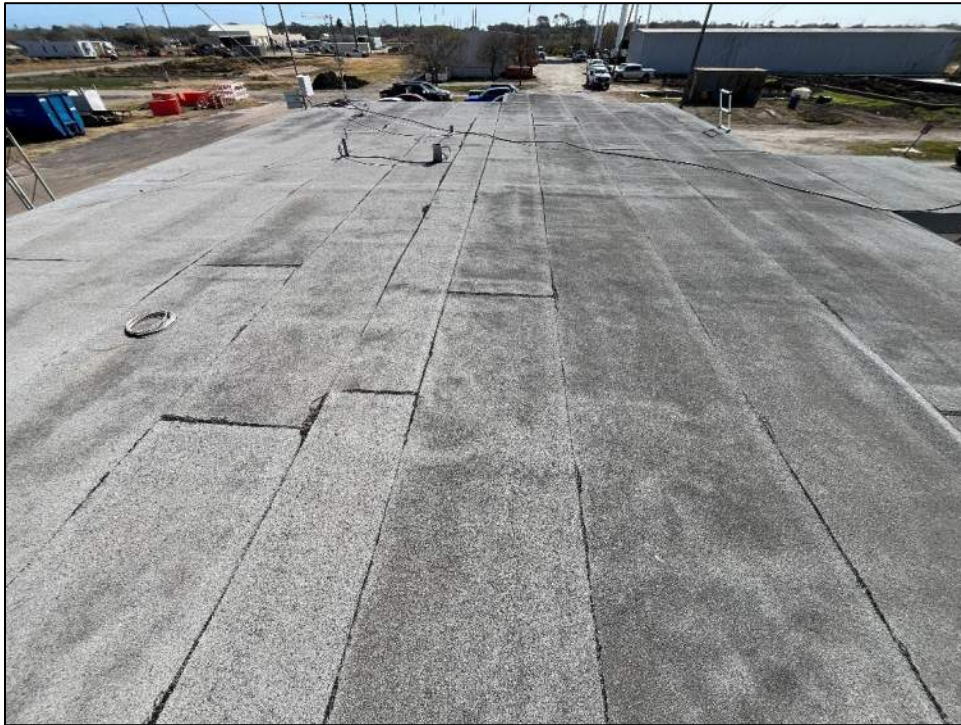
Photo 42: Mod-bit roofing overview.
