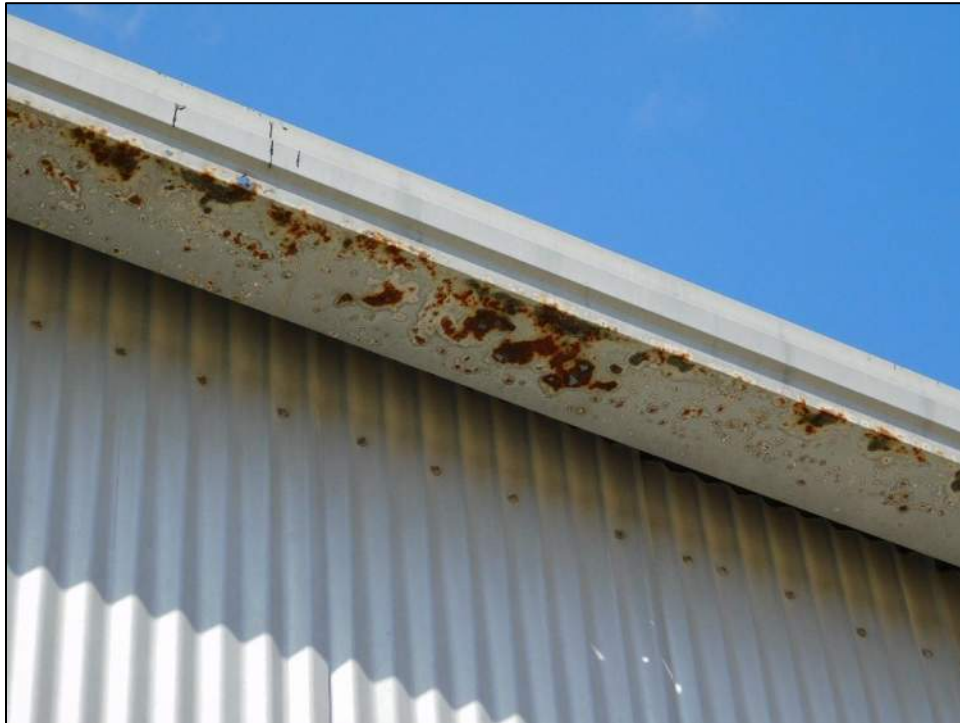
Photo 89: Corroded gutter.
