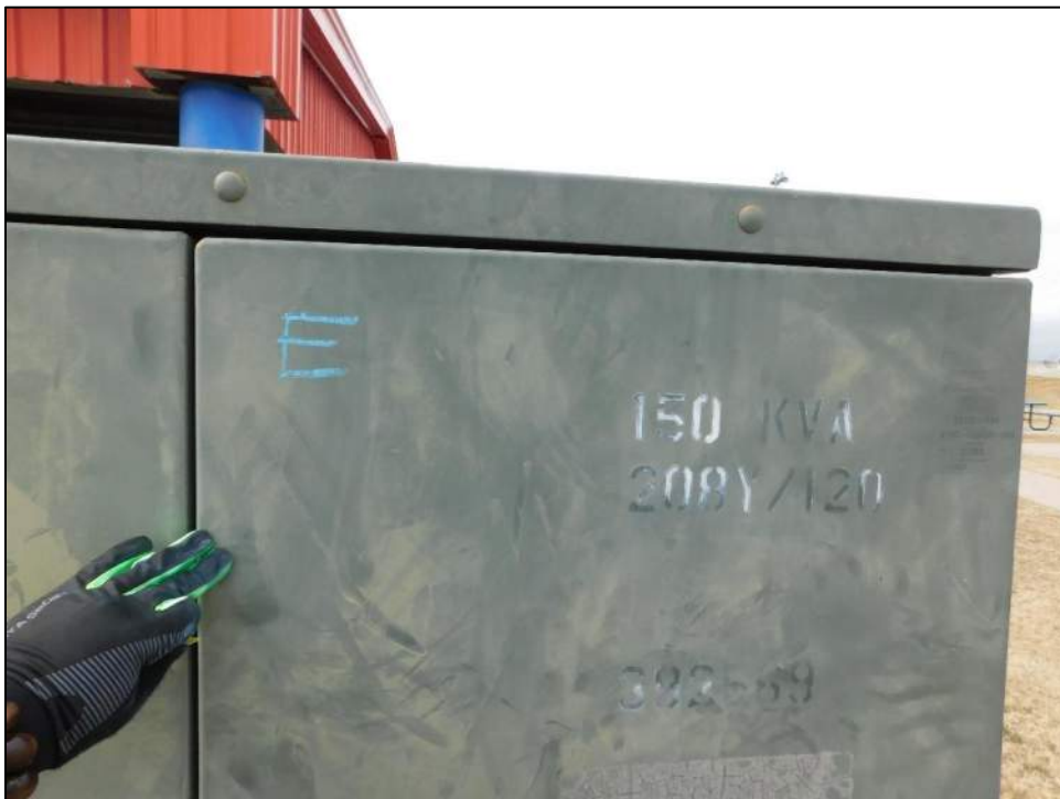
Photo 30: No hail spatters on east-facing surfaces.
