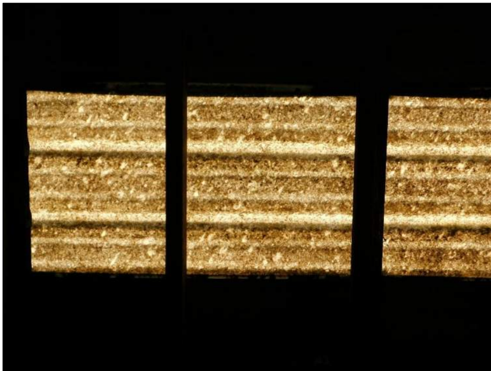
Photo 99: No fractures observed on the underside of the skylight panels observed in the enclosed storage room at the south end of the vehicle storage building.
