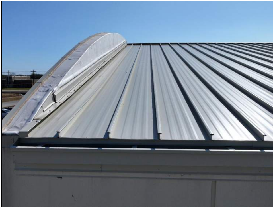
Photo 31: Double-lock standing seam of the metal roofing above the fire department was newly installed.
