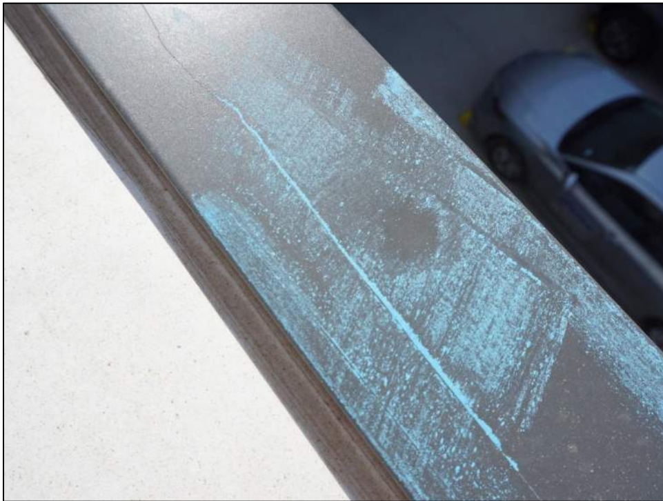
Photo 22: No coating disruptions were observed at the dent in the parapet coping.
