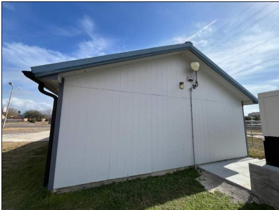
Photo 2: West elevation. No hail peck marks were observed on the wall panels.
