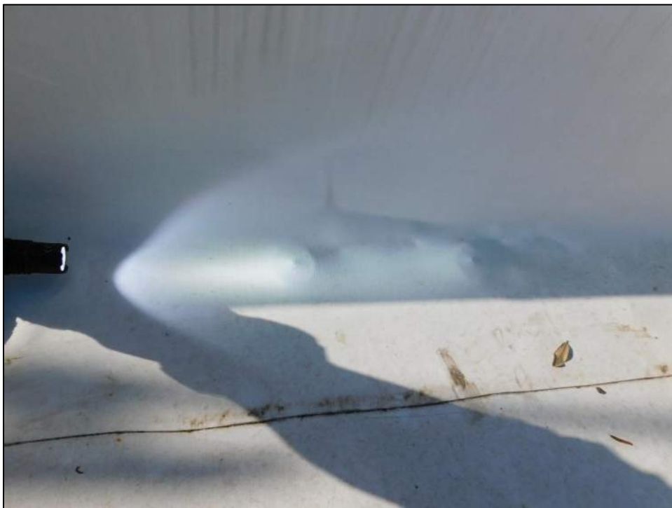
Photo 50: Parapet bases facing the direction of the hail impact were closely inspected for hail impact.
