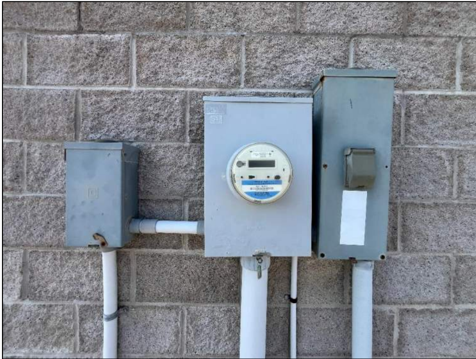
Photo 7: East wall was unaffected by hail.
