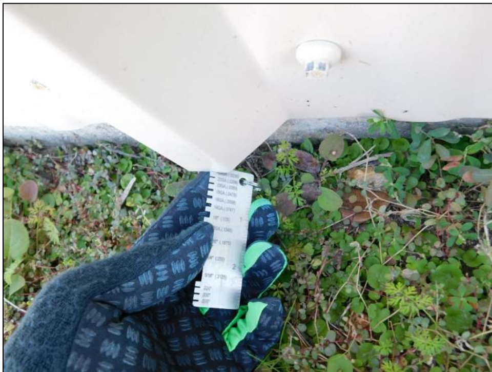
Photo 8: 24 gauge wall panels.
