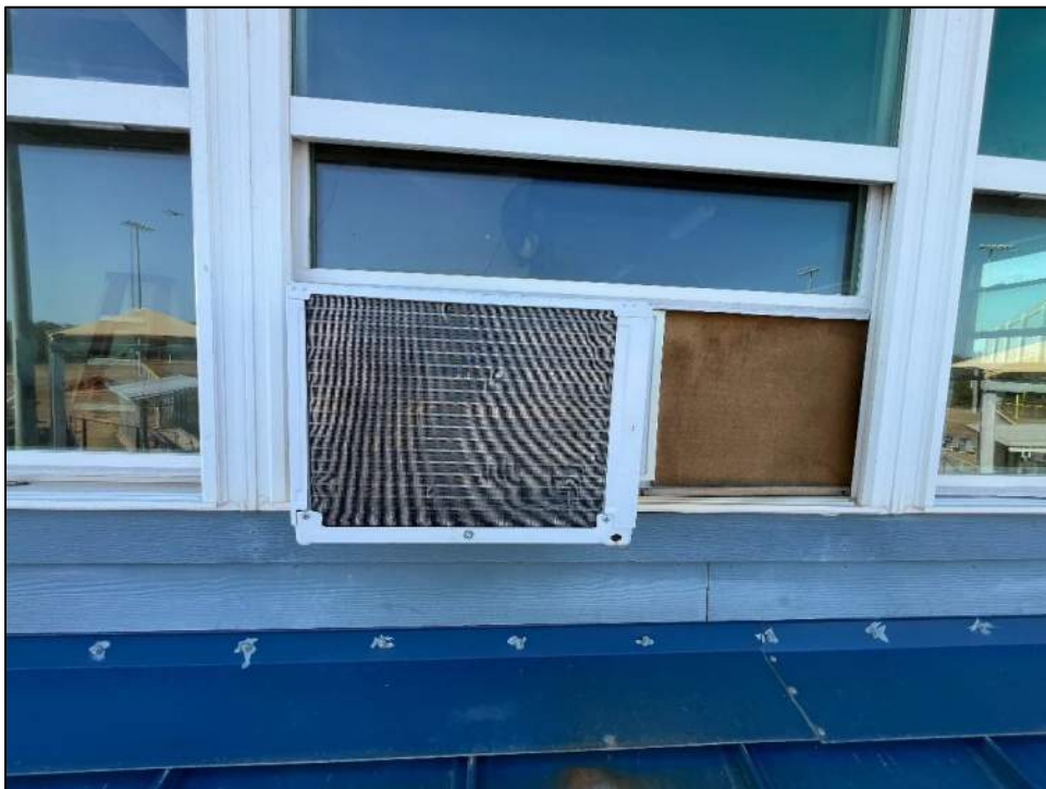
Photo 24: Window AC unit in east-facing window were absent of hail denting.
