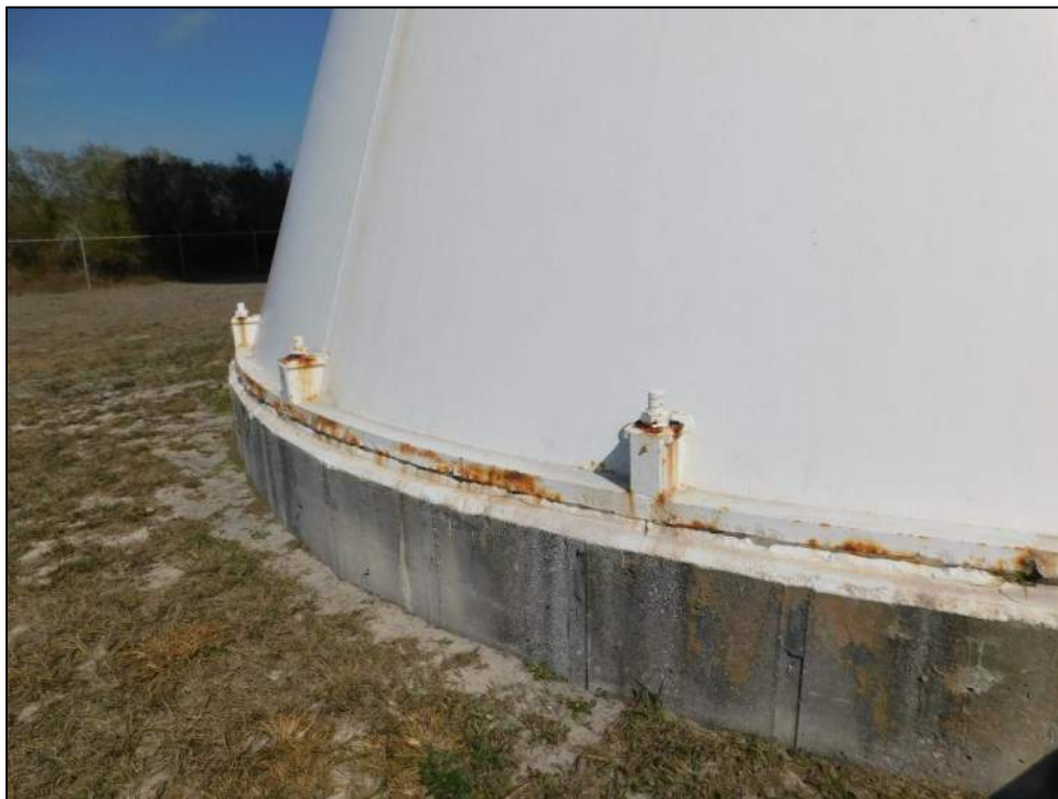
Photo 8: Base attachment to concrete foundation remained intact.
