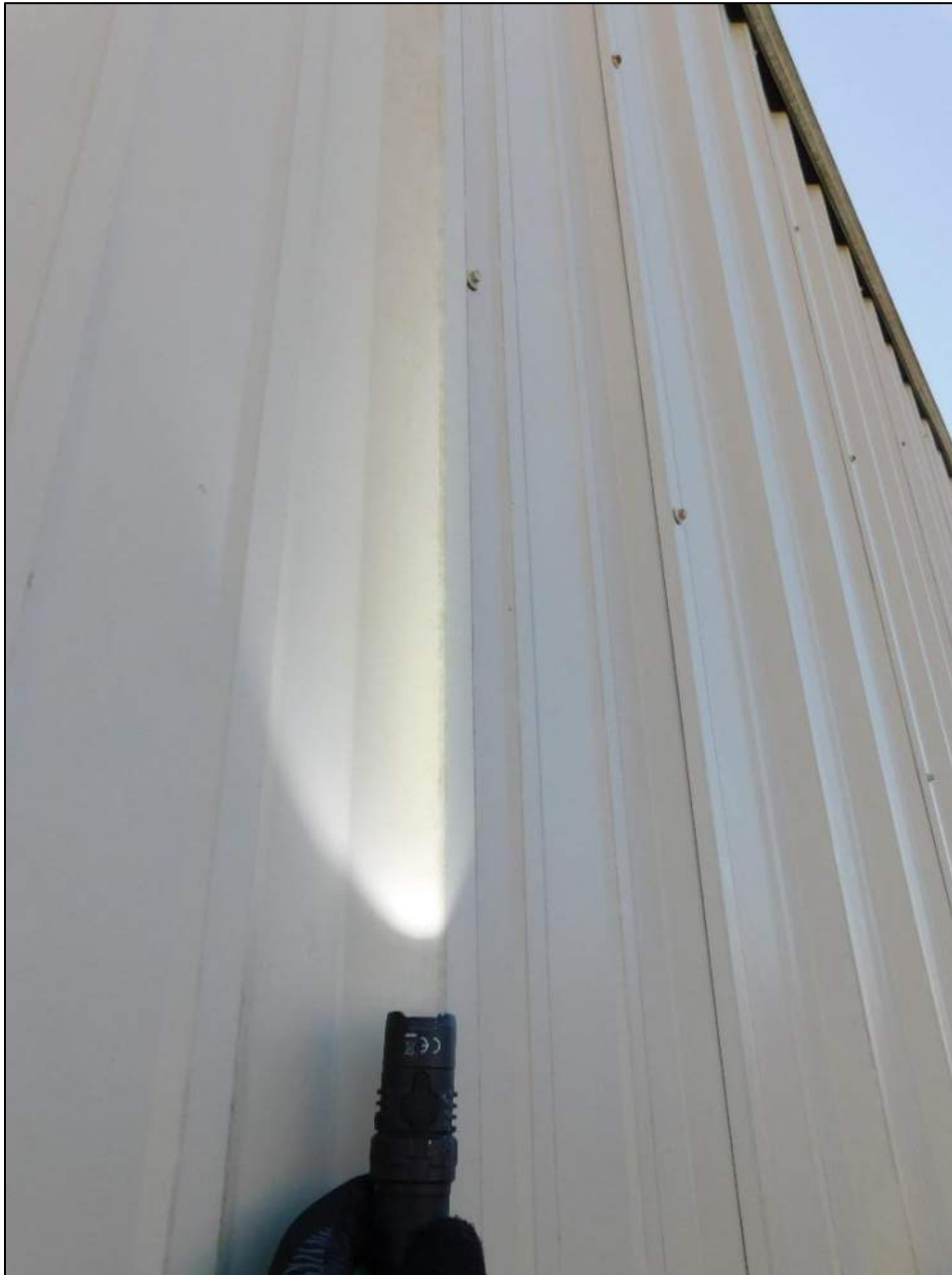
Photo 98: No hail indentations observed on the metal R-panel walls in the north elevation.
