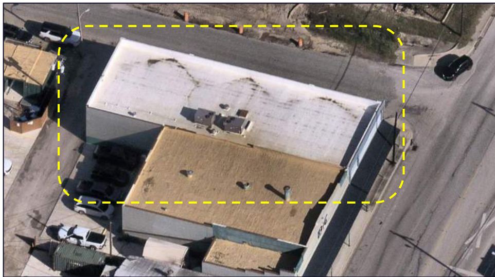
Figure 10 – Structure 014-001, the Humber Youth Rec Center. Date of Imagery: December 2, 2025. Source: Nearmap®.
