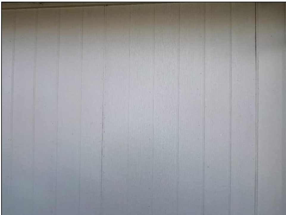
Photo 8: Siding panels were absent of hail peck marks.
