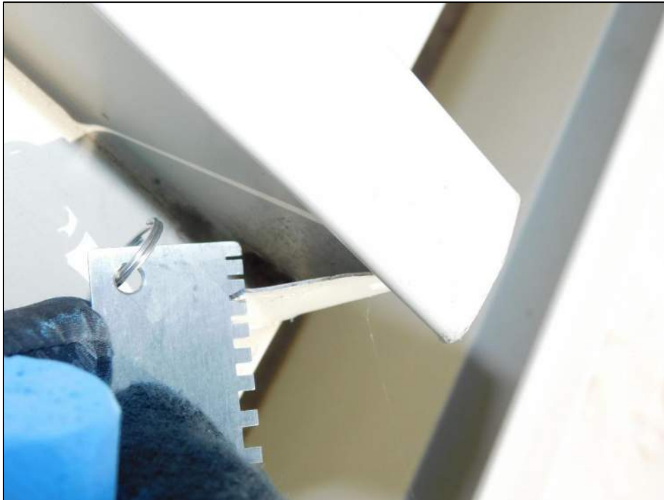
Photo 55: 20 to 22-gauge thickness recorded for the standing seam metal roofing of the fire department building.
