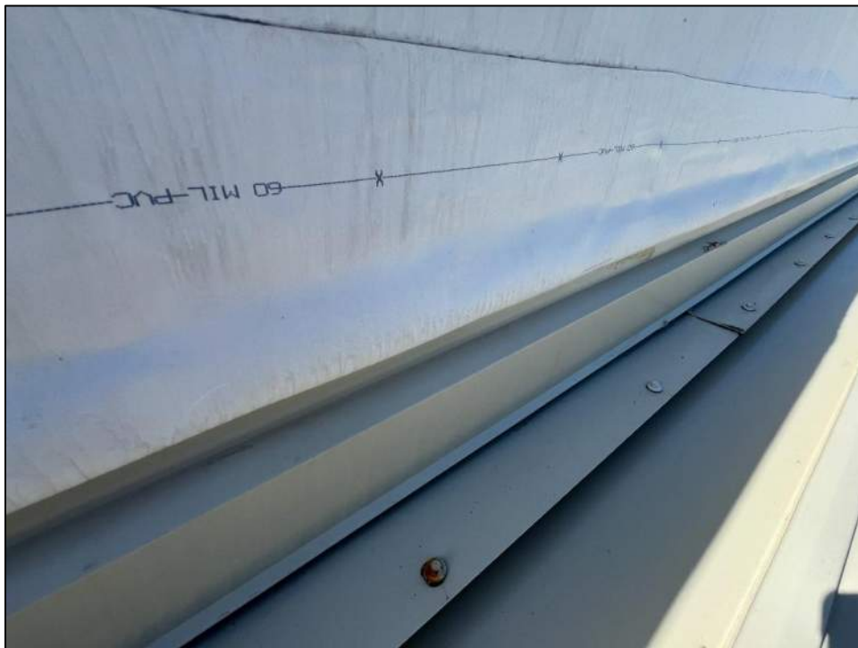
Photo 71: Intact PVC membrane at the base of the south kneewall above the fire department roof.
