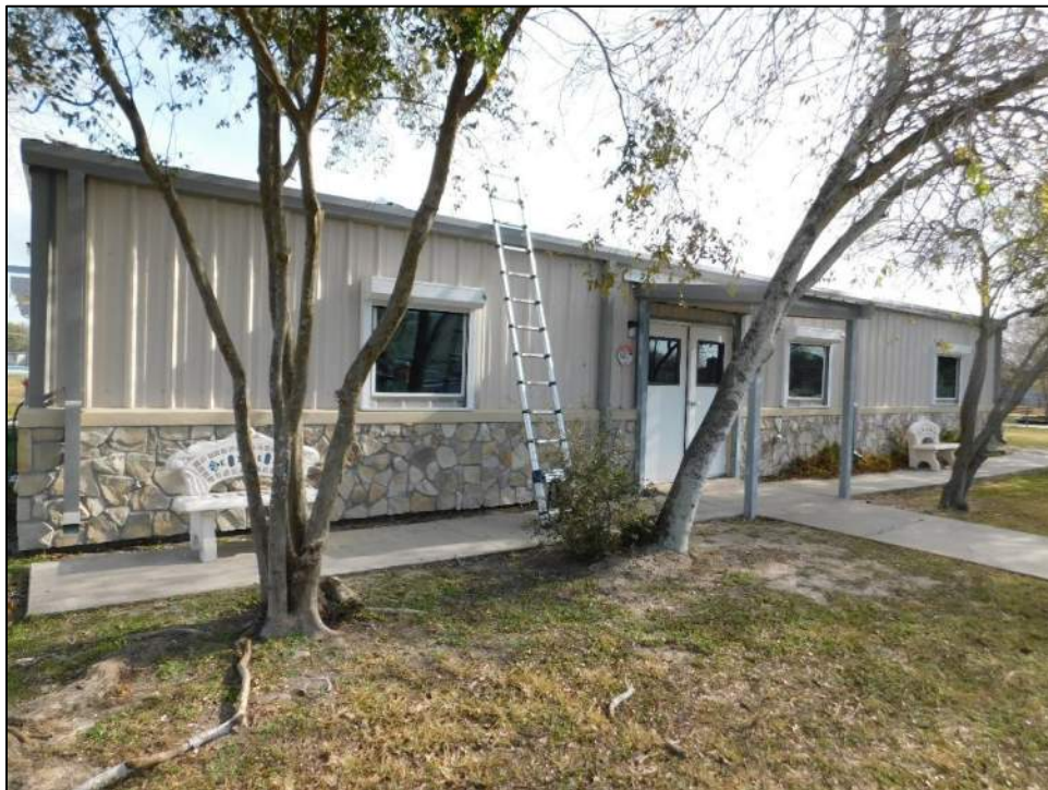
Photo 2: South elevation. No window glazing damage observed.
