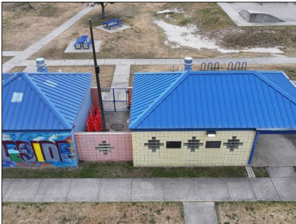
Photo 55: Top-down overview of the concession stand and the park restroom.
