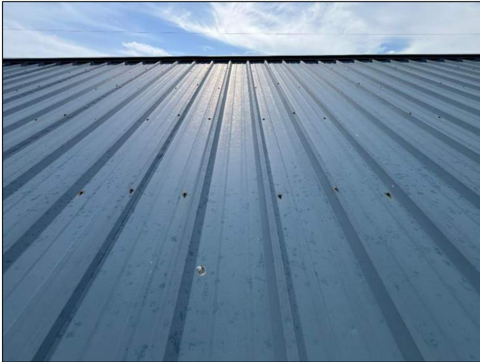
Photo 15: North slope overview.
