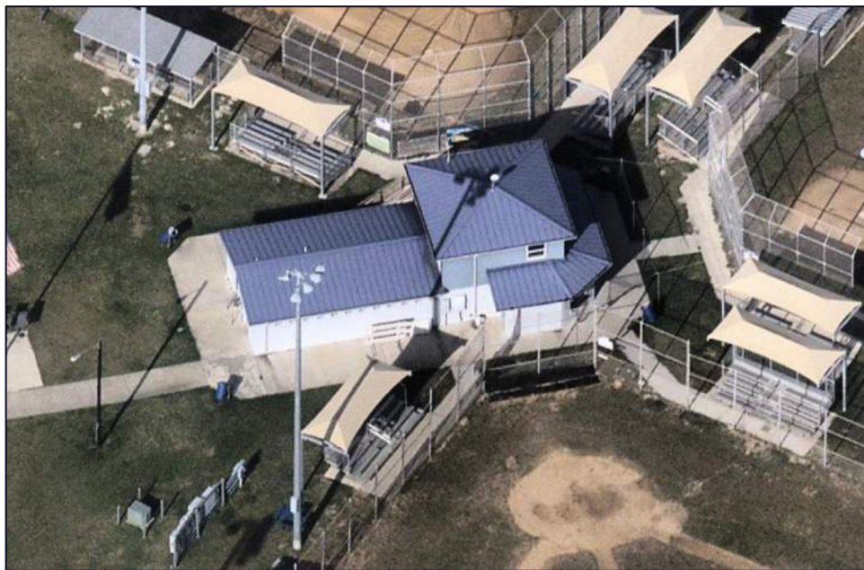
Figure 4 – Structure 004-003, the Concession Stand/Restroom – Parks & Rec / Bennie Diegel Park. Date of Imagery: December 2, 2025. Source: Nearmap®.
