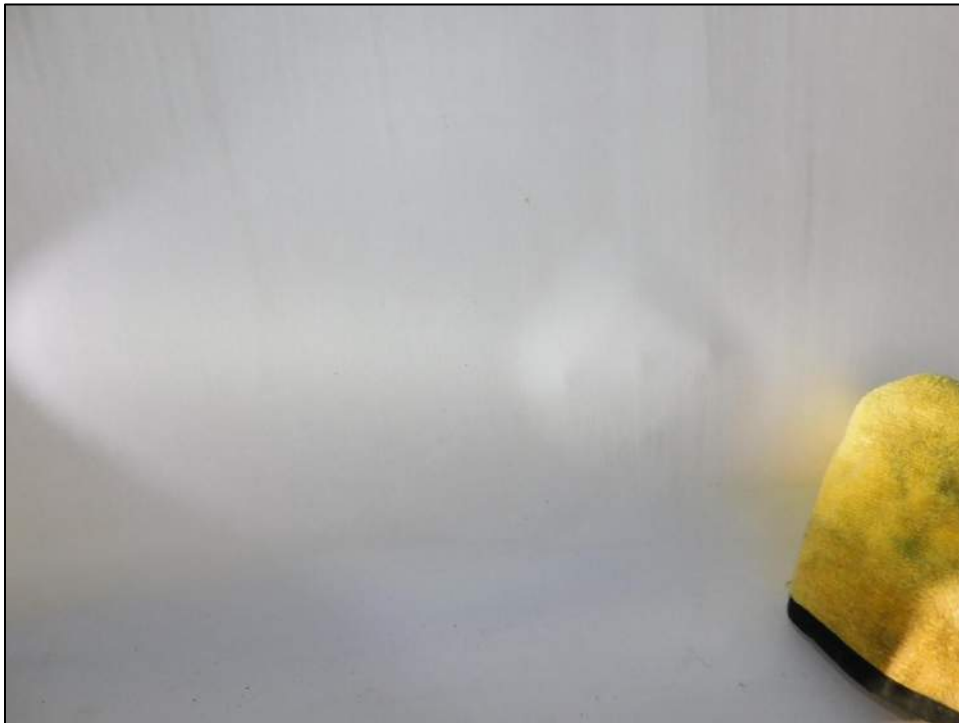
Photo 52: No hail impact dimpling puncture or surface disruptions were observed at the membrane flashing at the bases of the parapets.
