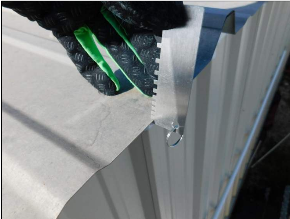
Photo 101: 24-gauge metal panel.
