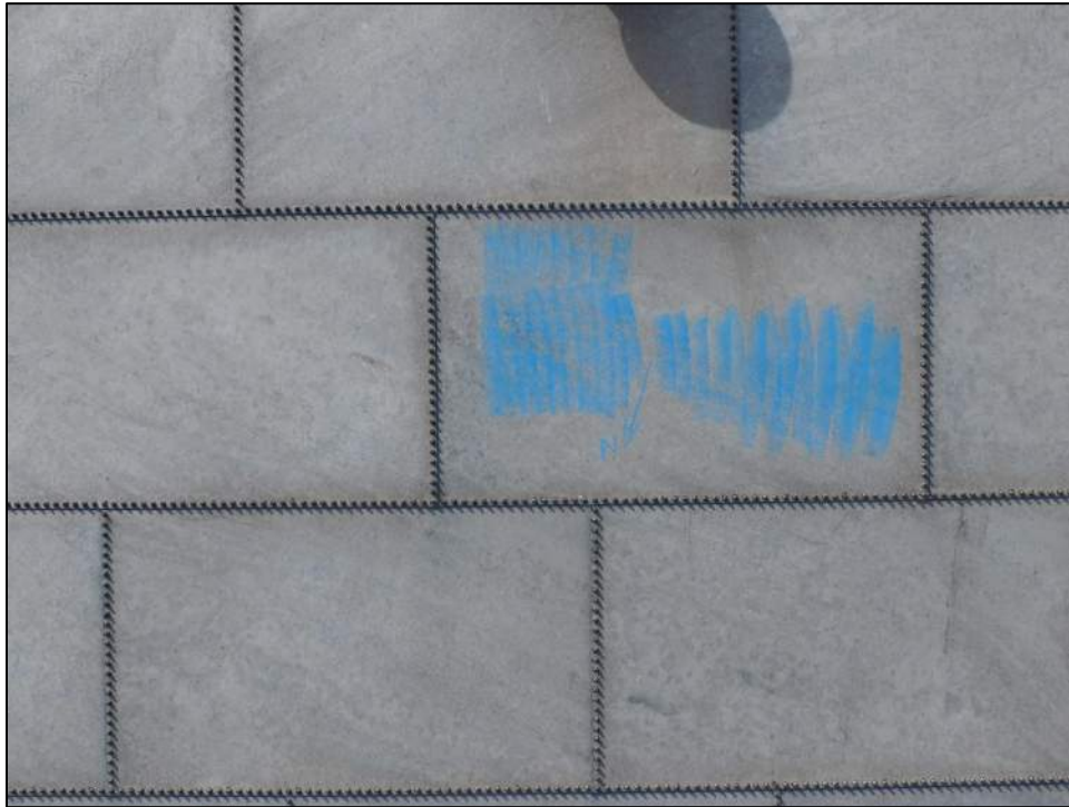
Photo 63: Tank walls exhibited no hail denting.
