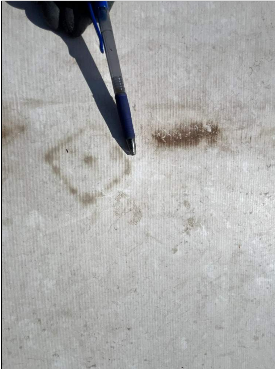
Photo 77: No impact fractures were observed at the tented membranes in the vicinity of stress plates.
