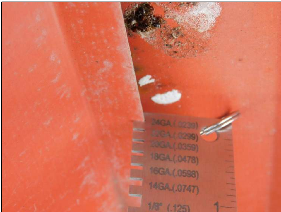
Photo 37: 24 Gas metal thickness.
