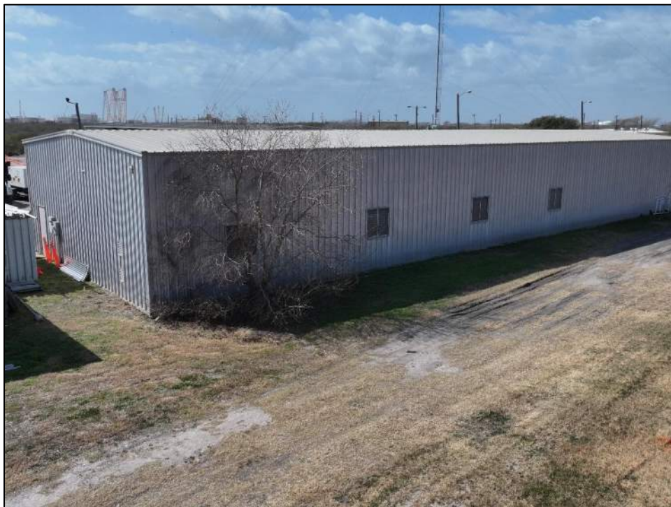
Photo 51: Rear elevation of the vehicle repair building. Screen covered louver windows were present along this elevation.
