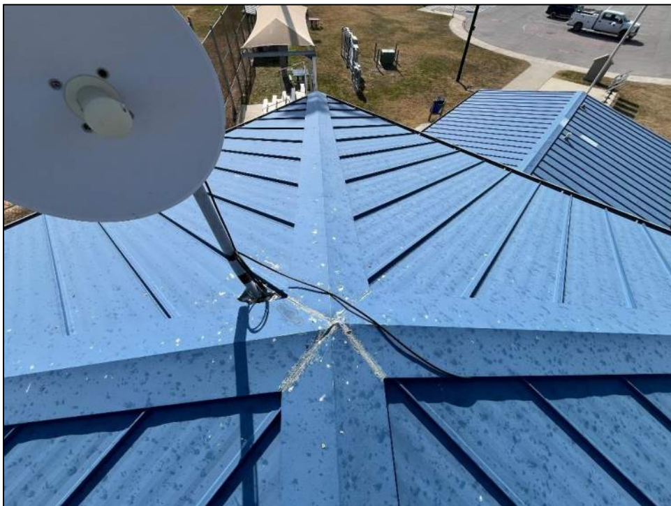
Photo 32: Rooftop appurtenances were not displaced or detached.
