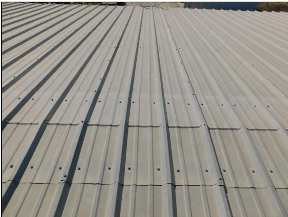
Photo 64: Ridge panels were intact.
