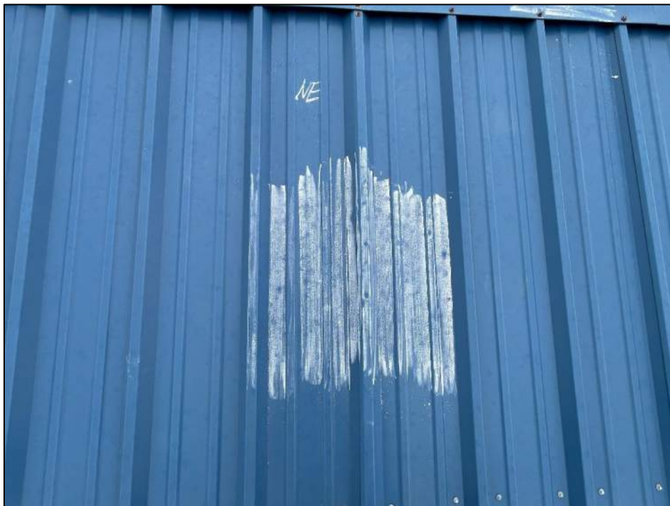
Photo 10: Hail spatters and denting observed on north slope indicative of 1-inch hail.
