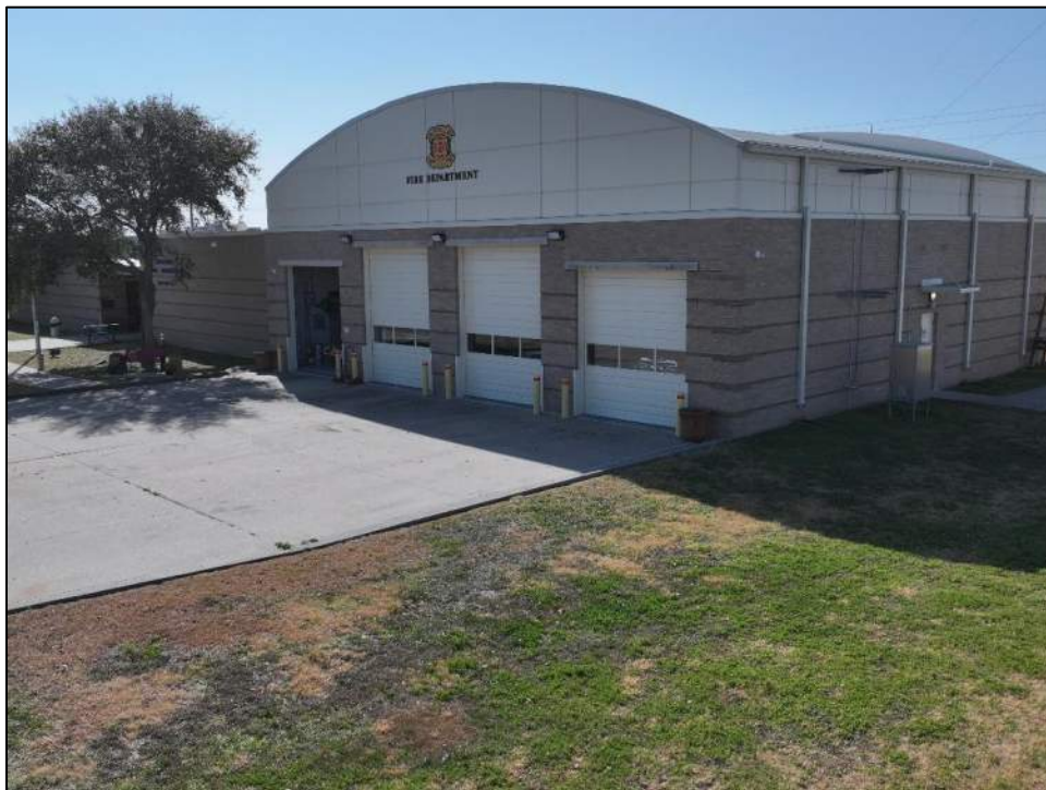
Photo 30: North (front) and west elevation of the fire department building.
