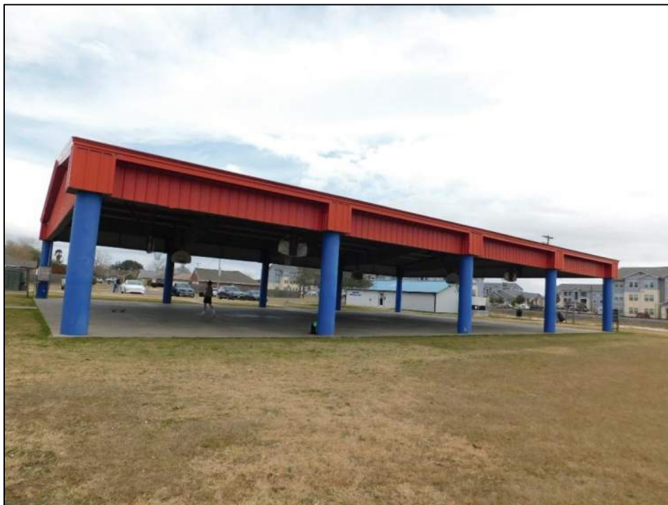
Photo 20: West elevation of the sports court.
