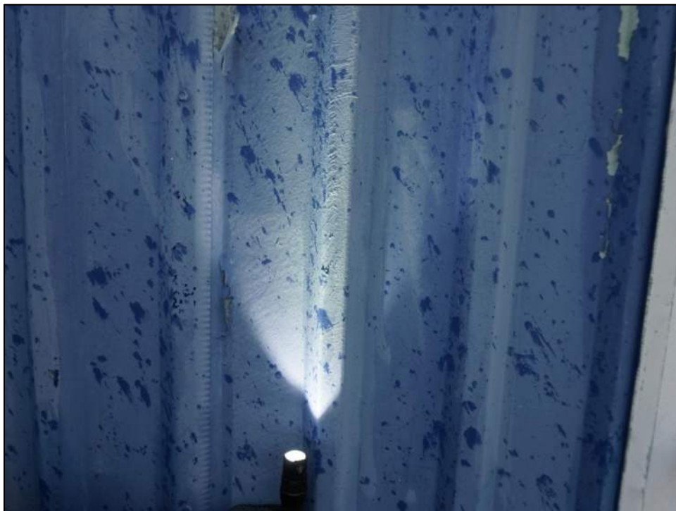
Photo 34: No hail denting was observed on the west wall. Existing coating exhibited aged-related peel.
