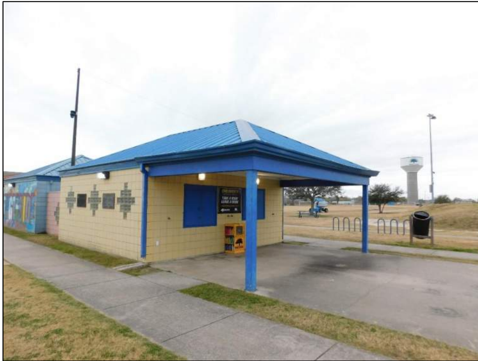
Photo 56: North and east elevation.
