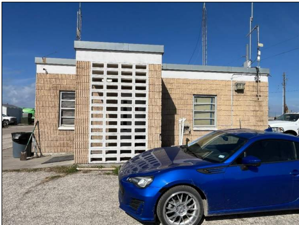
Photo 33: East elevation of the storage building (formerly the public works admin building). Windows were intact.
