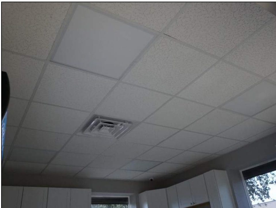
Photo 29: No moisture stains observed on ceiling tiles.
