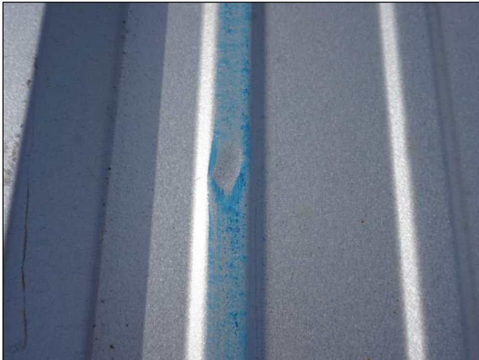
Photo 27: No coating disruptions were observed on the galvalume surface of the metal deck at the dents.
