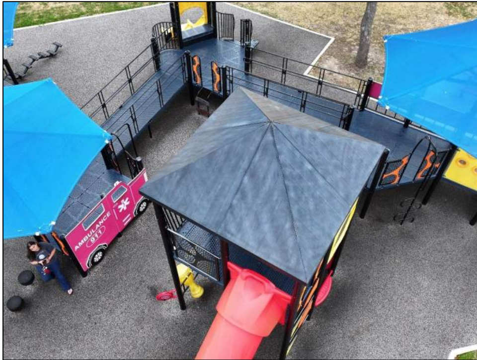
Photo 103: Top view of the playset metal roof.
