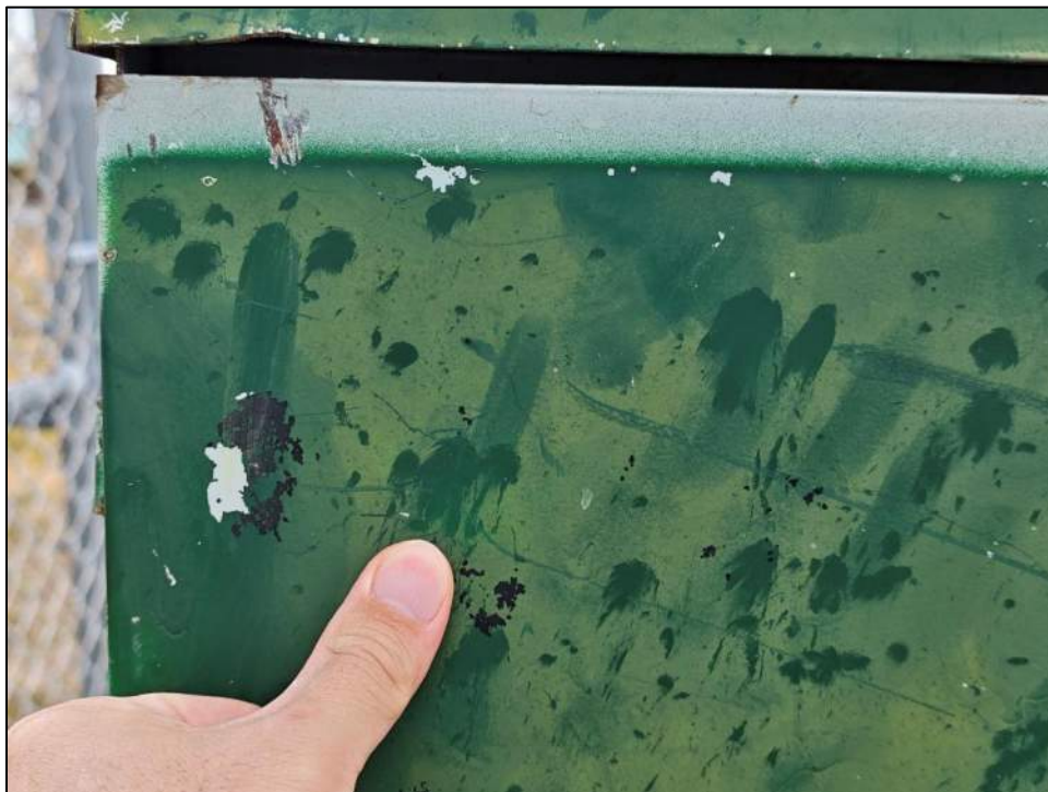
Photo 21: Hail spatters on nearby break panel box reflected approximately 1-inch hail.
