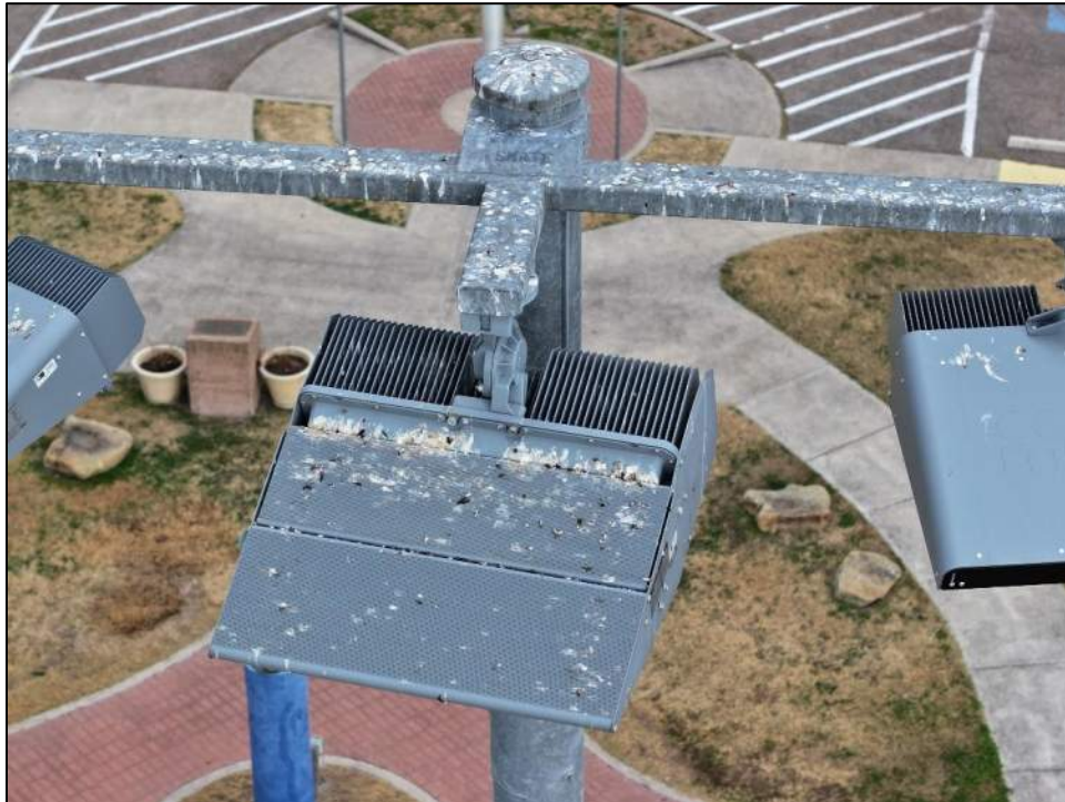
Photo 23: Nearby pole lights were not factured or dented.
