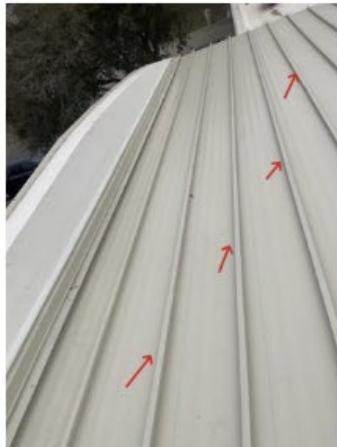
Photo Documentation 16 Crew has not started rolling metal seems
