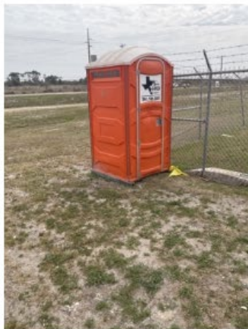
Photo Documentation 3 Porta-John remains on site
