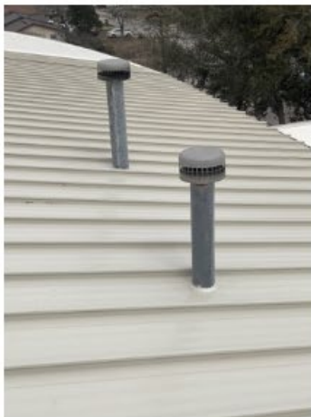
Photo Documentation 8 Penetrations caulked around vents
