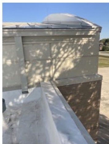
Photo Documentation 57 ID#/Building Fire Station - 100%
