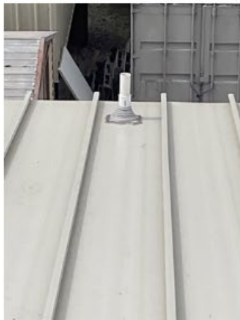
Photo Documentation 11 New neoprene boots installed over vents
