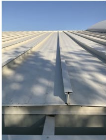
Photo Documentation 58 Metal roof panel seams rolled together
