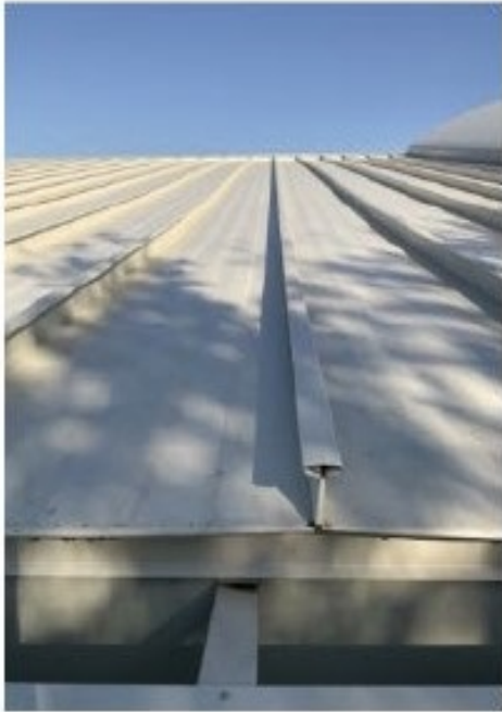
Photo Documentation 58 Metal roof panel seams rolled together
